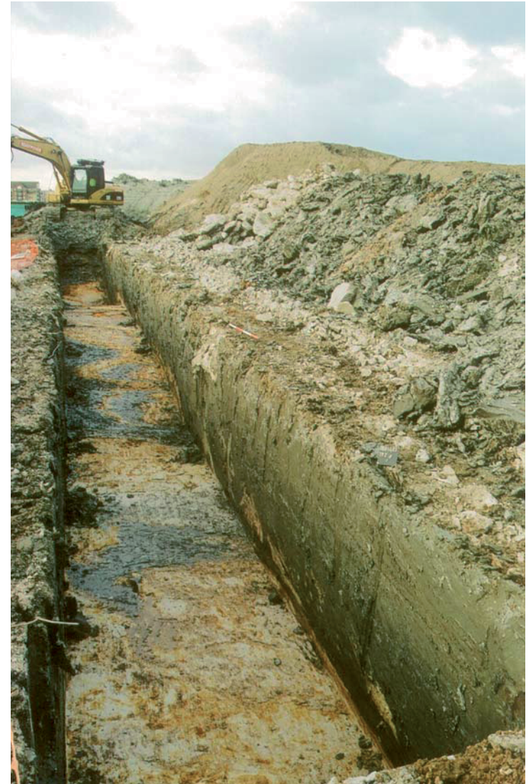
Plate 2. Trench 2b before extension, looking west: scale: 2m.
