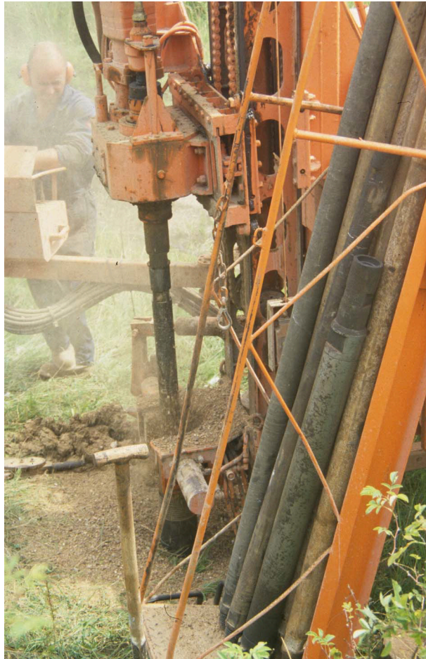
Plate 23: The casing being inserted
