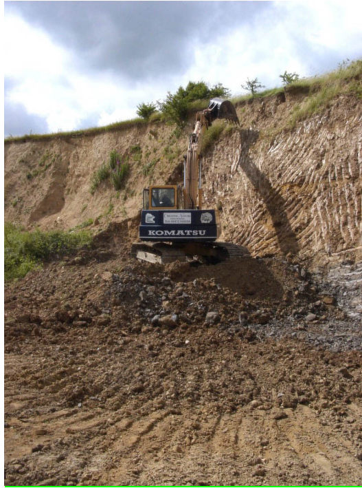
Plate 4: The western face during Facelift work (Photo Helen Gamble)
