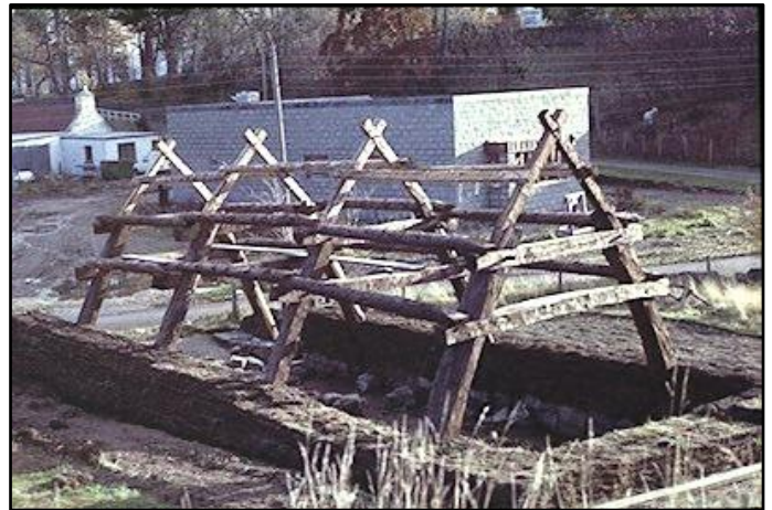
Plate 4: Reconstruction of house in progress showing stone wall 17
