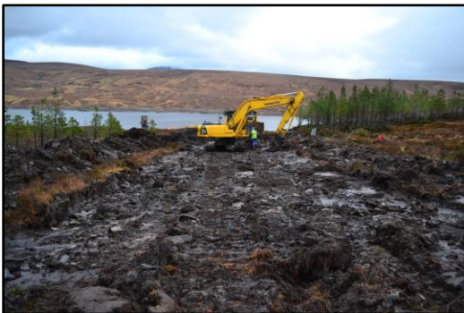
Plates 1 and 2: Stripping the access road.
