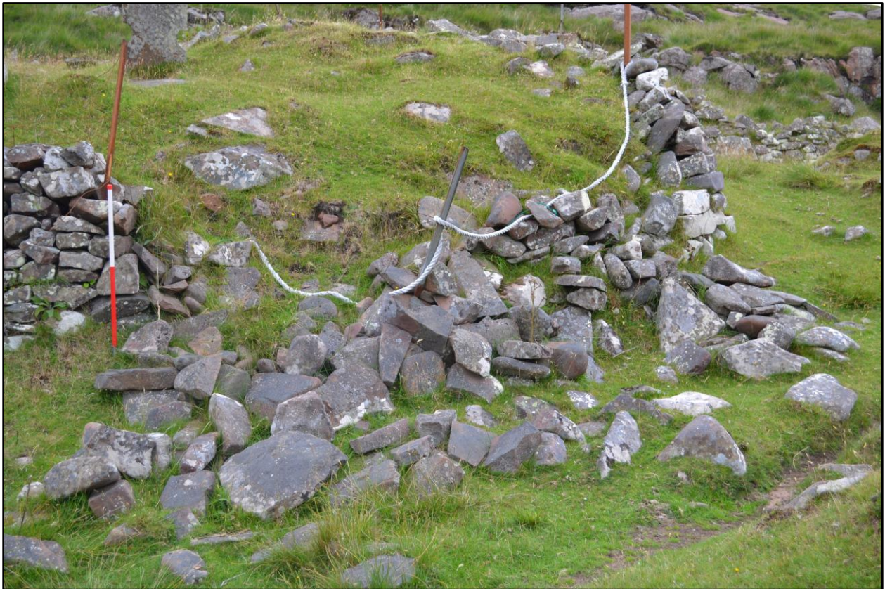
Plate 5: The north-east corner of the wall has the most significant damage. The Cowan headstone can also be seen top left, with the small 'cairn' to its right.
