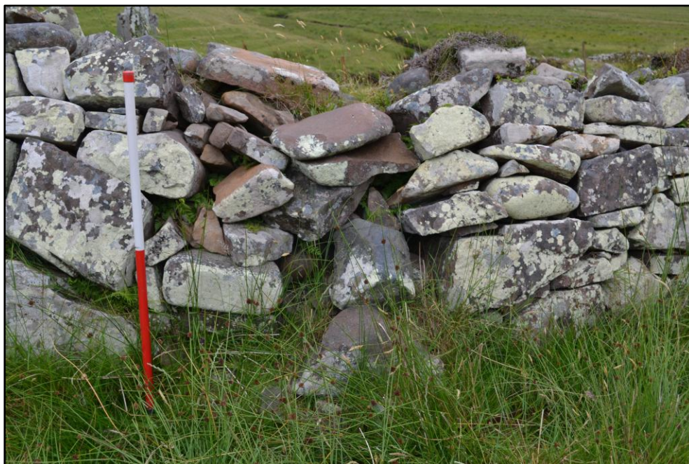
Plate 8: The north-west corner of the wall is starting to collapse.
