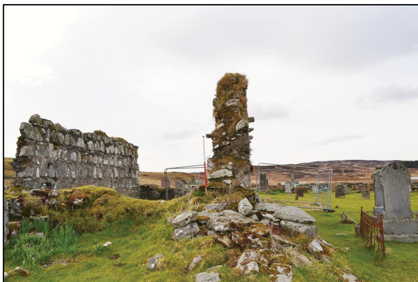
Plate 9: View of the exterior of the east wall (scale 1m)
