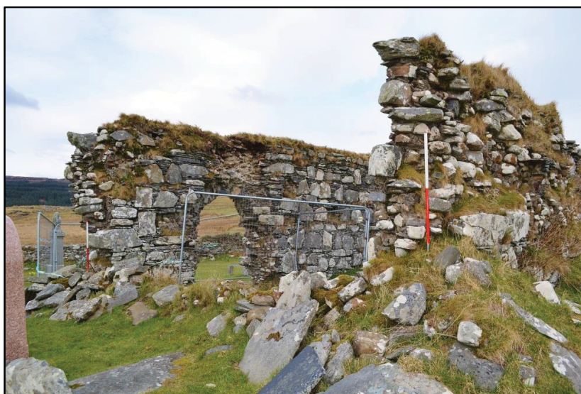
Plate 10: View of the exterior of the west wall (scale 1m)
