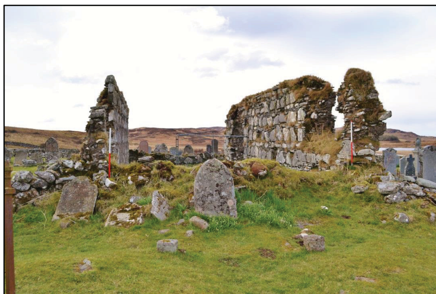
Plate 2: East end of the church showing the extent to which the walls stand
