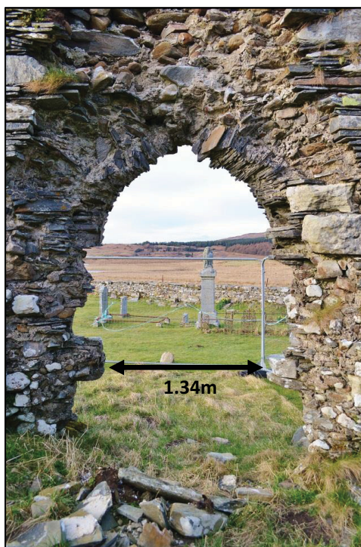
Plate 4: Interior view of the arched doorway showing the stones, which indicate the original width of the doorway
