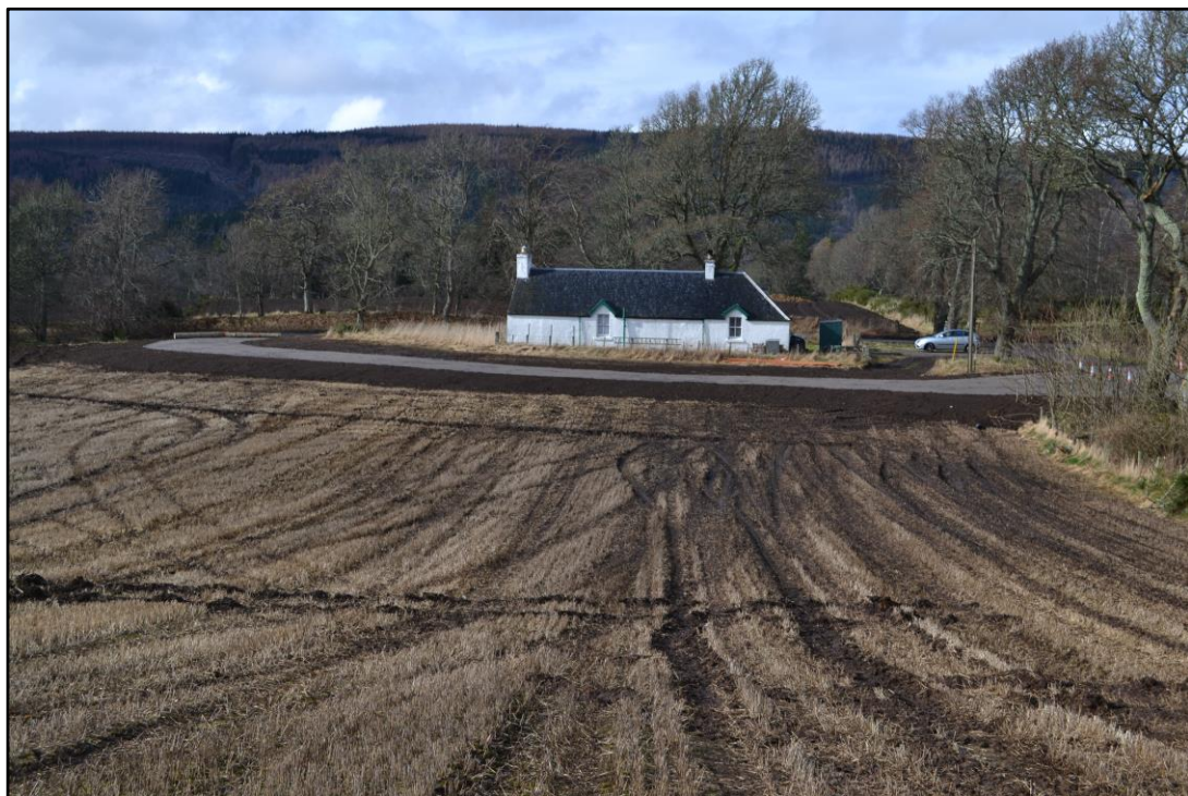
Plate 3: New access track
