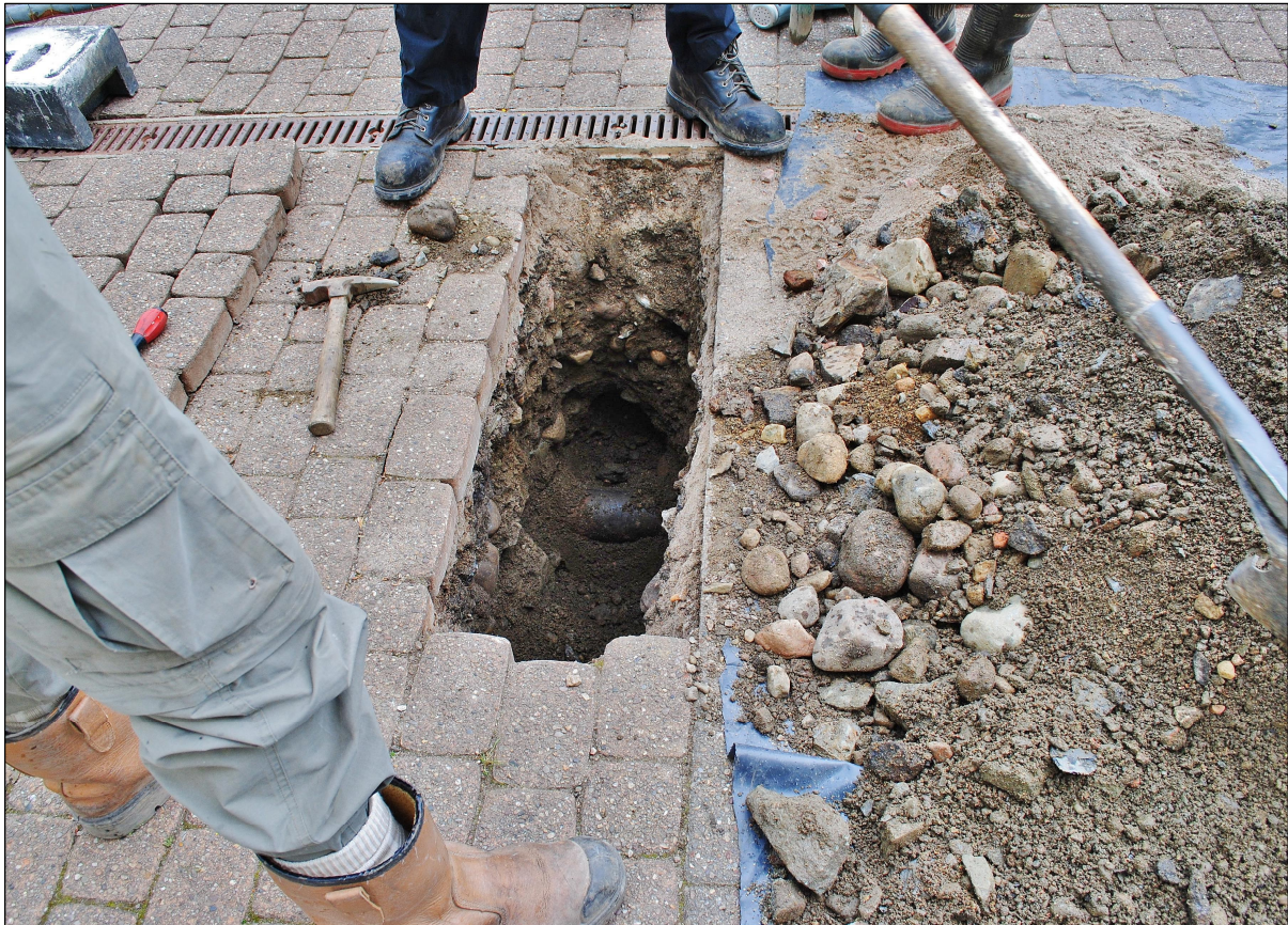
Plate 3 TT13/01, utilities pipeline at the base of the trench
