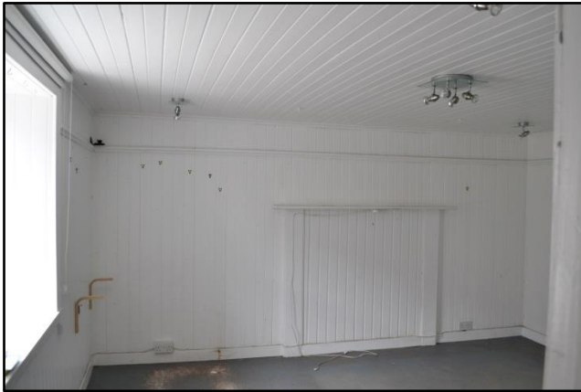
Plate 1: Room 1 with blocked fireplace in west wall.
