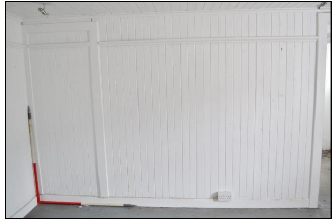
Plate 2: Room 1 with blocked doorway in east wall.
