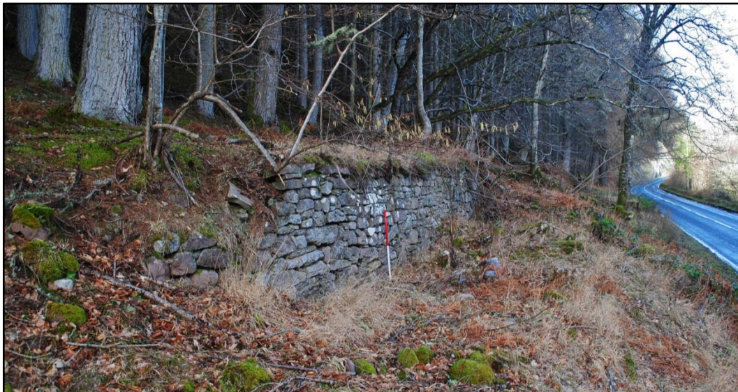
Plate 7: Site 35 showing the NW wall revetted into the slope.
