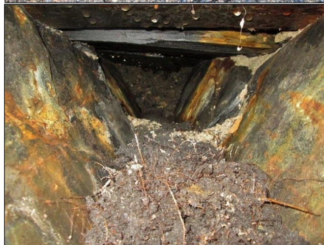
Plate 11 (top) Feature 3 drain: SW-facing photo of the drain after excavation
