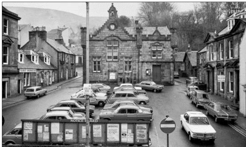
Plate 2 The Cameron Square car park, before the Town House was destroyed, facing SE; photograph taken in 1973 by T. Kenneth Mackenzie 15
