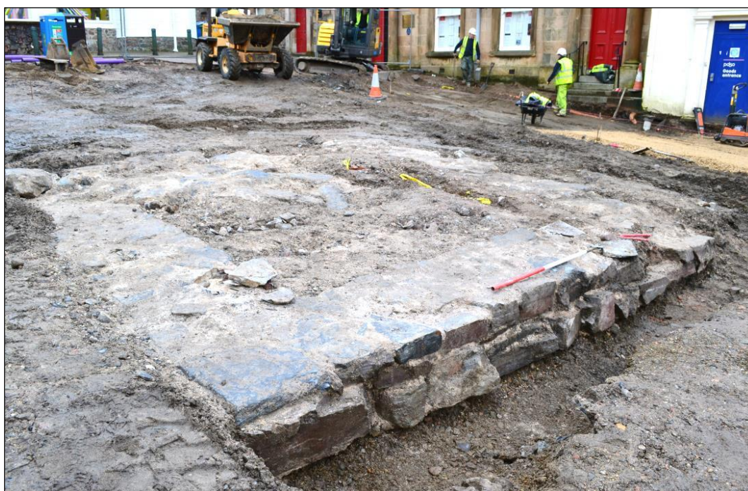
Plate 9 Remains of the Kennedy monument plinth and NW-facing wall profile, facing S
