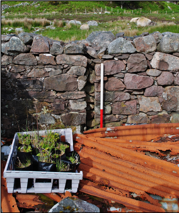
Plate 2: Cruck-slot, south side of western wall
