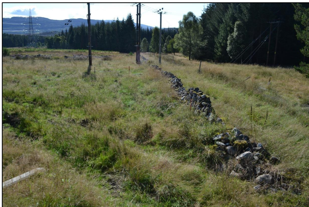
Plate 1: The drystone dyke looking S from the SW corner of the existing substation
