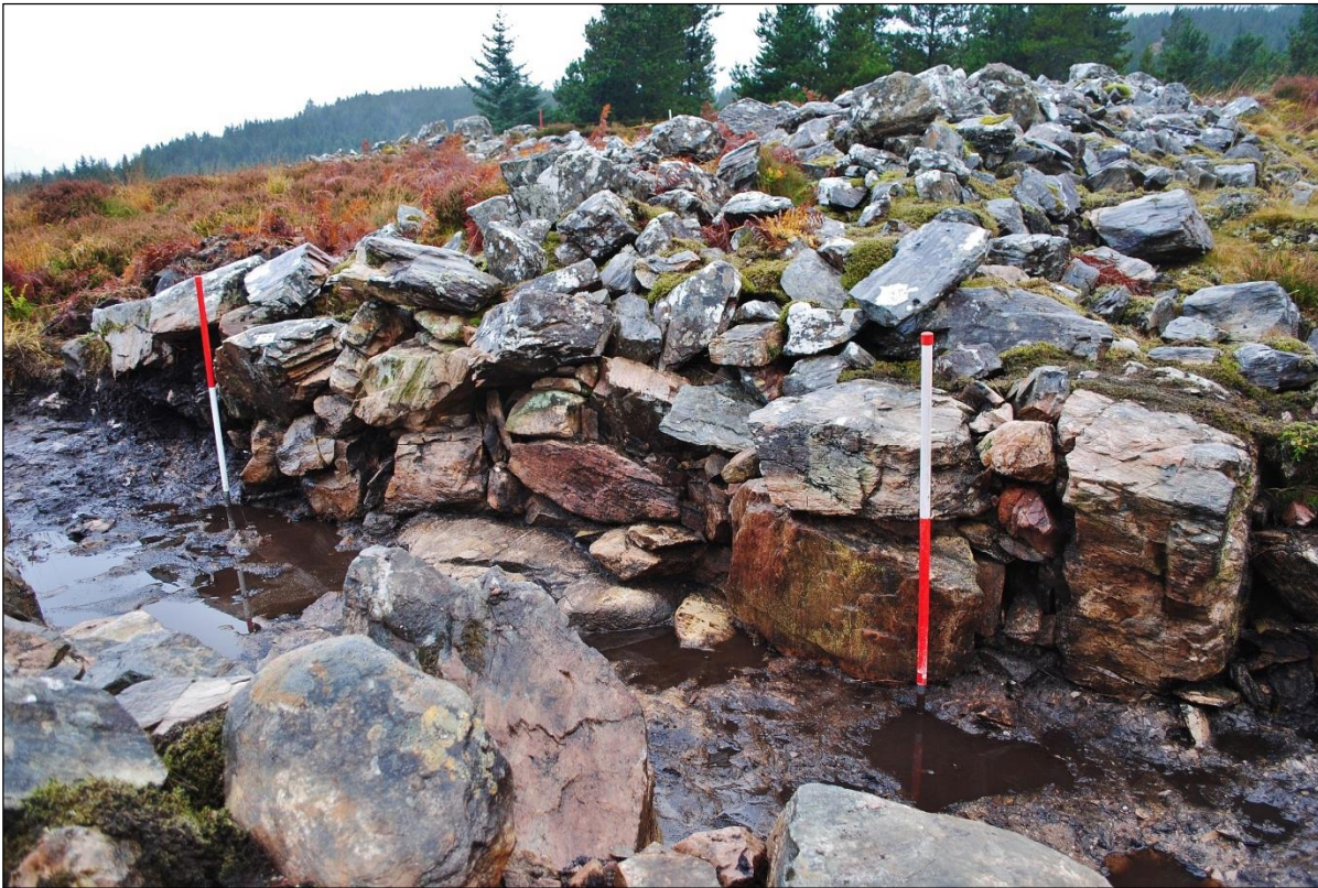
Plate 7: Close view of the NW entrance passage wall, door check visible behind the front 1m pole, facing W
