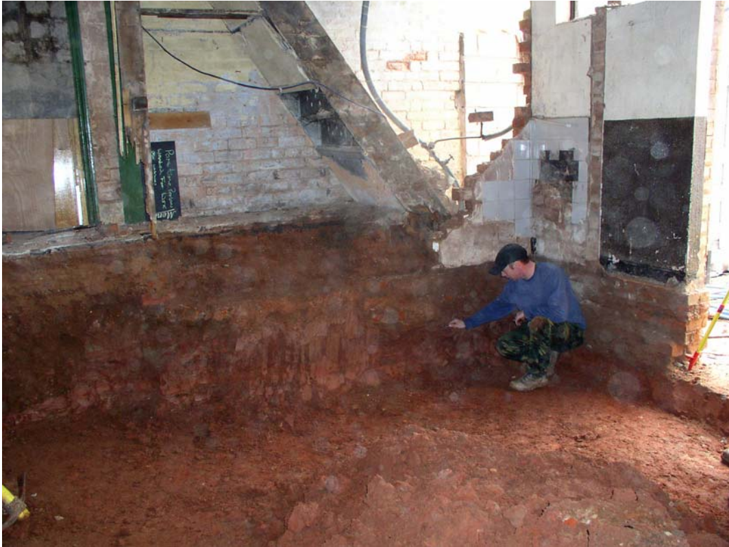
Fig 4: The internal reduced floor after excavation
