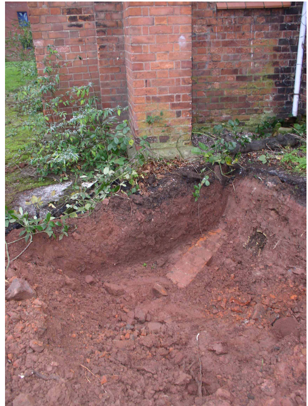
Fig. 13: Trench 3 drains 305 and 307
