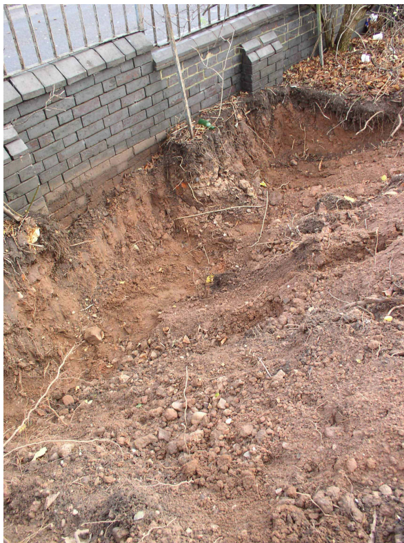
Fig. 10: Trench 1C looking south-east
