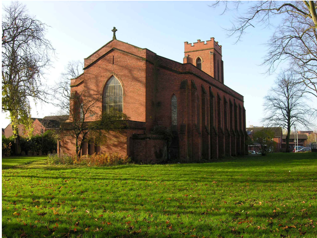
Fig. 24: View of church looking south-west
