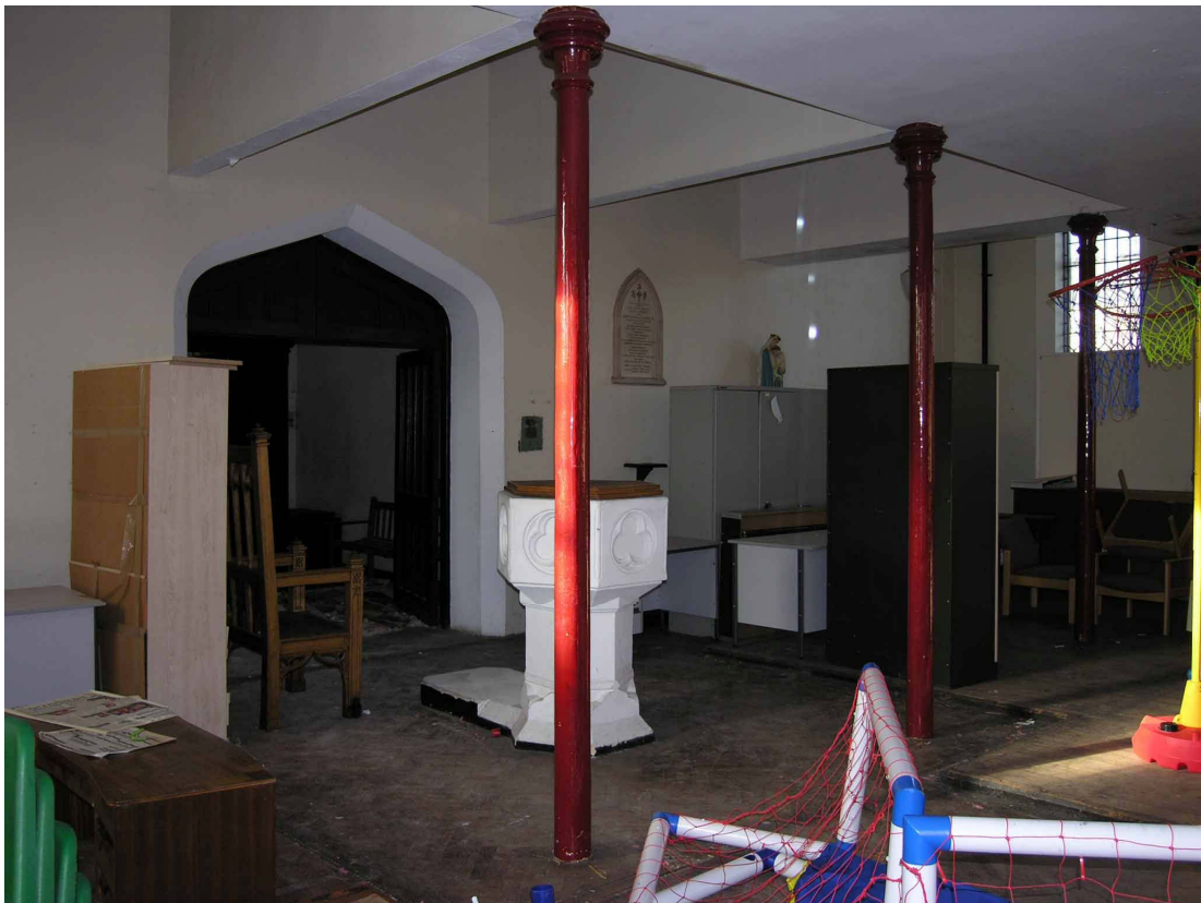
Fig. 41: Columns supporting gallery
