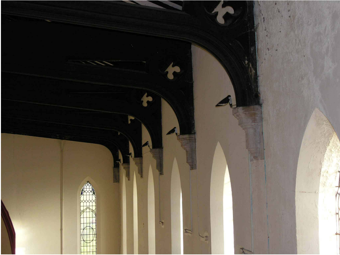
Fig. 38: Corbels supporting roof timbers
