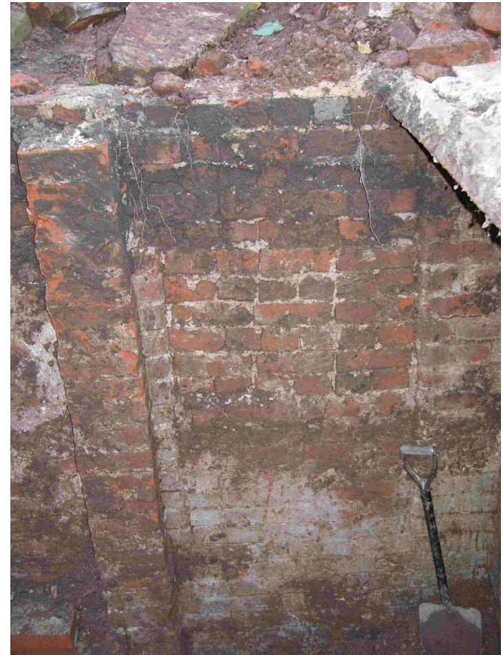
Fig. 20: Entrance to vault
