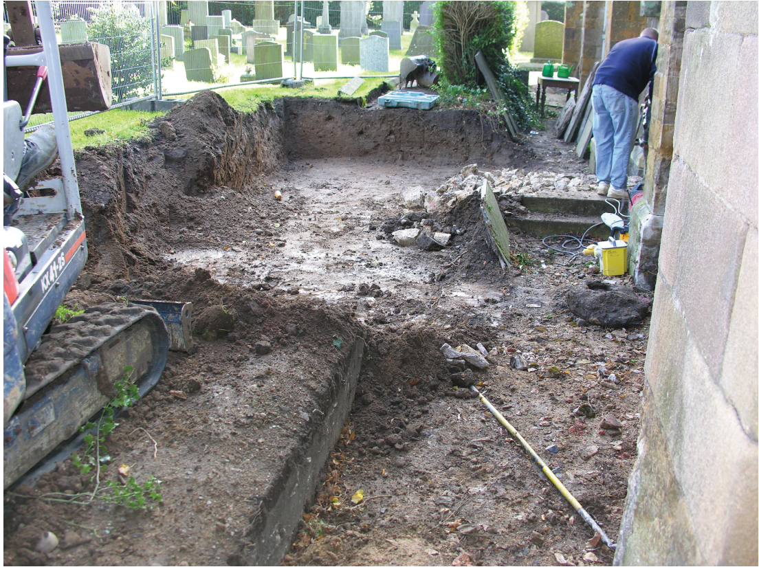
Fig. 2: Ground reduction looking east
