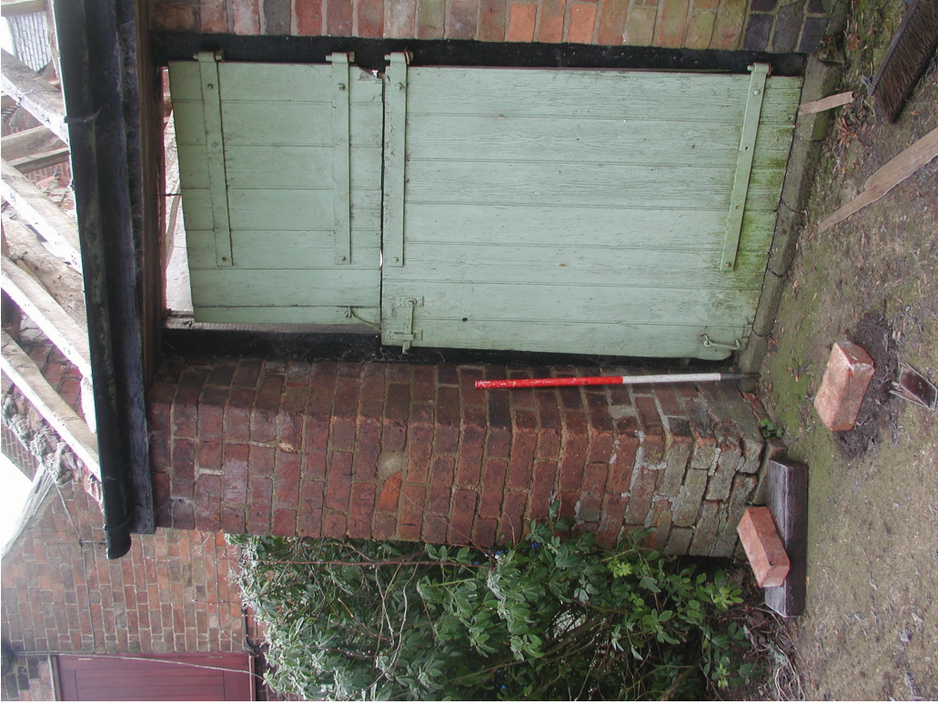
Fig. 7: Stable door and corner of wall
