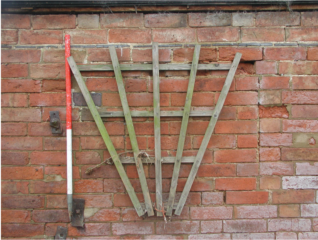
Fig. 11: Blocked window (south-east wall)
