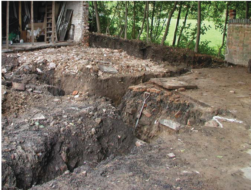
Fig. 5: Overall view of site looking west
