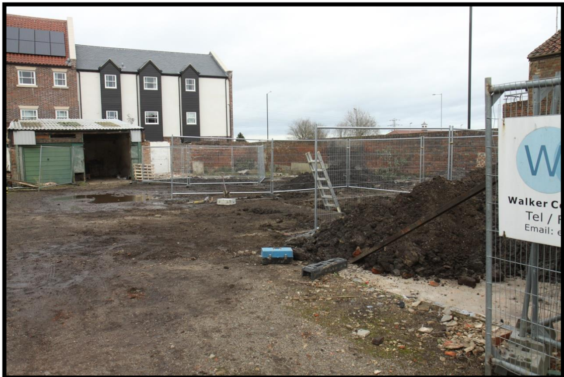
Plate 2: General view of site from Southwest.
