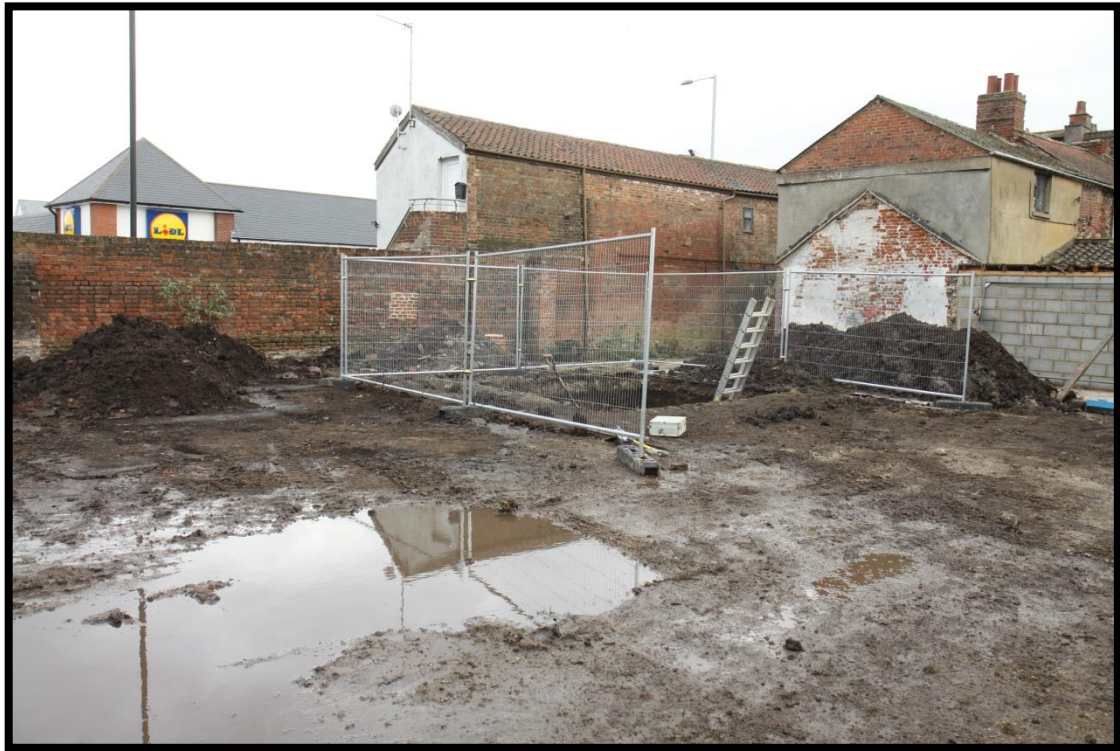
Plate 3: General view of Trench 2 location from Northwest.
