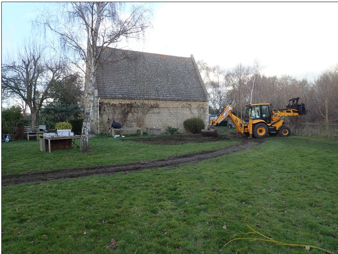
Plate 6: Backfilling the trench, looking north
