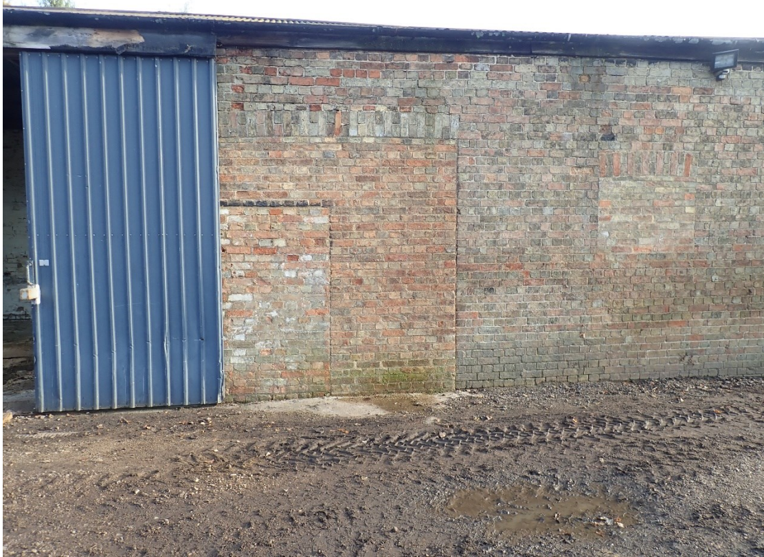
Plate 17: View of west face segment of workshop building, looking east
