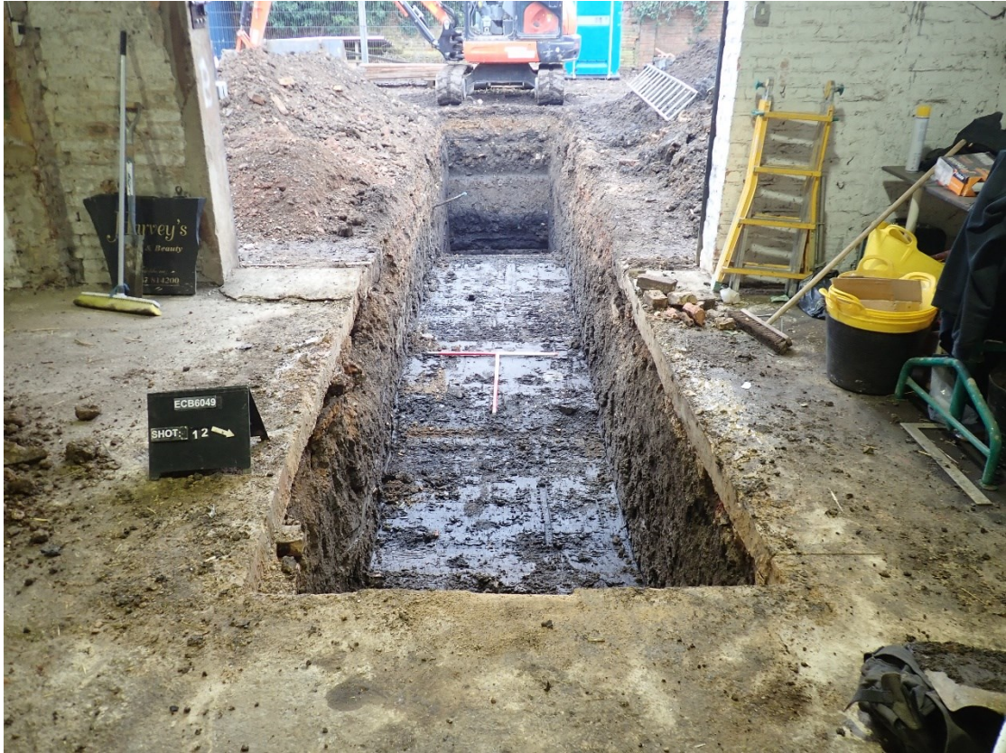
Plate 7: Overall view of Trench 2, looking west north-west, 2x1m scales
