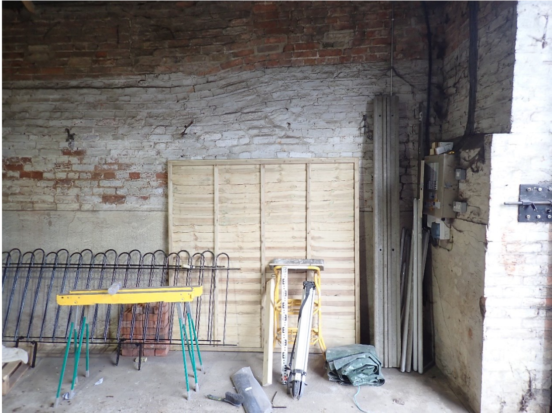
Plate 19: View of east inner wall detail of workshop building, looking east
