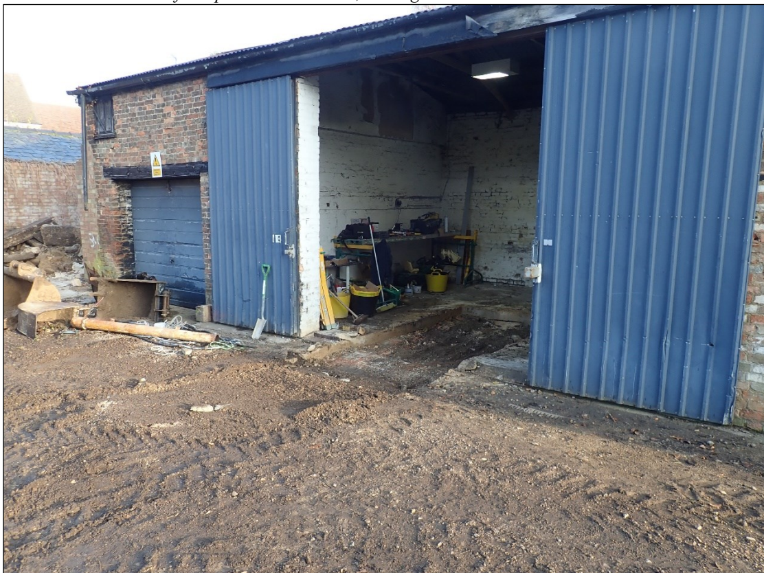
Plate 2: General view of site prior to excavation, looking north-east
