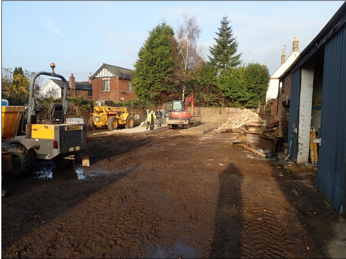
Plate 1: General view of site prior to excavation, looking north-west
