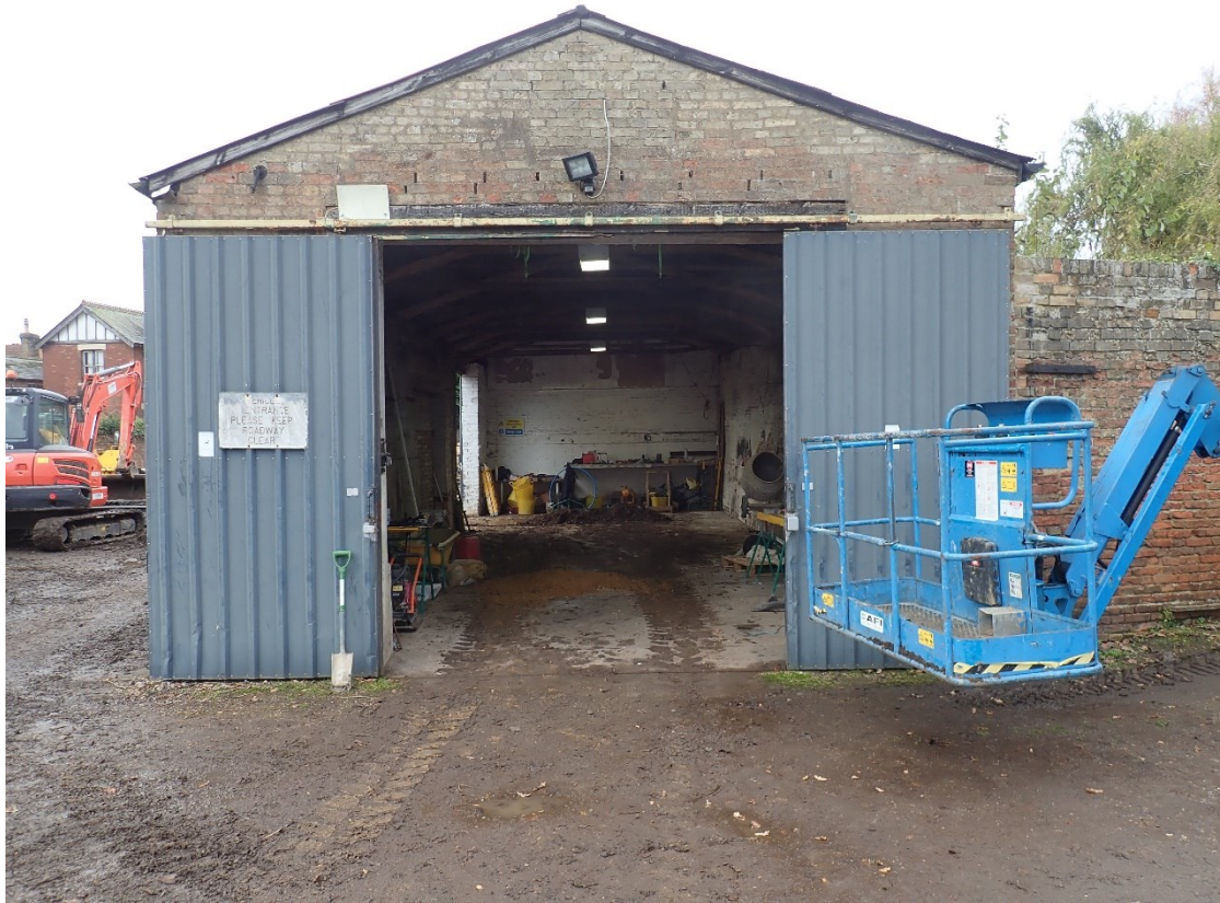
Plate 15: View south face of workshop building, located on the south-east corner of site, looking north
