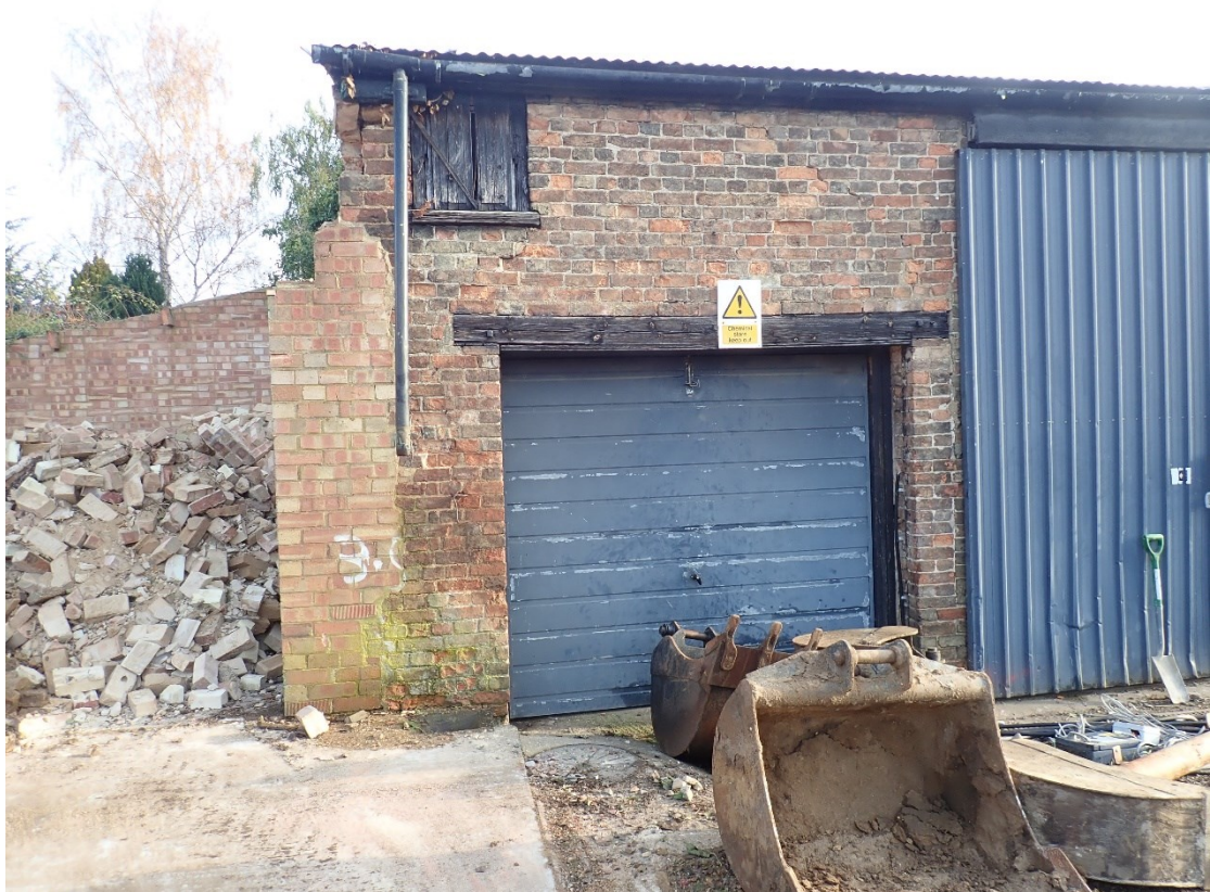
Plate 16: View of west elevation of workshop building, looking south-east
