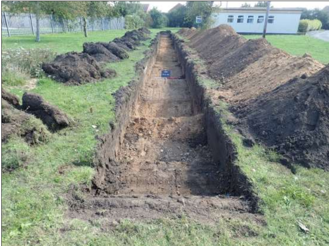
Plate 1: Trench 1 looking north-east. 2 x 1m scales.
