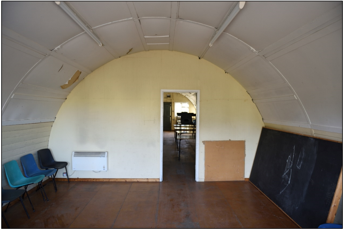
Plate 8: Interior of Block 36, northern room, looking south-west
