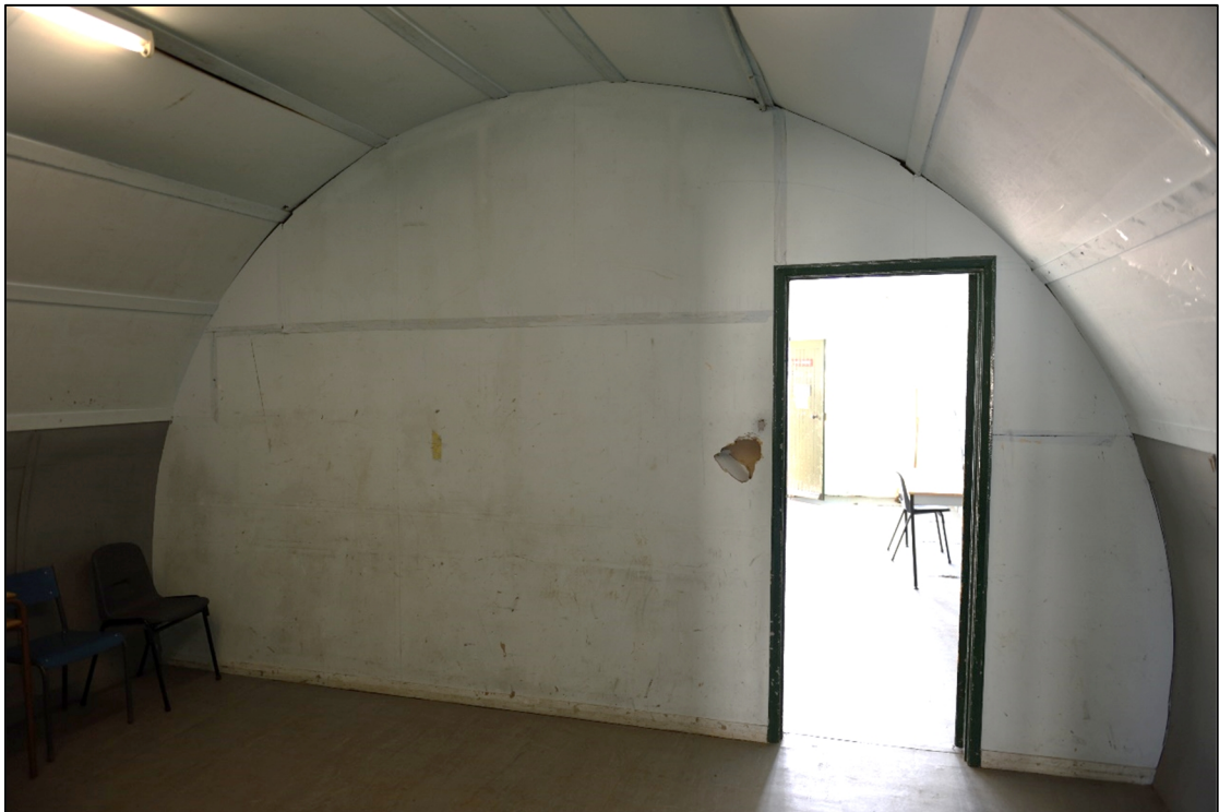
Plate 23: Interior of Block 63, central room, looking south-east
