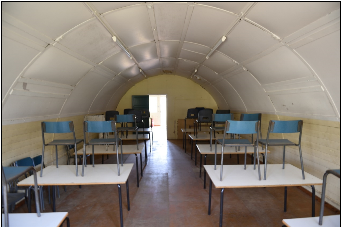
Plate 9: Interior of Block 36, southern room, looking north-east
