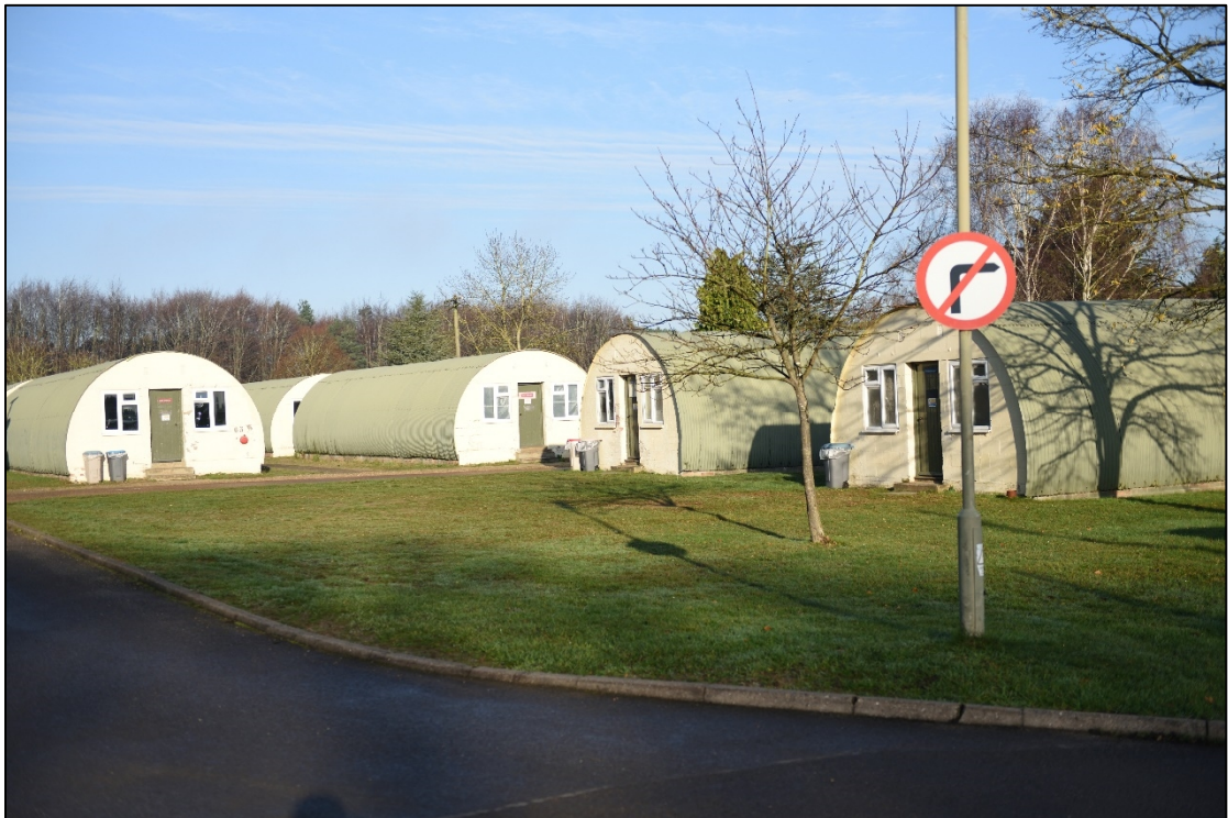
Plate 13: View of Blocks 47, 48 (right), 63 and 49 (left), looking north
