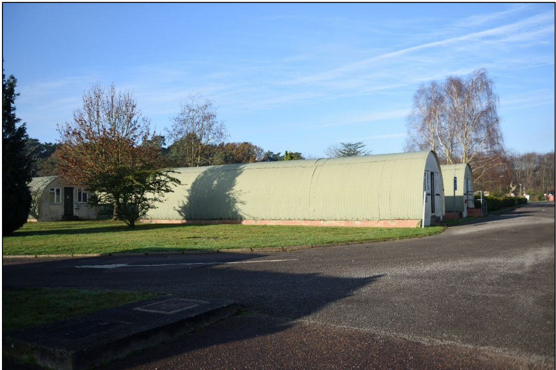
Plate 11: View of Blocks 35, 36 (right), 47 and 48 (left), looking north-west
