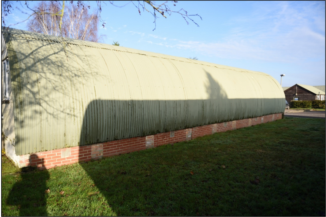
Plate 6: Detail of south side of Block 35, looking north
