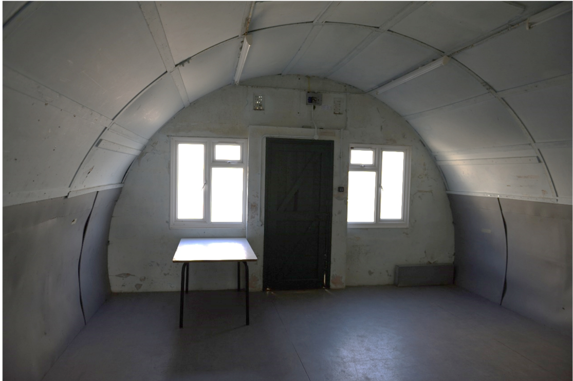
Plate 24: Interior of Block 63, north room, looking north-west
