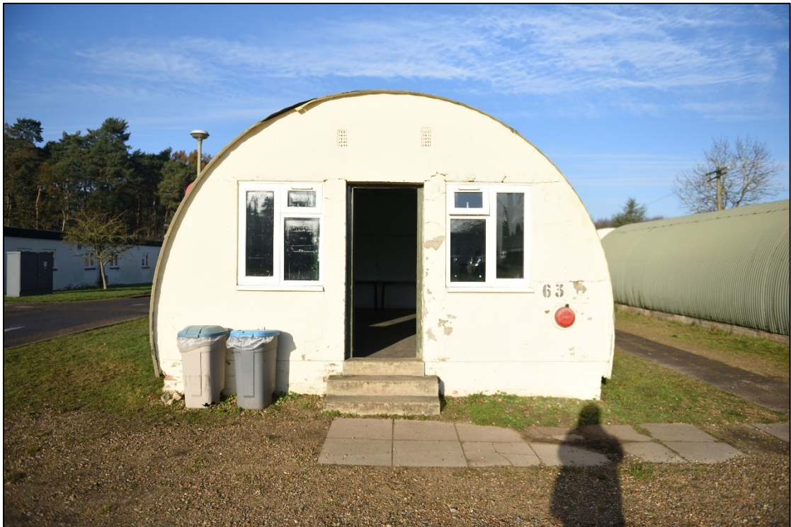
Plate 21: South-east elevation of Blok 63, looking north-west
