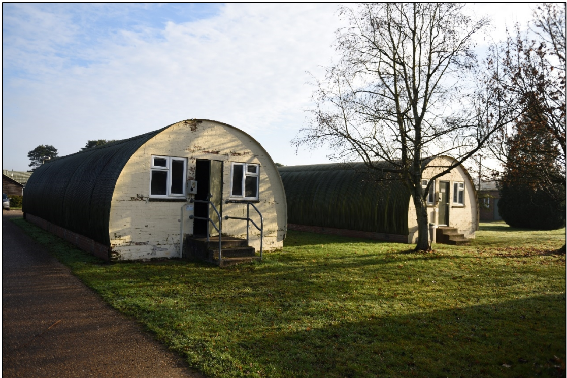
Plate 5: South-west elevation of Blocks 35 (left) and 36 (right), looking north-east
