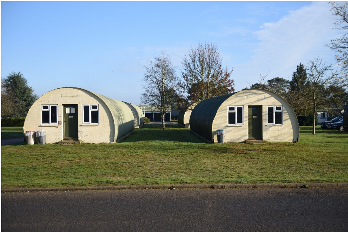
Plate 15: South-west elevations of Blocks 47 (right) and 48 (left), looking north-east
