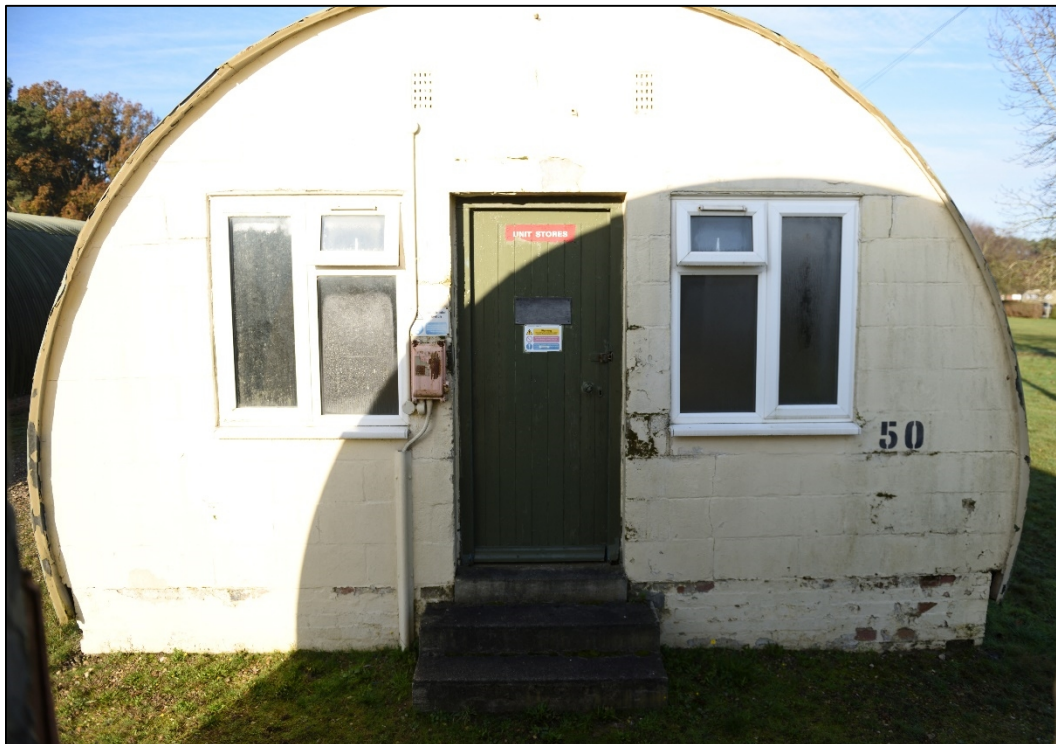
Plate 25: South-east elevation of Block 50, looking north-west
