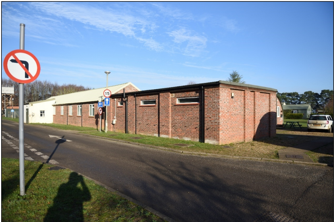
Plate 27: Building north-west of Blocks 62 and 50, looking north
