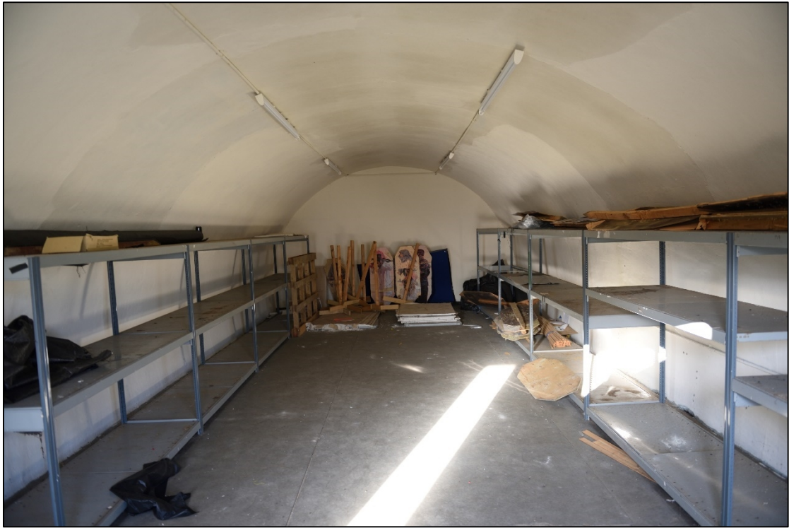
Plate 26: Interior of Block 50, looking north-west
