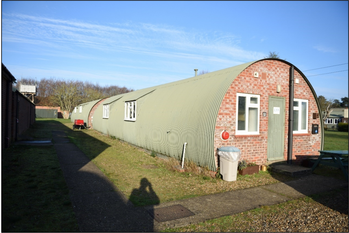
Plate 28: View of blocks at the north-west corner of the site, facing the north-west of blocks 62 and 50, looking north
