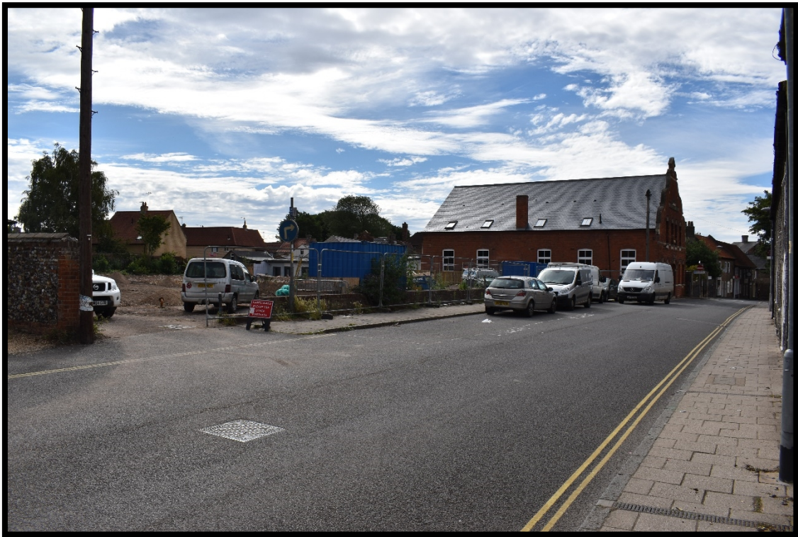
Plate 1: View of development site from the Earl Street frontage facing southeast.
