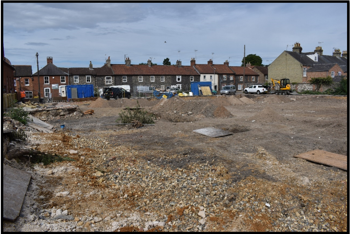
Plate 5: General view of the development site facing southwest.
