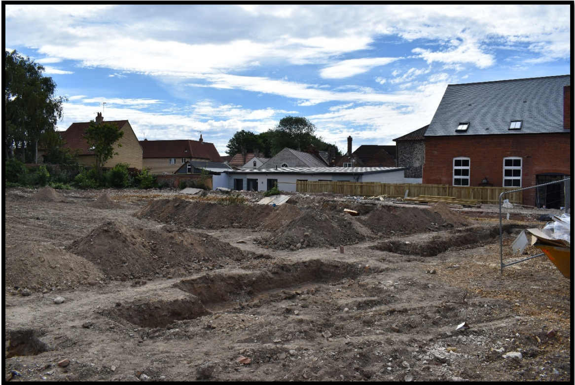
Plate 3: General view of the development site facing southeast.
