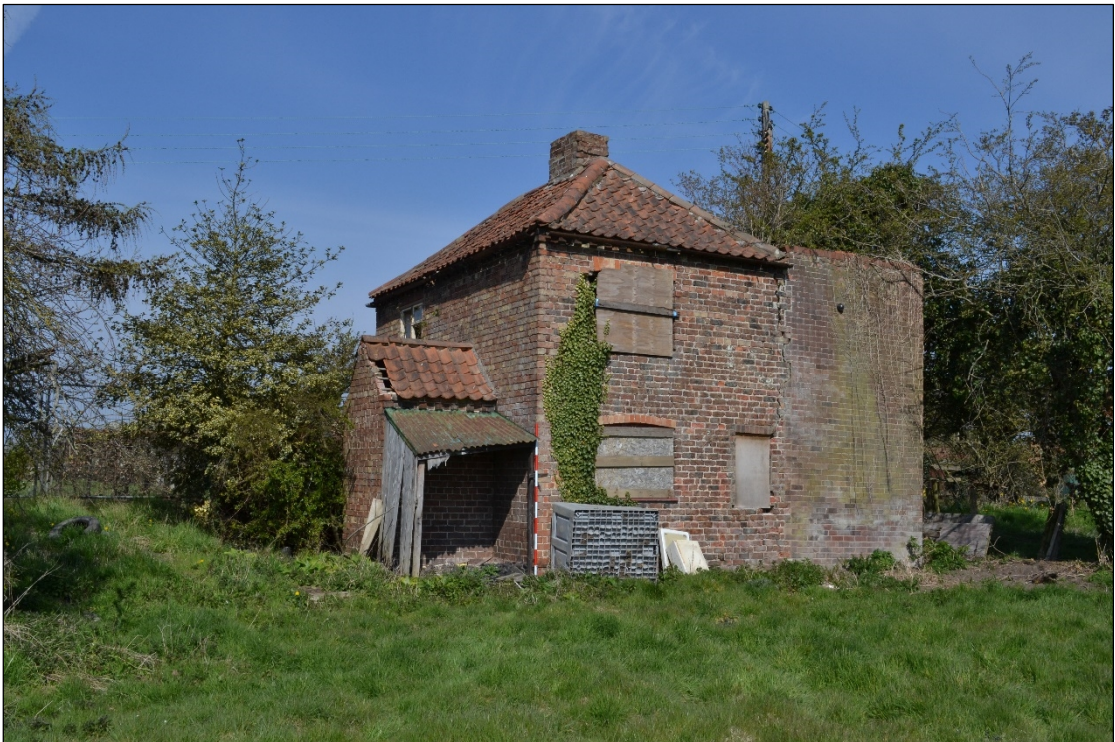
Plate 10: Derelict cottage 'Welbourn', looking north-west. 2m scale
