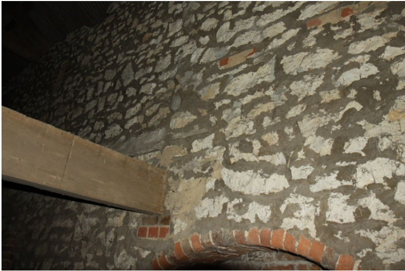
Plate 45: Surviving beam and plaster on southwest wall
