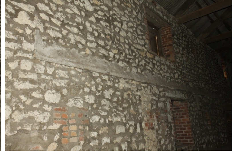
Plate 41: Building 5 - plaster on interior of southwest wall
