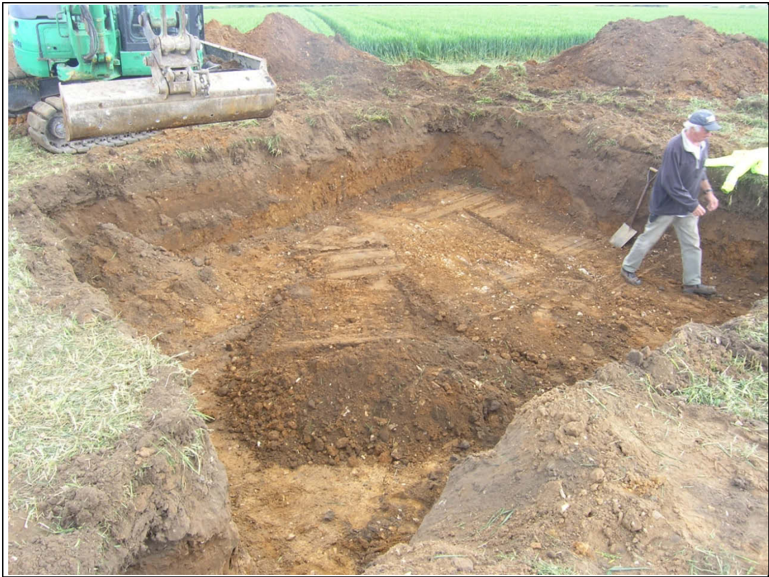
Plate 1: Excavation for the base of the turbine, looking southeast
