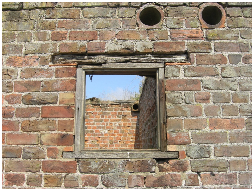
Plate 13: Building 2 – high level opening to Unit A
