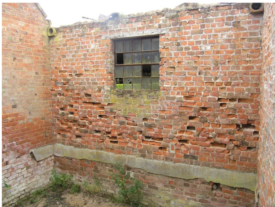
Plate 15: Building 2 – rear of Unit A
