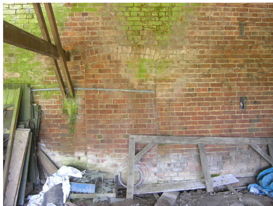
Plate 5: Blocked in doorway to rear of Building 1 (view from Building 3)
