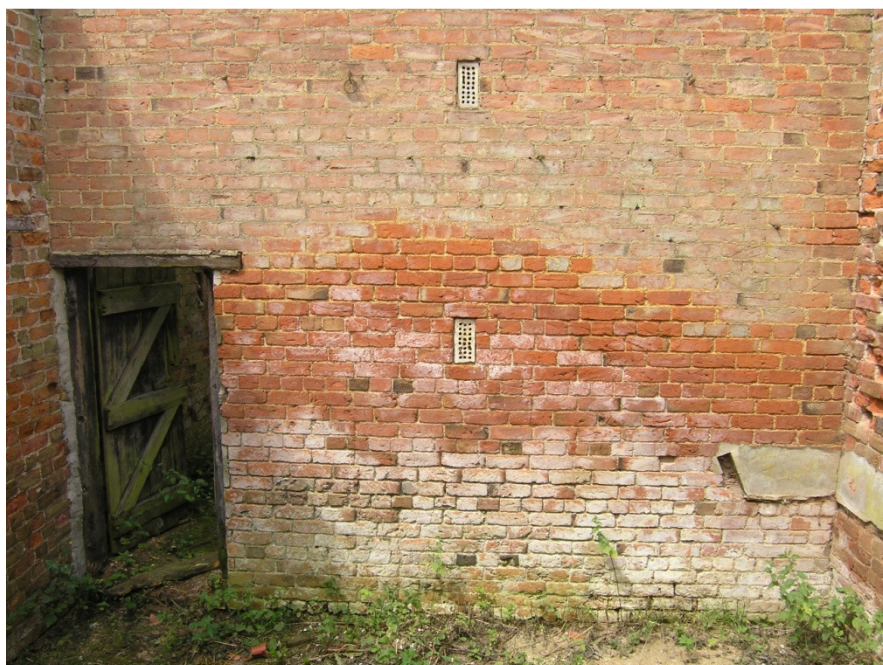
Plate 4: Building 1 – lower extent of southeast wall as seen from inside Building 2
