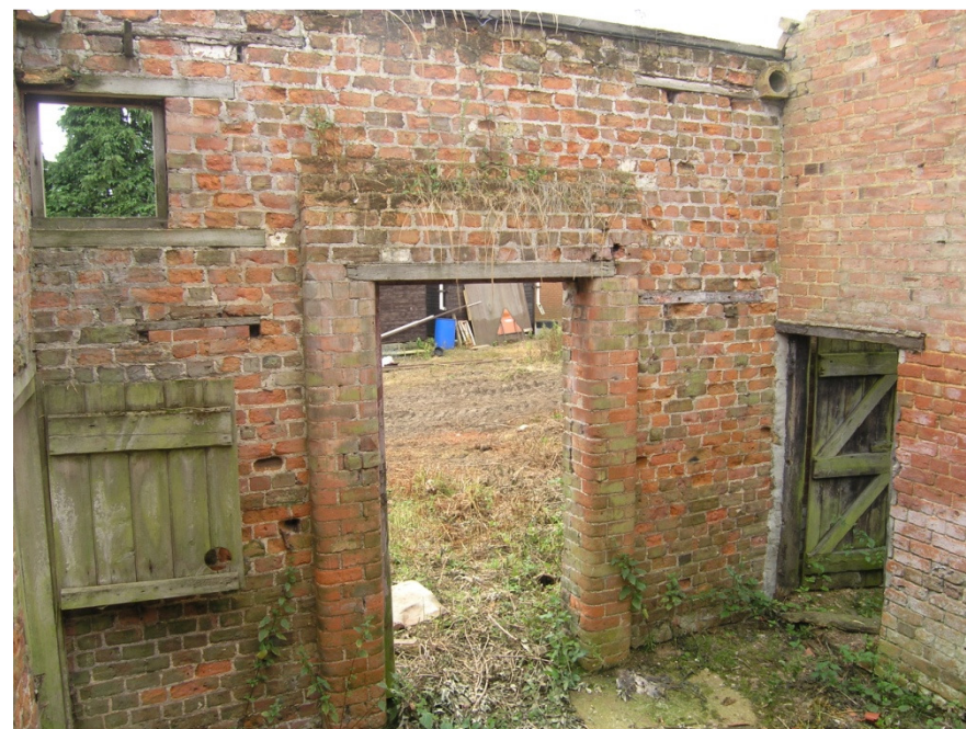
Plate 18: Building 2, Unit A – southwest side
