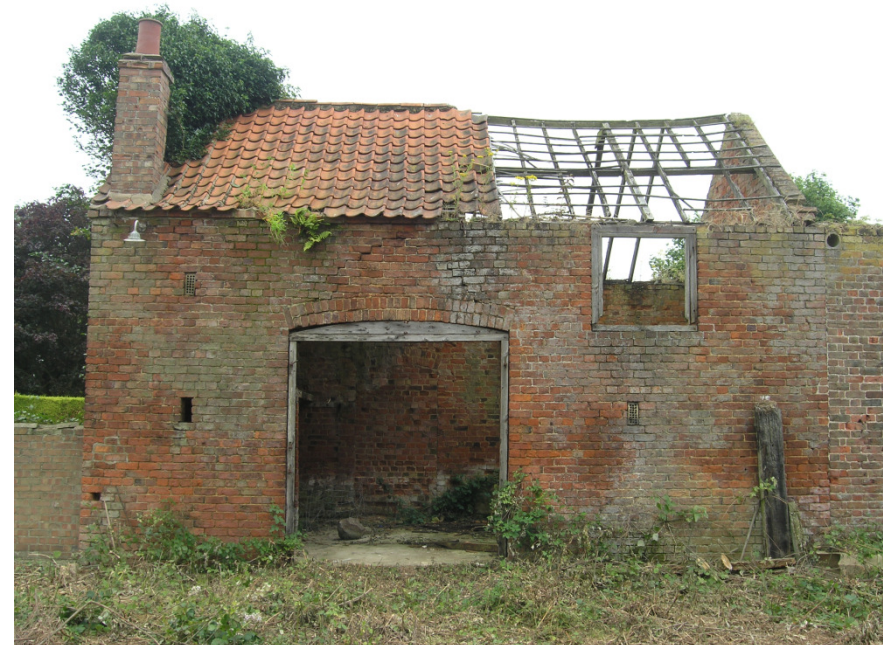
Plate 3: Front elevation of Building 1
