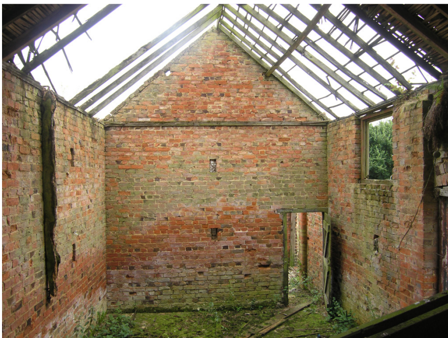
Plate 6: Interior of Building 1, southeast end
