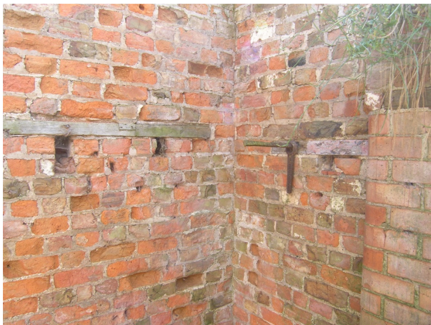
Plate 23: Building 2, Unit B – detail adjacent to the doorway
