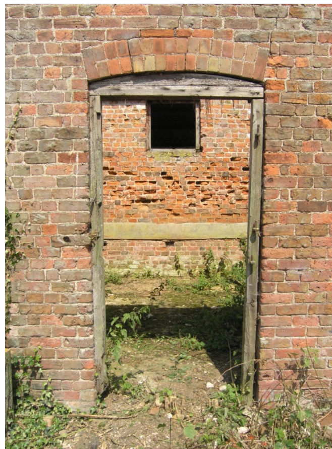
Plate 14 – Building 2 – door to Unit B
