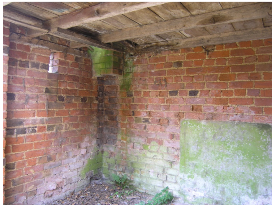
Plate 9: Base of chimney at western corner of Building 1
