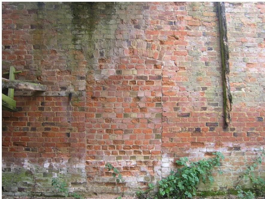
Plate 8: Blocked in doorway seen from the inside of Building 1
