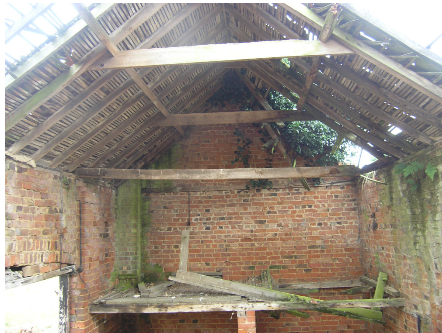
Plate 11: Surviving part of the roof in Building 1
