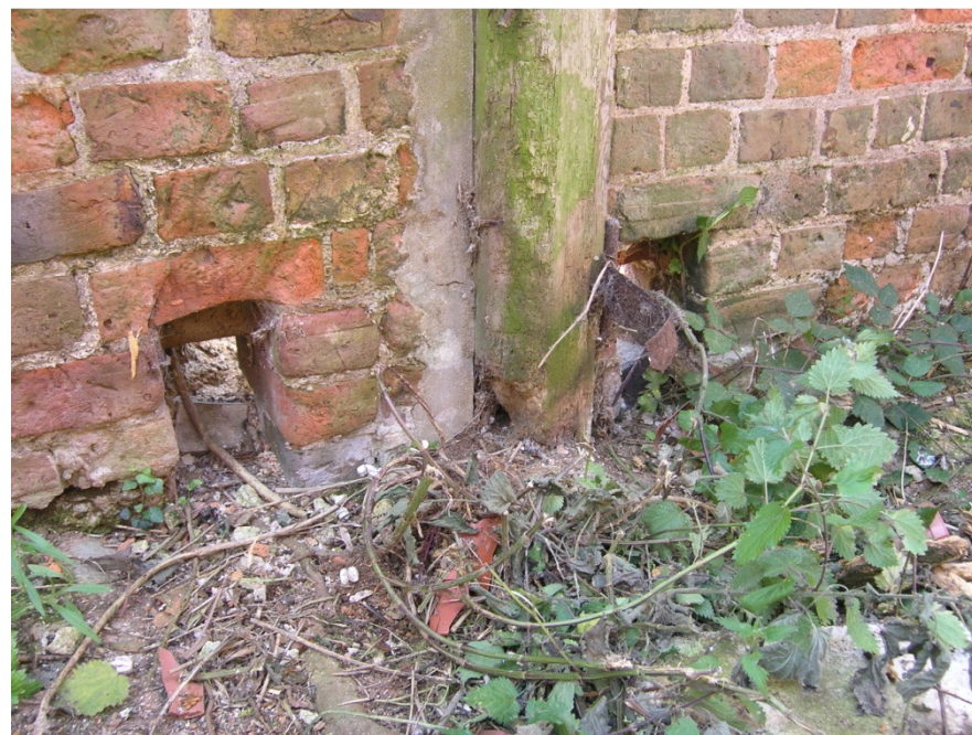
Plate 26: Building 2, Units A & B – floor level openings
