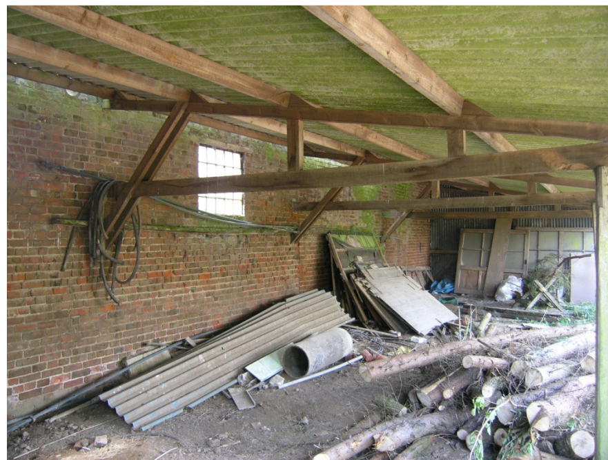
Plate 28: Building 3 – interior, looking west
