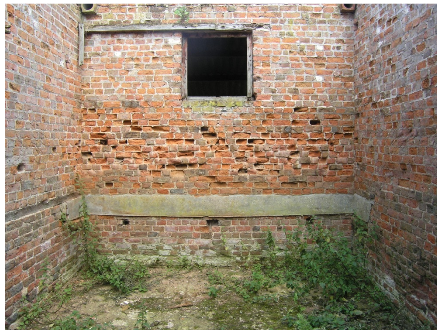
Plate 20: Building 2, rear of Unit B
