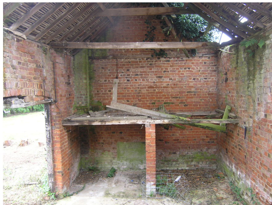
Plate 7: Interior of Building 1 – northwest end
