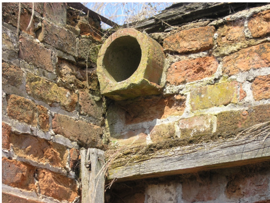
Plate 25: Vent at in the rear wall of Unit B
