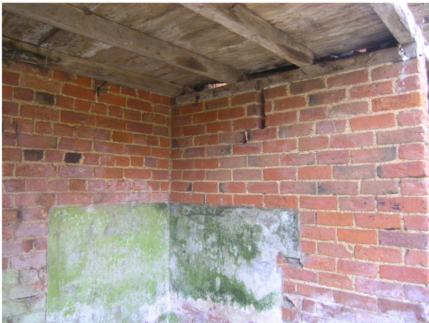
Plate 10: Lined area adjacent to the chimney in Building 1
