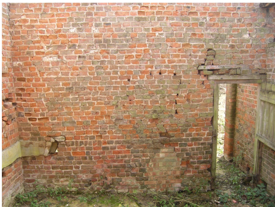
Plate 17: Building 2, Unit A – internal wall and door to Unit B
