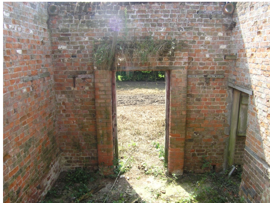
Plate 22 Building 2, Unit B – southwest side
