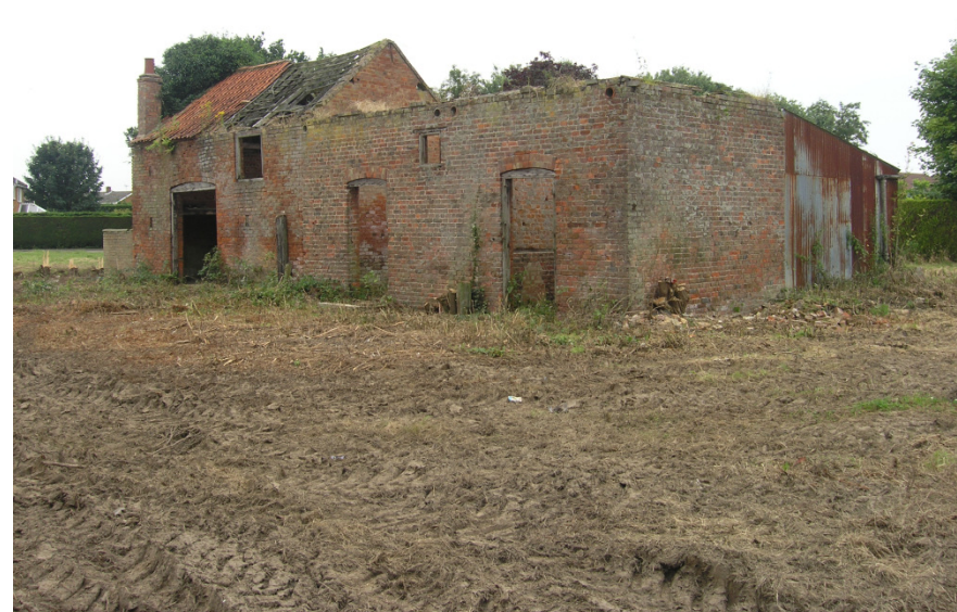
Plate 12: Building 2 in the foreground, viewed from the south
