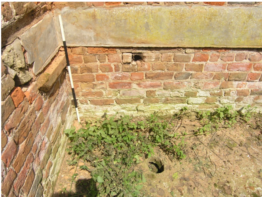
Plate 21: Building 2, Unit B – northwest end of manger (1m scale)
