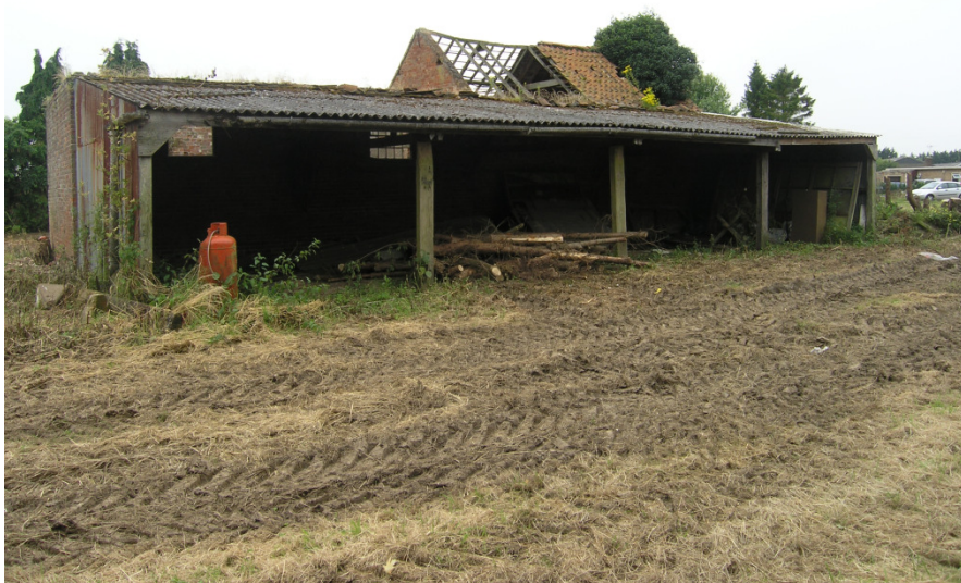
Plate 27: Building 3 – view from the east, looking west
