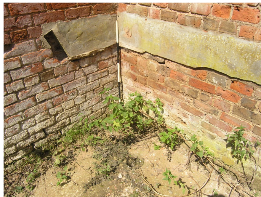
Plate 16: Building 2 – northwest end of the manger in Unit A (1m scale)
