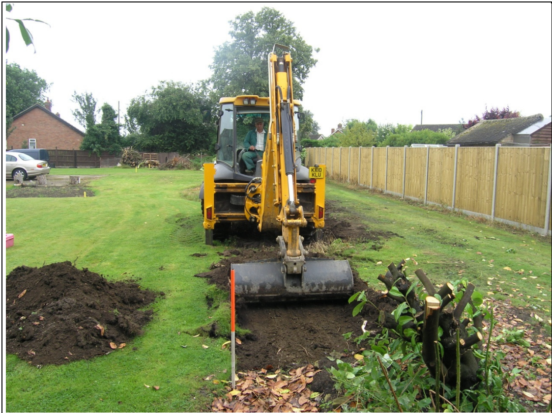
Plate 1 - Topsoil removal in progress, looking southeast
