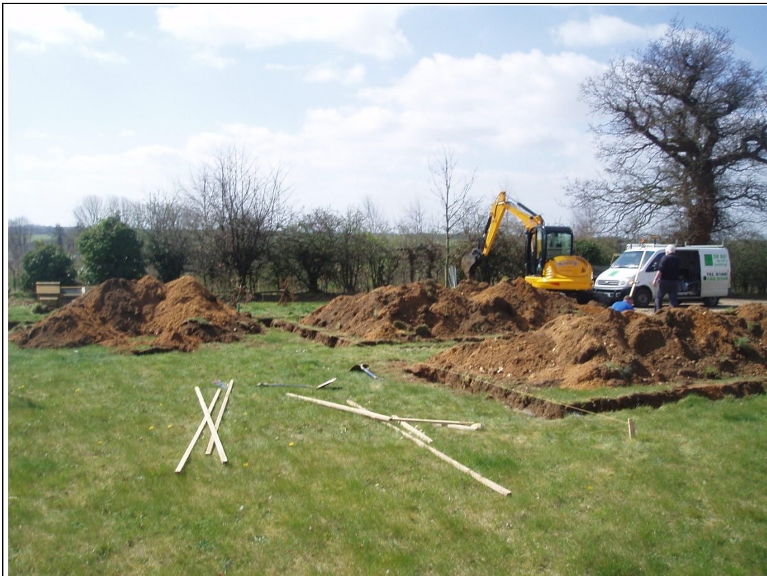
Plate 2: View showing site during excavation of foundations. Facing South.
