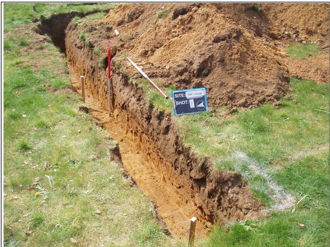
Plate 6: View showing north part of foundation
