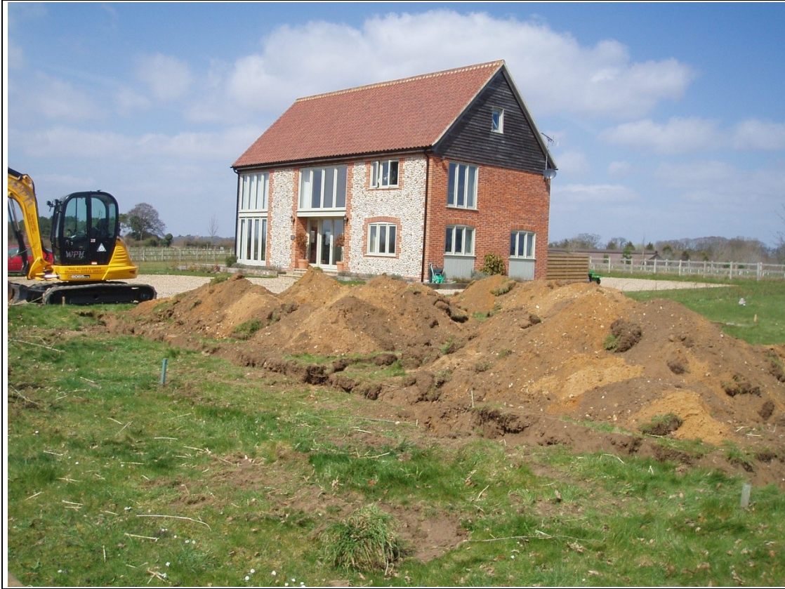
Plate 3: View showing excavated foundations. Facing northwest. Oakhill Barn in background.
