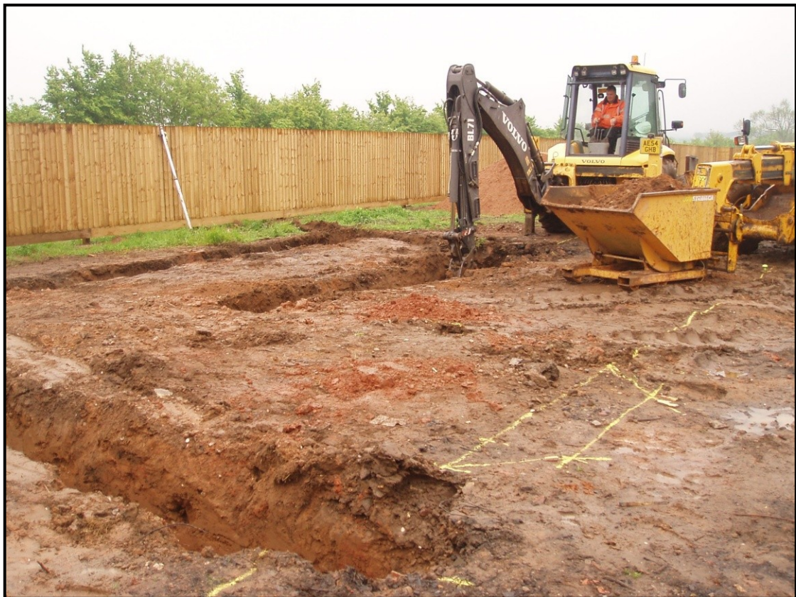
Plate 10 - Excavation of foundation trenches
