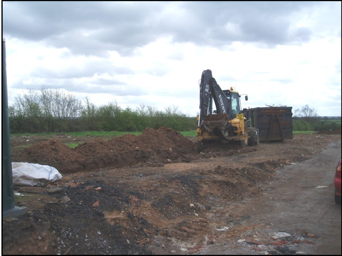
Plate 3 - Excavation of Evaluation Trench 1, looking southeast
