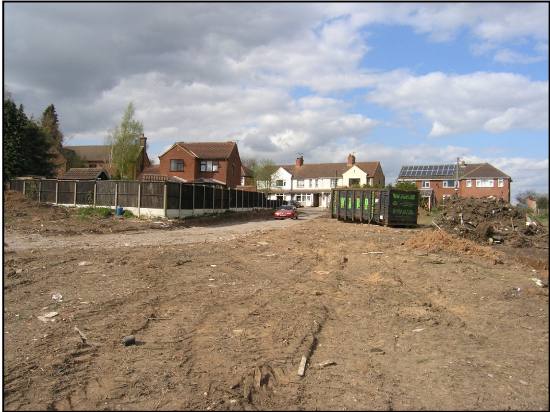
Plate 1 – General view of the site from the southeast corner, facing north
