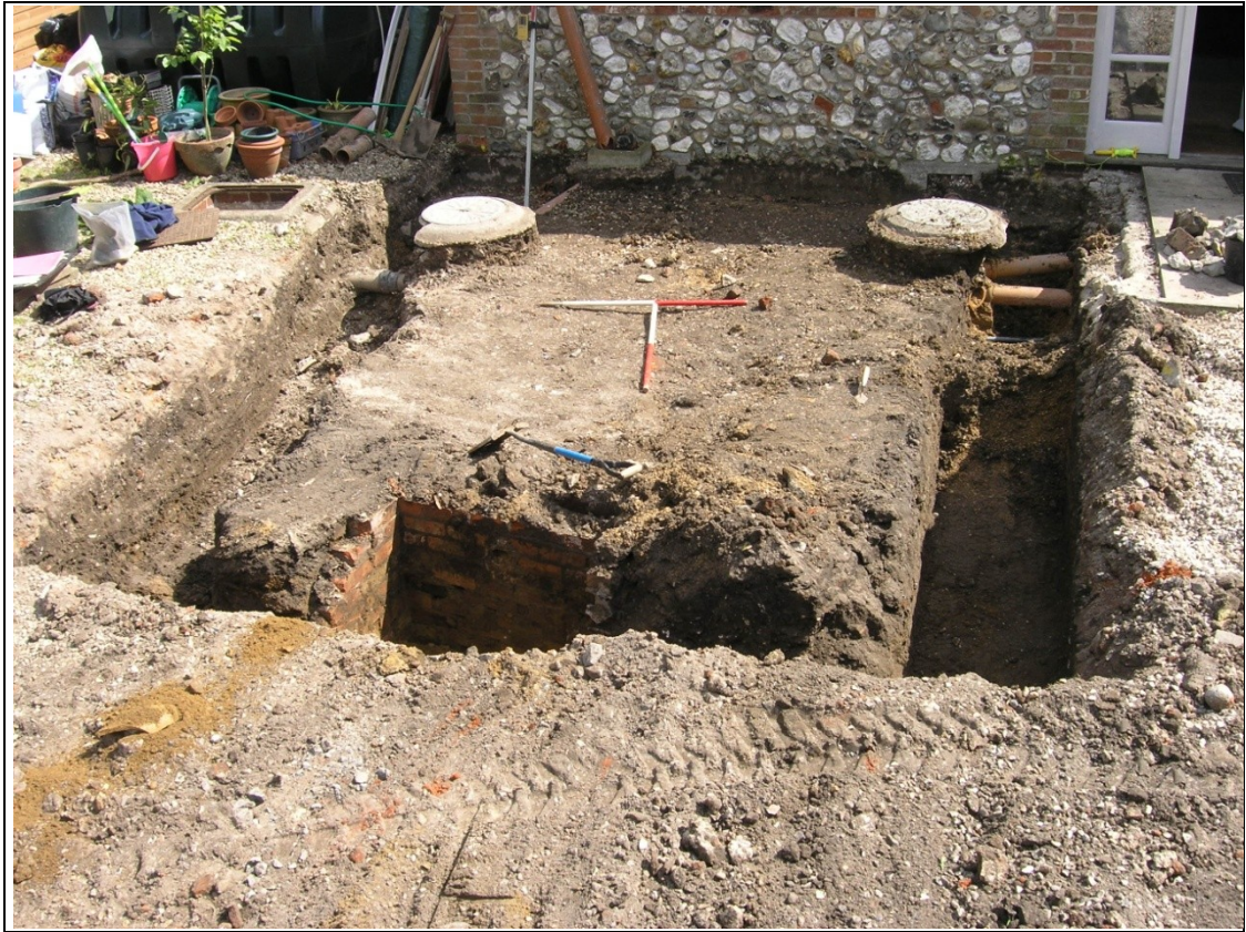
Plate 3: View showing fully excavated foundations. Facing South.
