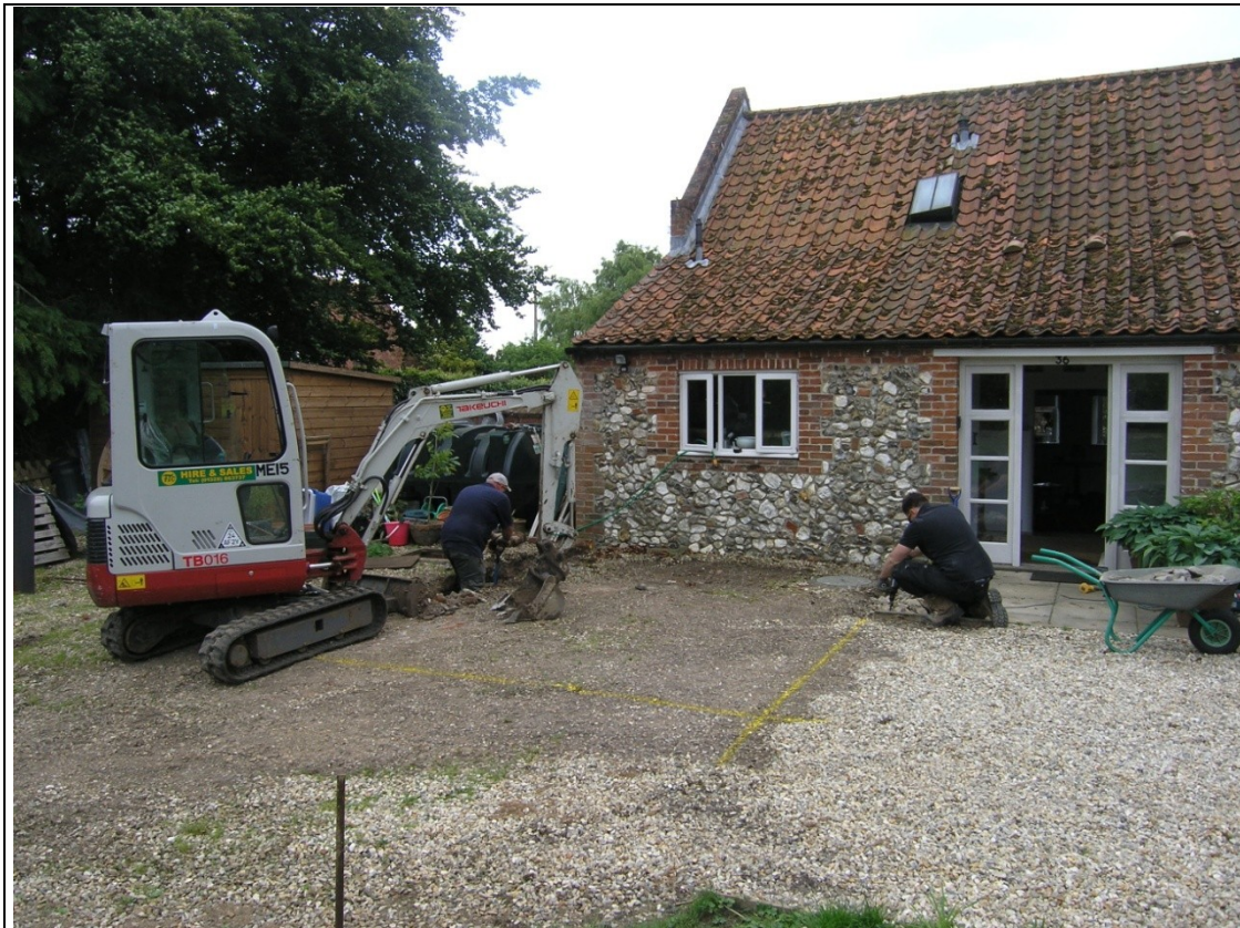
Plate 2: View showing site during excavation of foundations. Facing Southeast.
