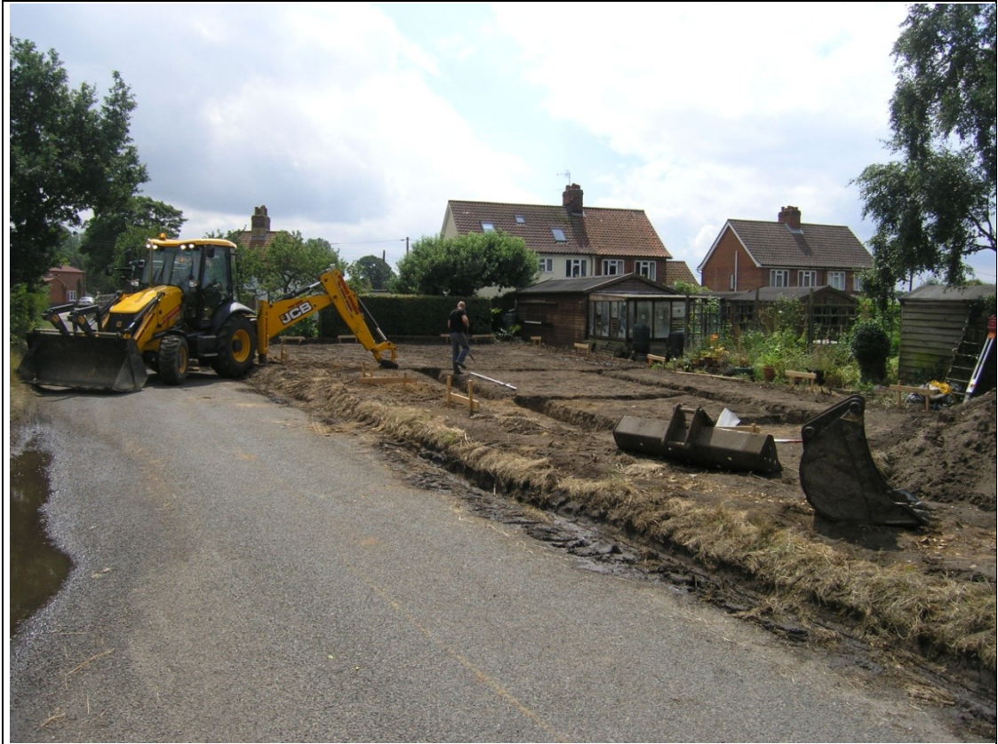
Plate 1: View of the site during excavation of foundations. Facing southwest
