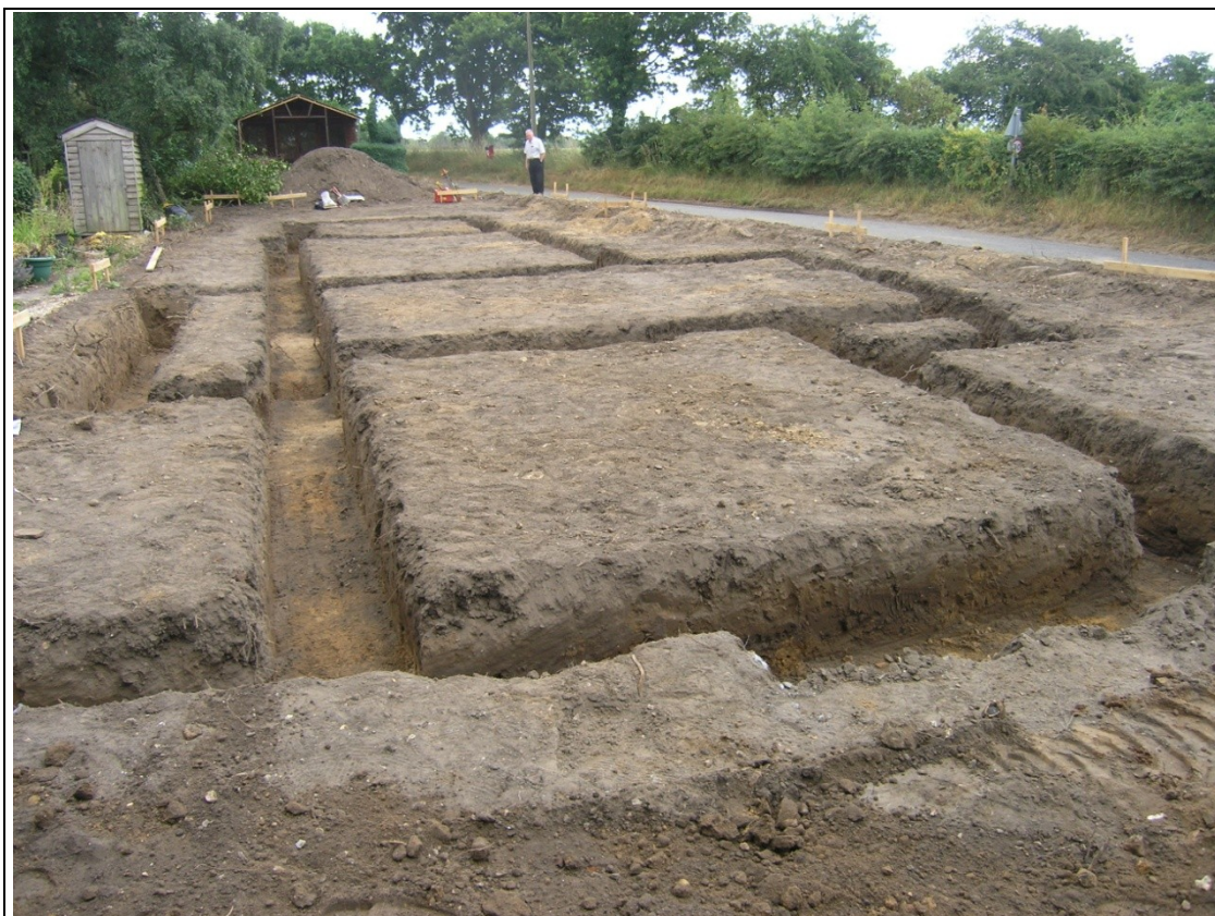
Plate 5: View of fully excavated foundations. Facing north.
