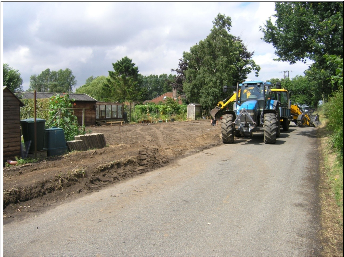
Plate 2: View of the site during excavation of foundations. Facing northwest.
