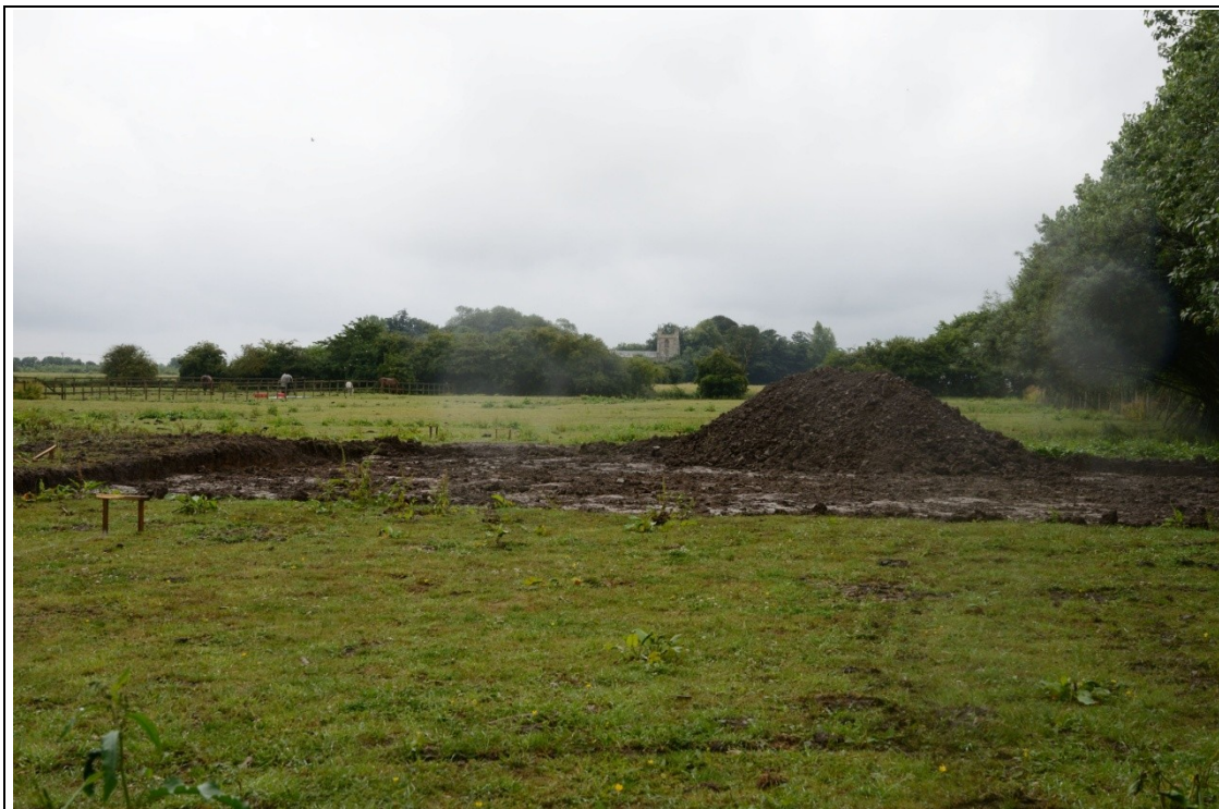
Plate 2: Area of stables and yard with overburden removed, looking south
