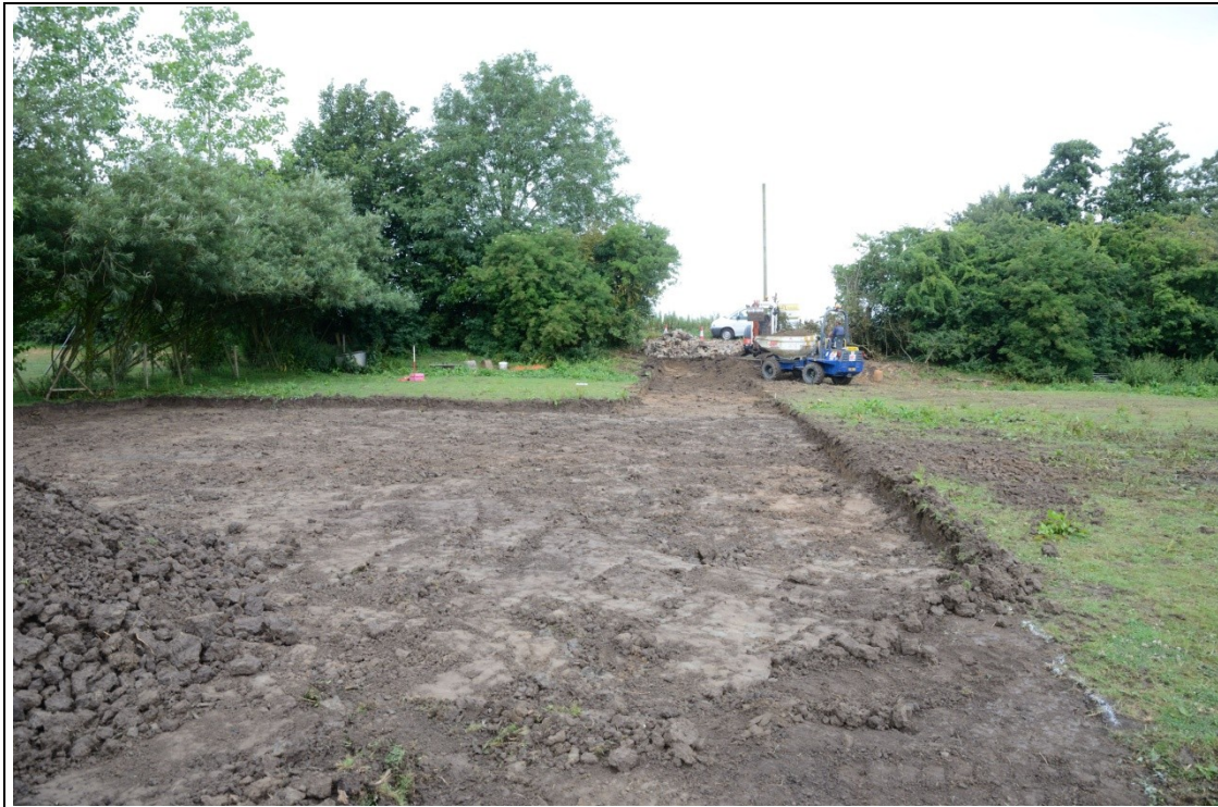
Plate 1: Work in progress, looking north
