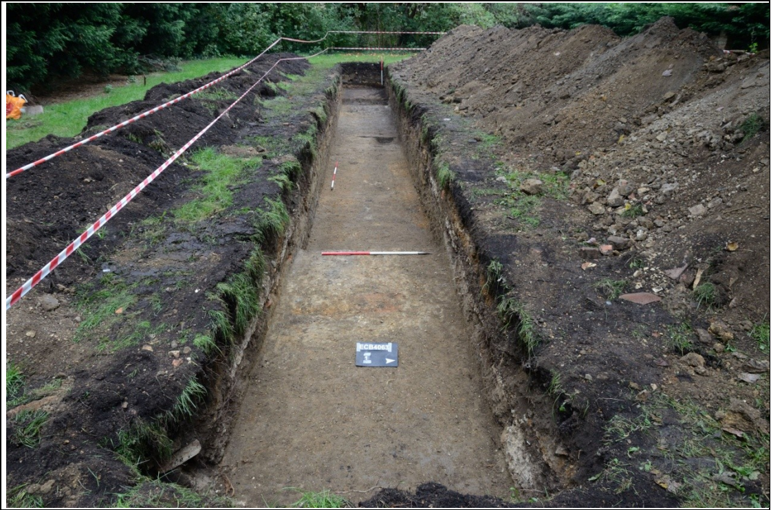
Plate 3: Trench 2, looking west; 2 x 1m and 2m scales
