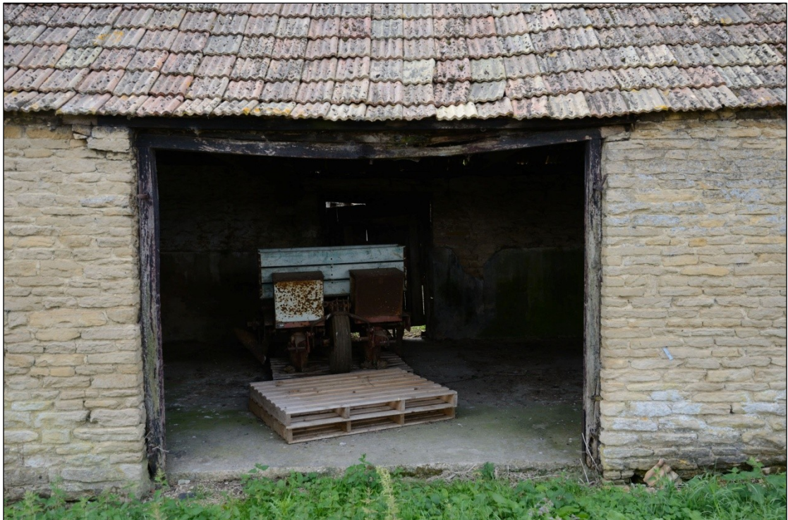
Plate 57: North door to Building 2, looking south-southeast
