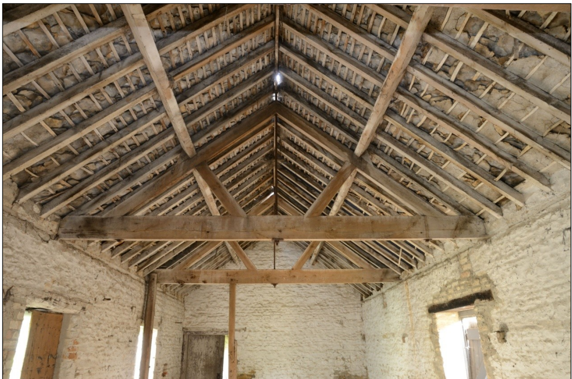
Plate 43: Roof structure inside Building 5C, looking south-southeast
