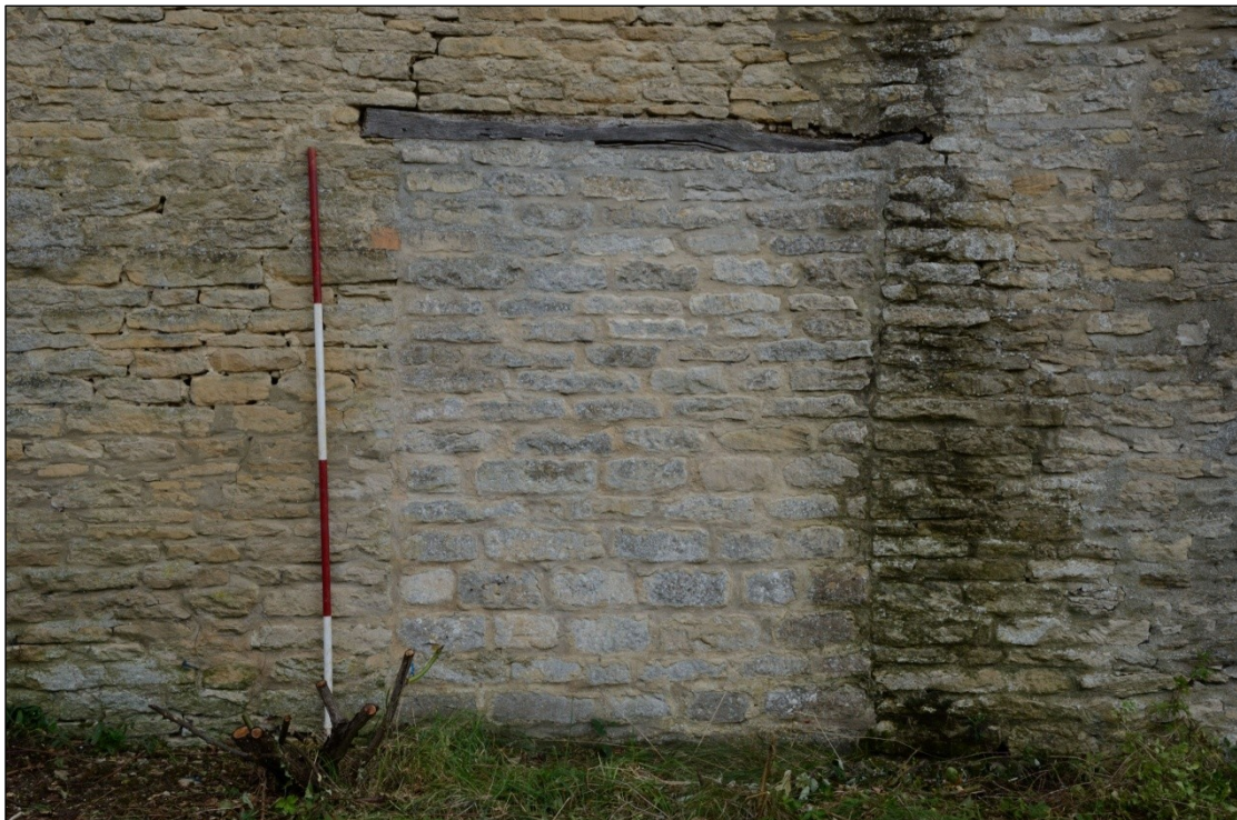
Plate 67: Blocked doorway in the south wall of Building 1, looking north-northwest
