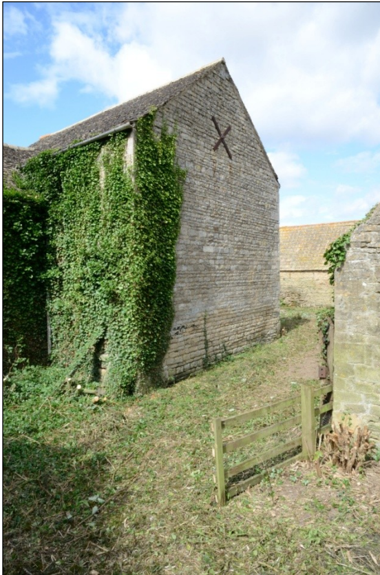
Plate 16: East facing elevation of Building 5A, looking northwest
