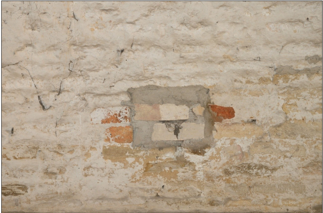
Plate 42: Recess in the east wall of Building 5C, looking east-northeast
