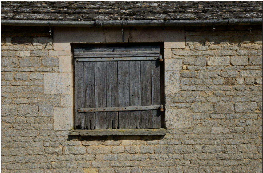
Plate 4: Pitching door in the west wall of Building 5C, looking east-northeast
