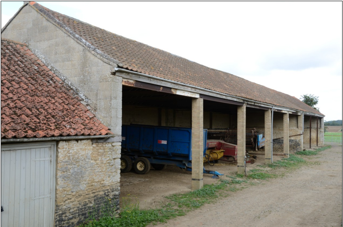
Plate 93: East elevation of Building 6 (A and B), looking northwest
