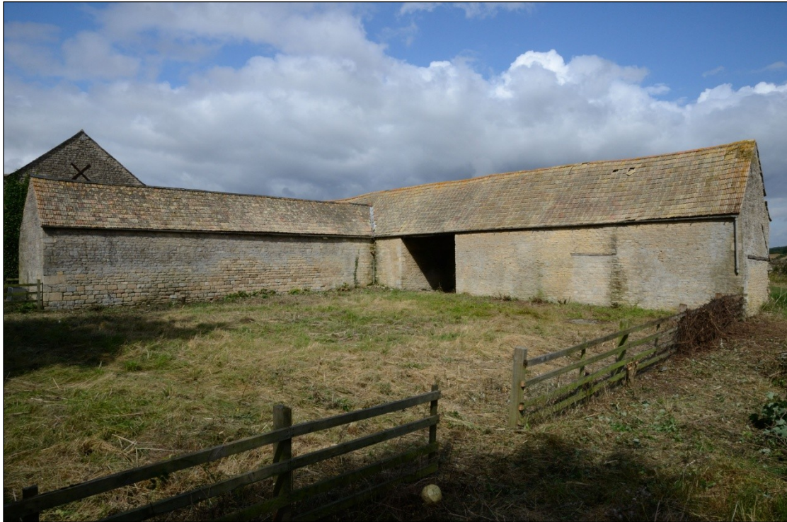
Plate 64: South elevation of Building 1 and east elevation of Building 2, looking west
