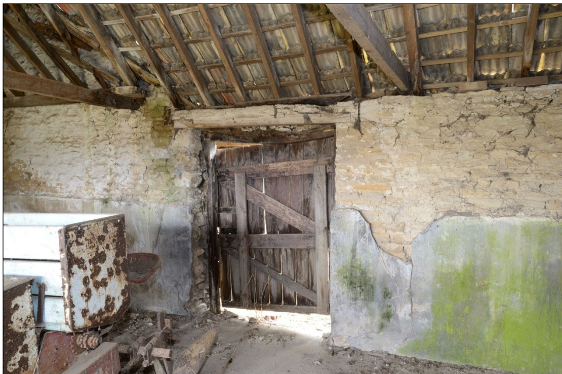
Plate 76: Door in the south wall of Building 2, looking southeast
