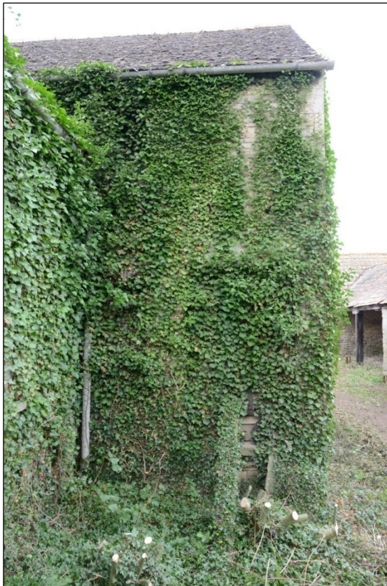
Plate 15: South facing elevation of Building 5A, looking north-northwest
