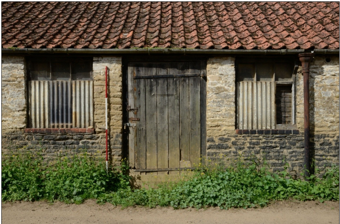
Plate 91: Door and windows to Building 6D, looking west-southwest (2m scale)
