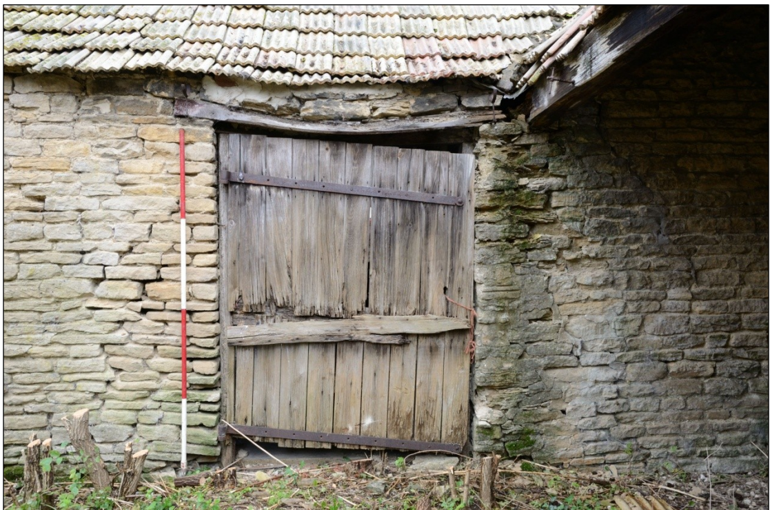
Plate 61: Door in the south wall of Building 2, looking north-northeast (2m scale)
