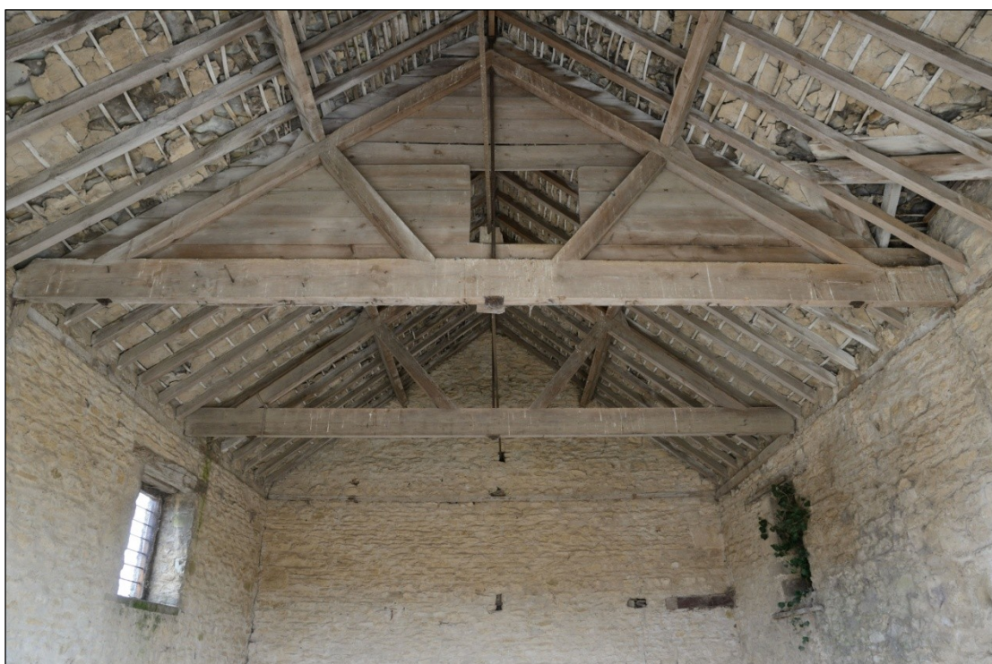
Plate 21: Roof structure in Building 5A, looking east-northeast
