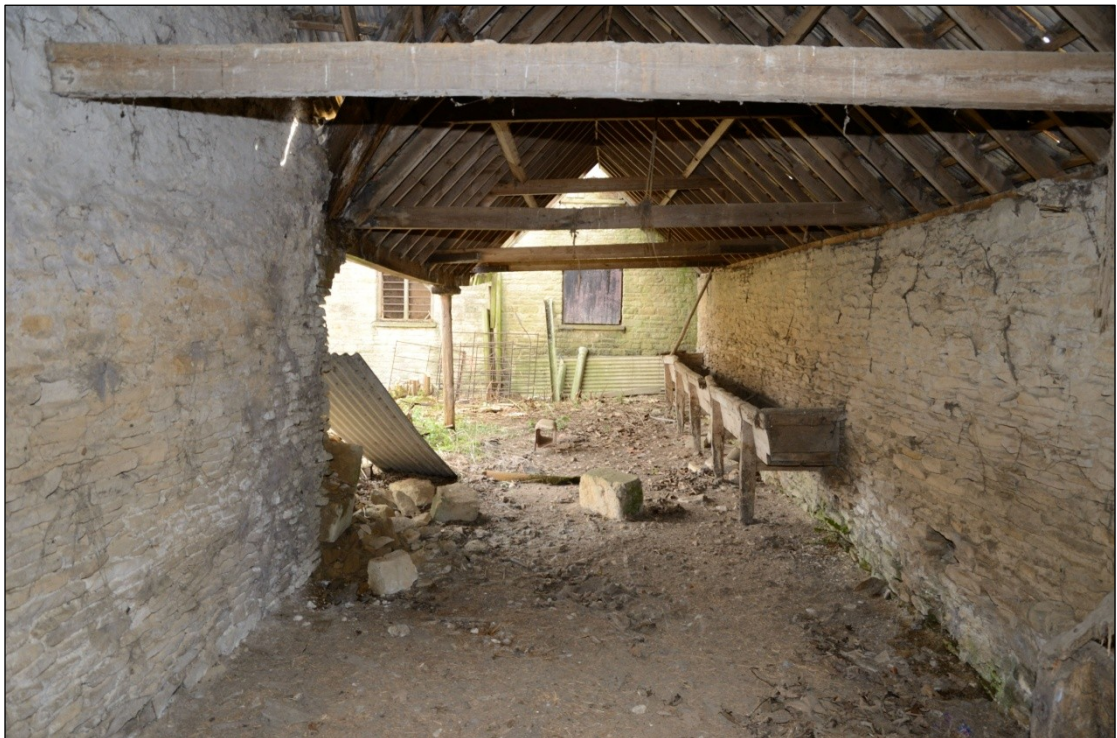
Plate 78: Interior of Building 4, looking south-southeast
