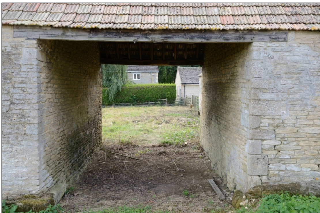
Plate 54: Covered entrance between Buildings 1 and 2, looking south-southeast
