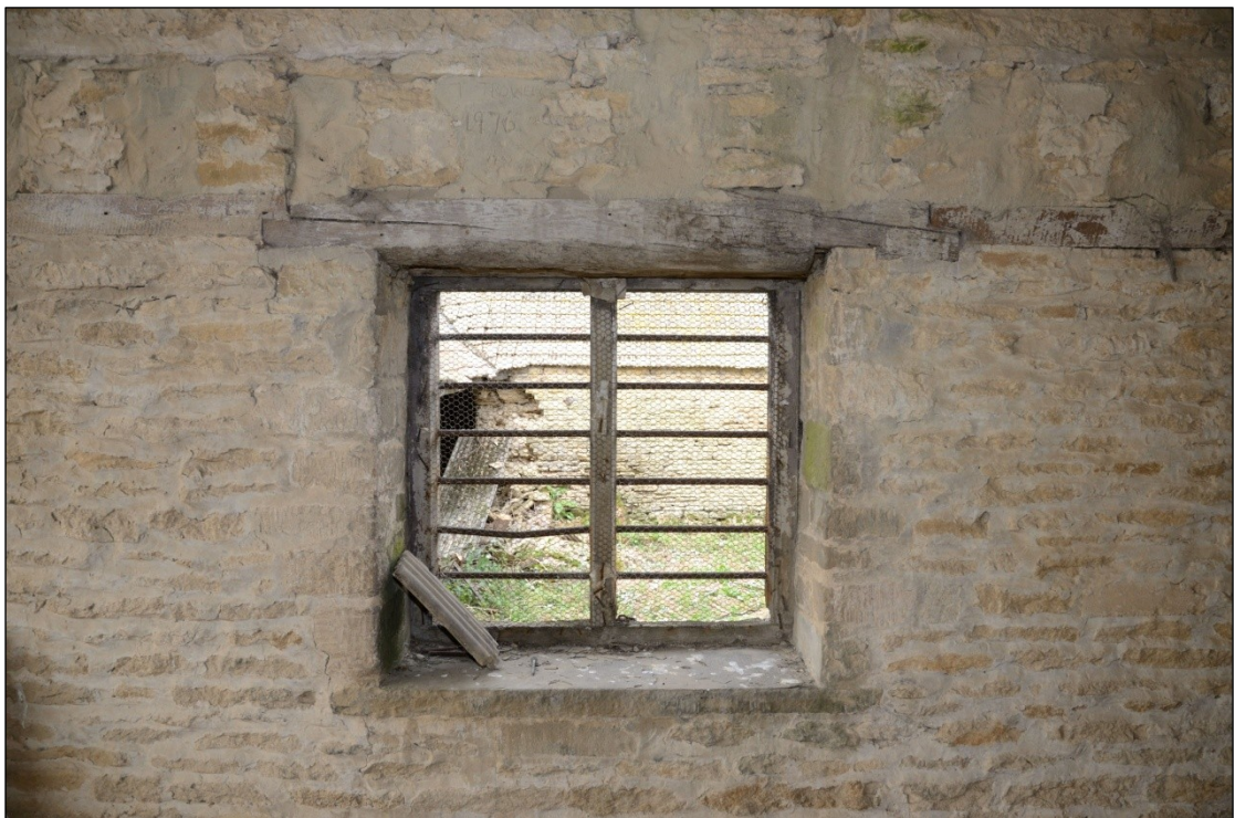
Plate 23: Window in the north wall of Building 5A, look north-northwest
