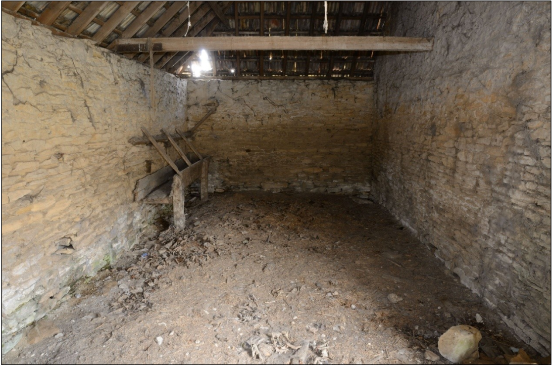
Plate 79: Interior of Building 4 (north end), looking north-northwest
