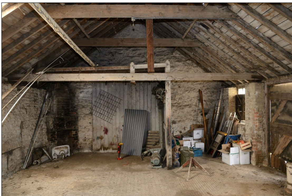
Plate 101: Interior of Building 6D, looking north-northwest
