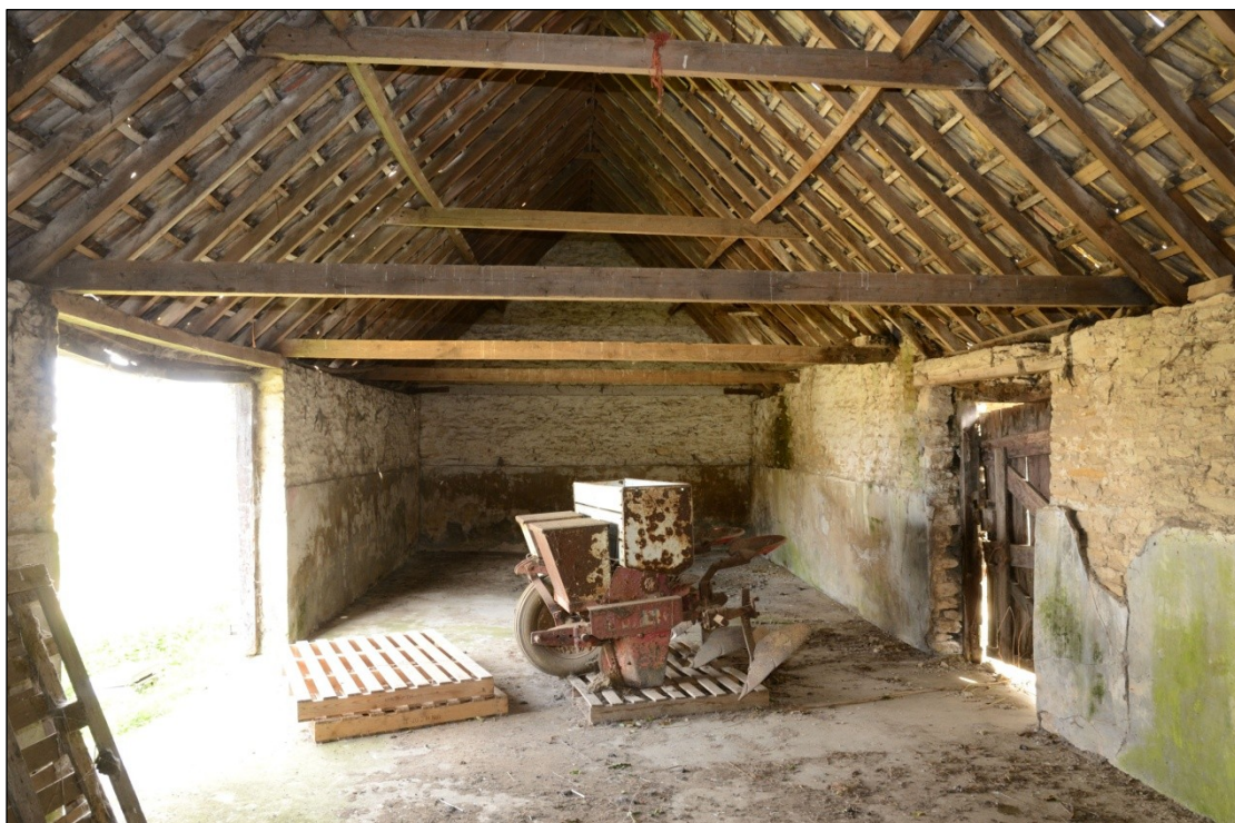
Plate 75: Interior of Building 2, looking east-northeast
