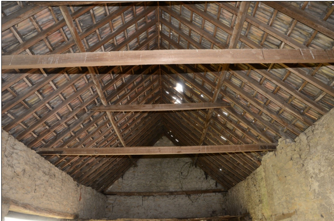
Plate 73: Roof structure in Building 1, looking east-northeast
