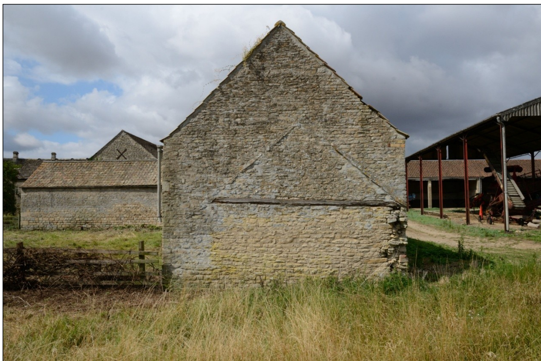
Plate 68: East elevation of Building 1, looking west-southwest
