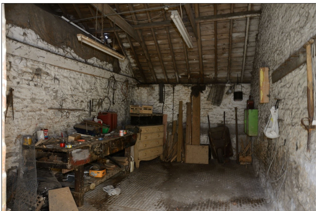
Plate 99: Interior of Building 6E, looking west-southwest
