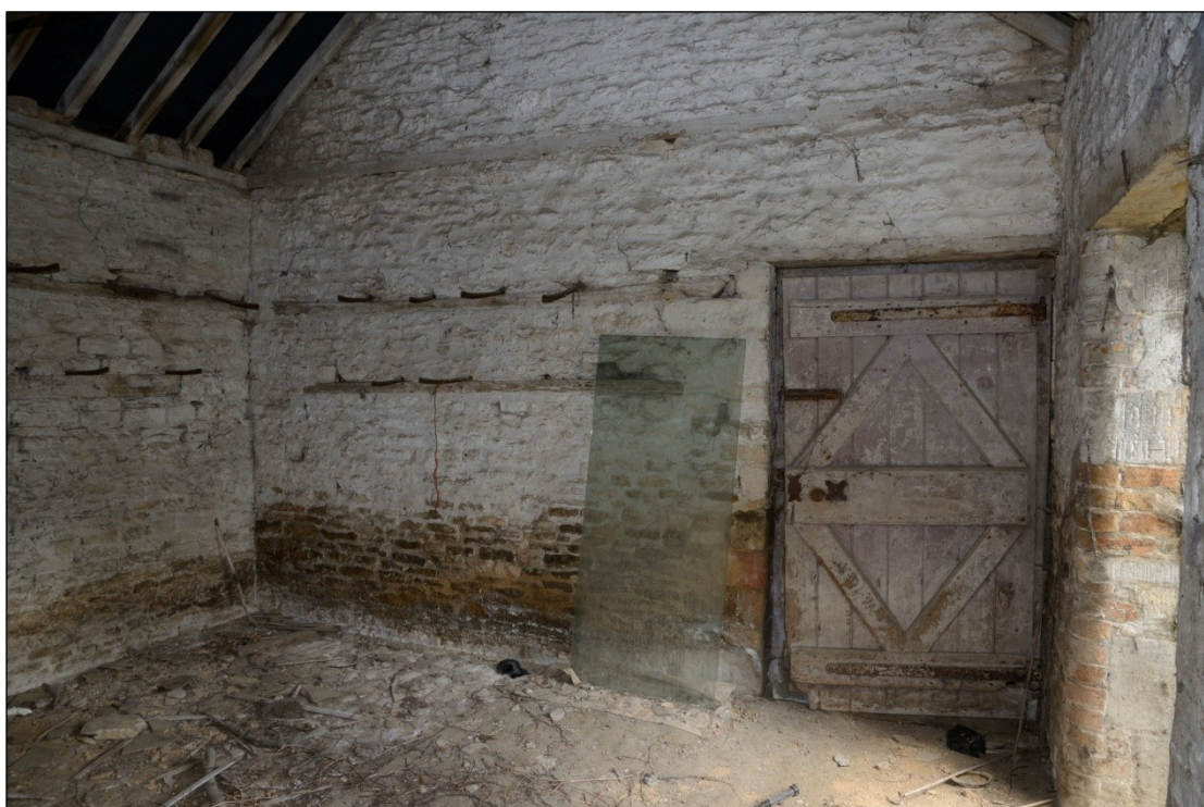
Plate 45: Interior of Building 5C, looking north-northwest
