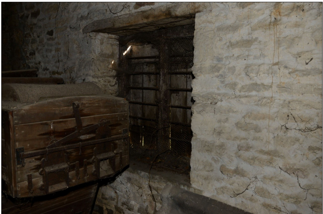
Plate 33: Window in the east wall of Building 5B, looking north-northeast
