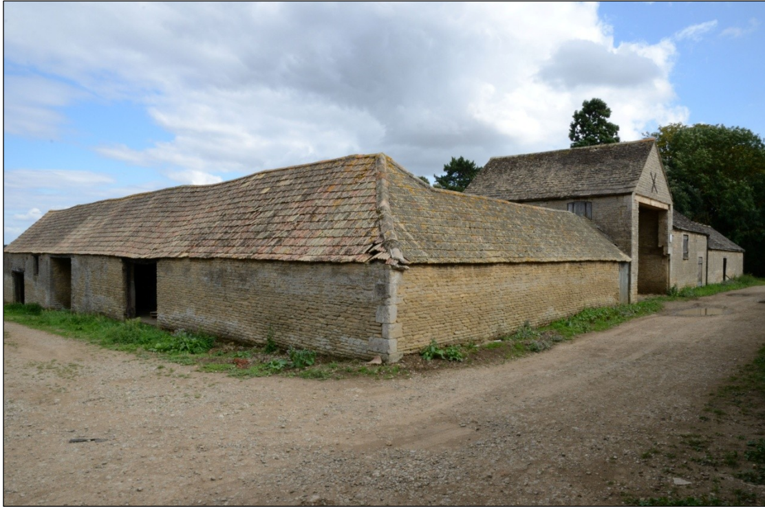
Plate 1: Buildings east side of the access track; north and west facing elevations, looking southeast
