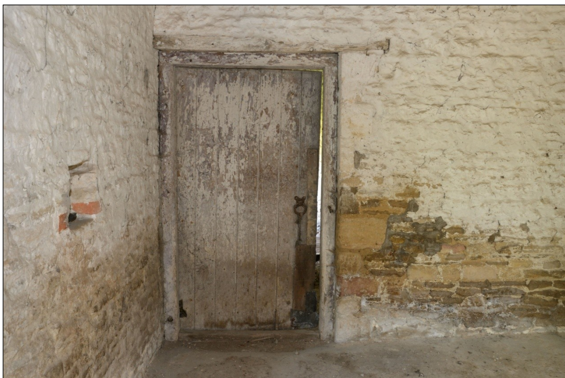
Plate 40: Door in the south wall of Building 5B, looking south-southeast
