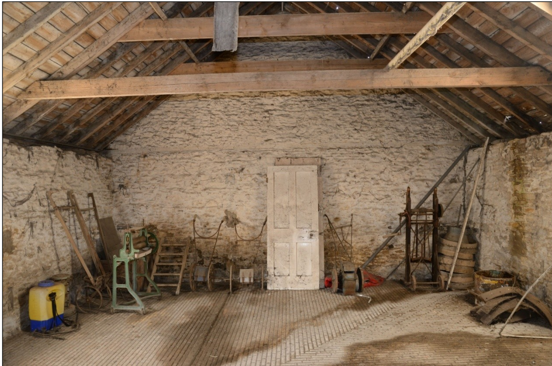
Plate 104: Interior of Building 6D, looking south-southeast
