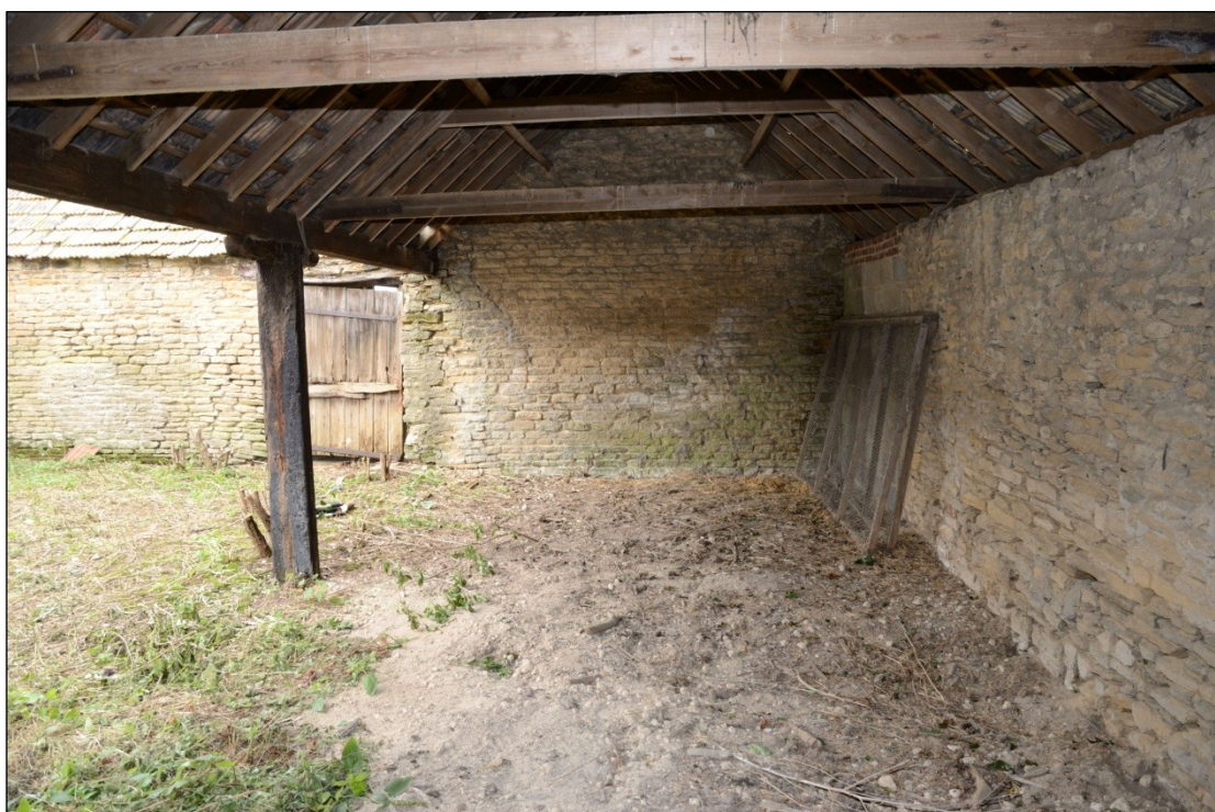
Plate 85: Interior of Building 3A, looking north-northwest
