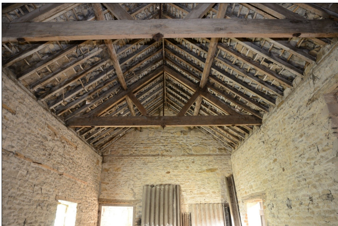
Plate 34: Roof structure in Building 5B, looking south-southeast
