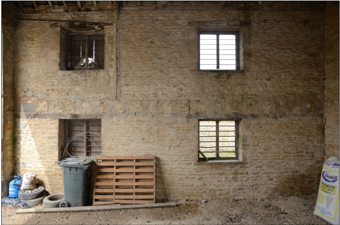
Plate 22: Interior of the north wall in Building 5A, looking north-northwest
