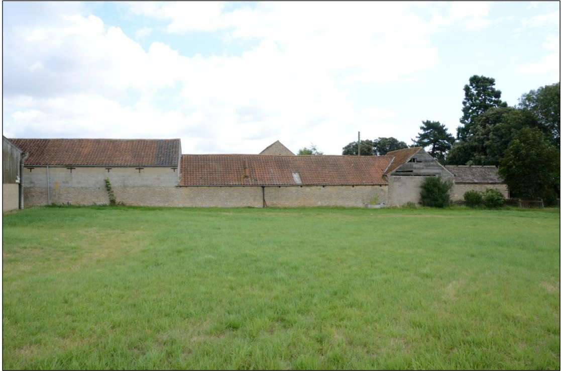
Plate 96: West elevation of Buildings 6 (obscured at northern end) and 7, looking east-northeast
