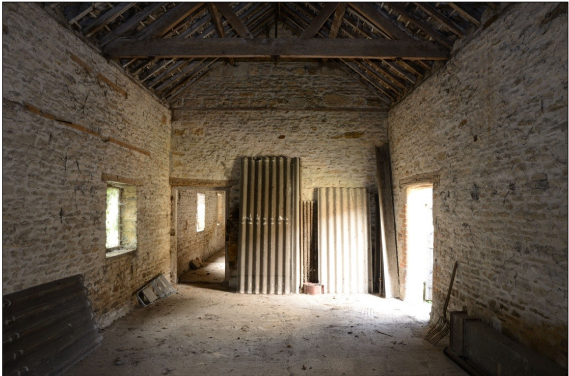
Plate 27: Southern end of Building 5B, looking south-southeast
