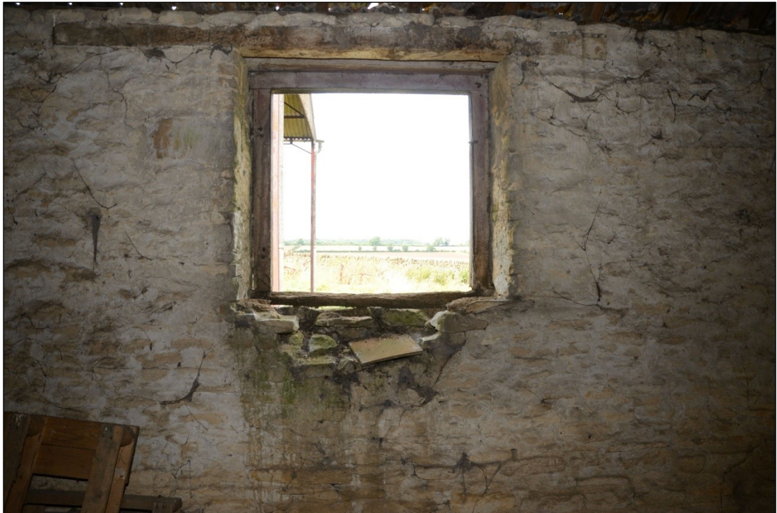
Plate 72: Pitching door in the north wall of Building 1, looking north-northwest
