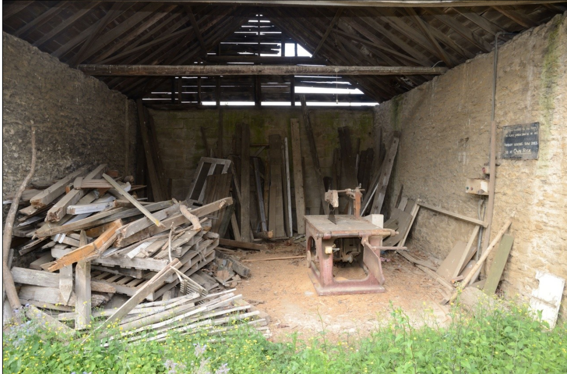
Plate 112: Interior of Building 7, looking west-southwest
