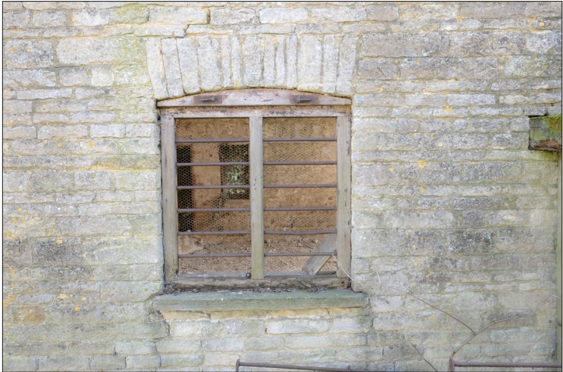
Plate 18: Window in the north facing elevation of Building 5A, looking south-southeast
