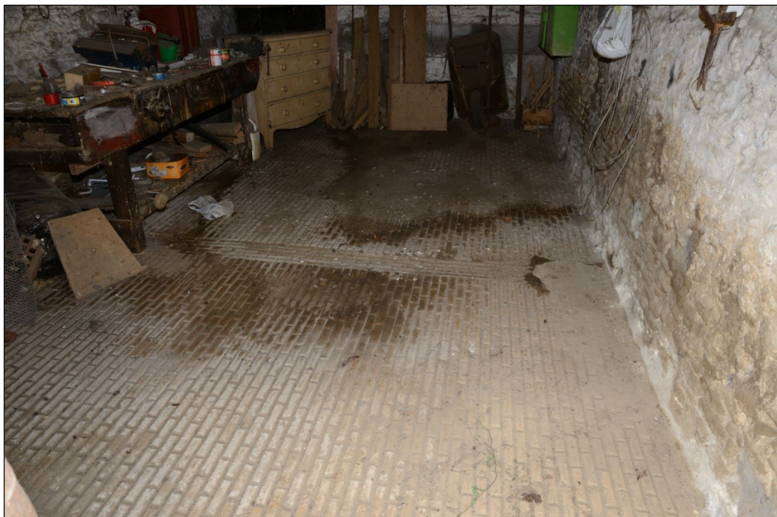
Plate 100: Floor in Building 6E, looking west-southwest
