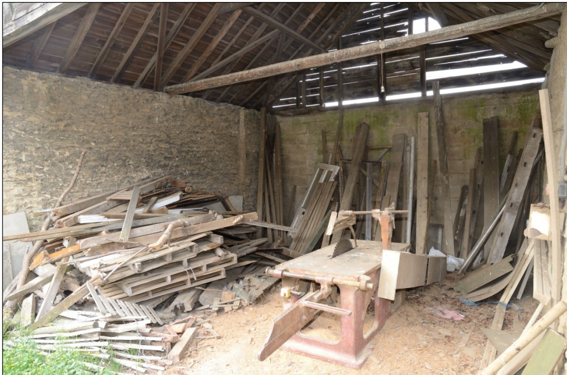
Plate 113: Interior of Building 7, looking southwest
