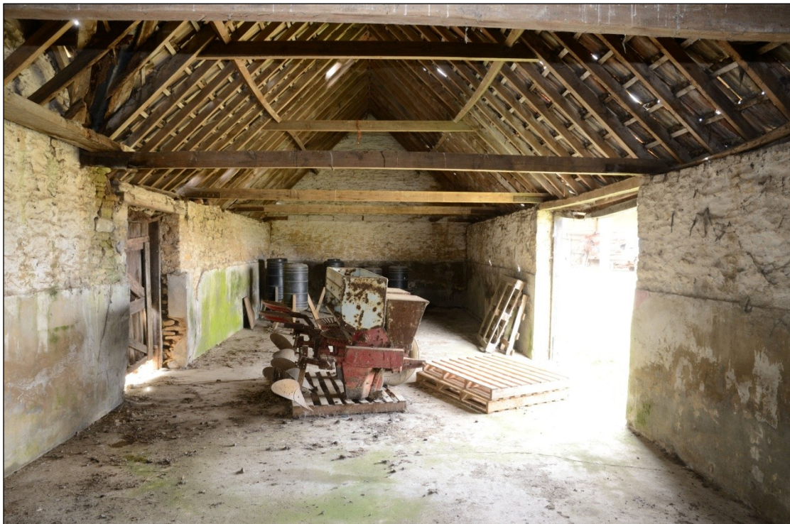
Plate 74: Interior of Building 2, looking west-southwest
