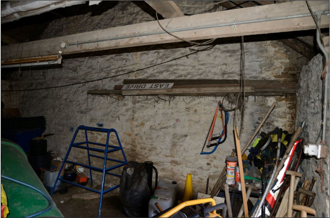
Plate 108: Interior of Building 6C, looking west-northwest
