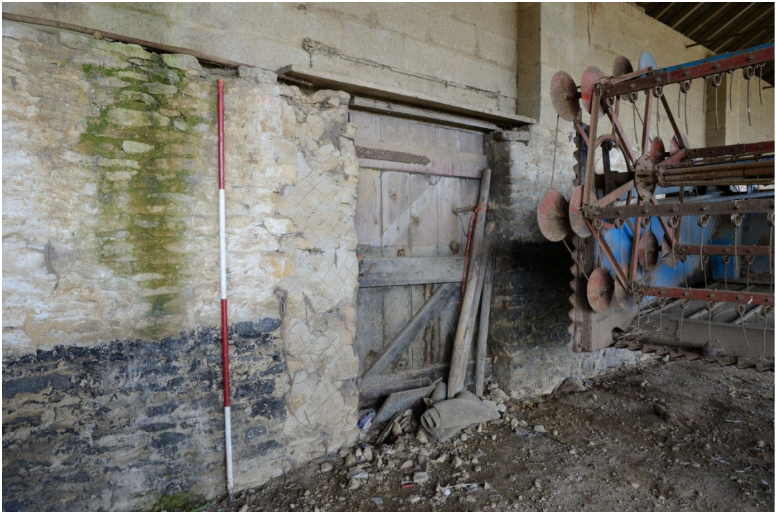
Plate 111: Door in the west wall of Building 6C, looking west-northwest
