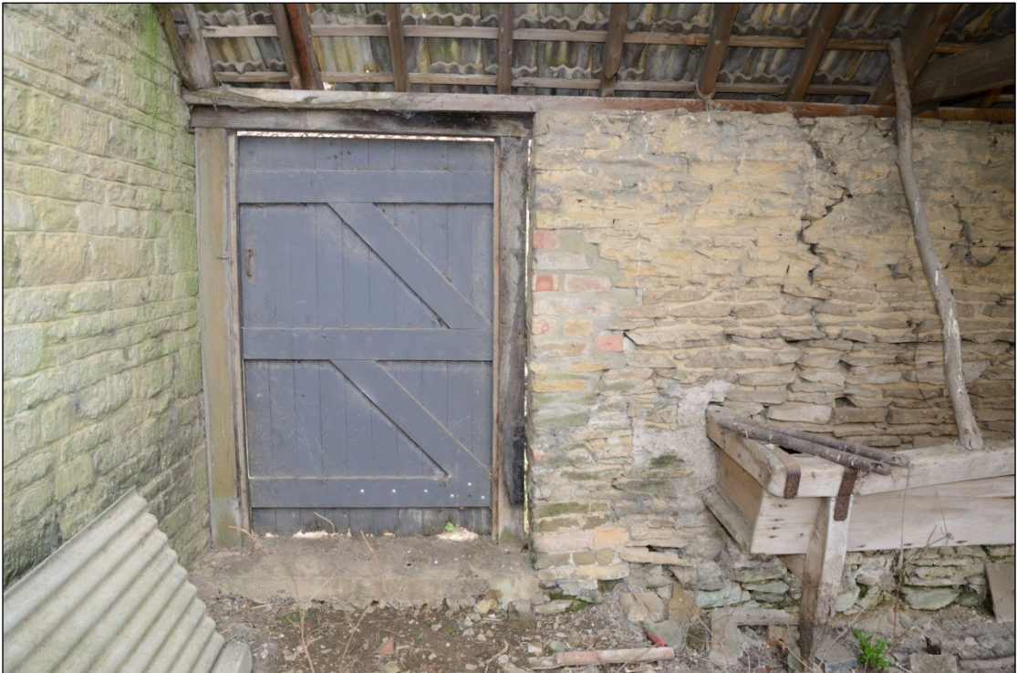
Plate 80: Door in the north wall of Building 4, looking west-southwest
