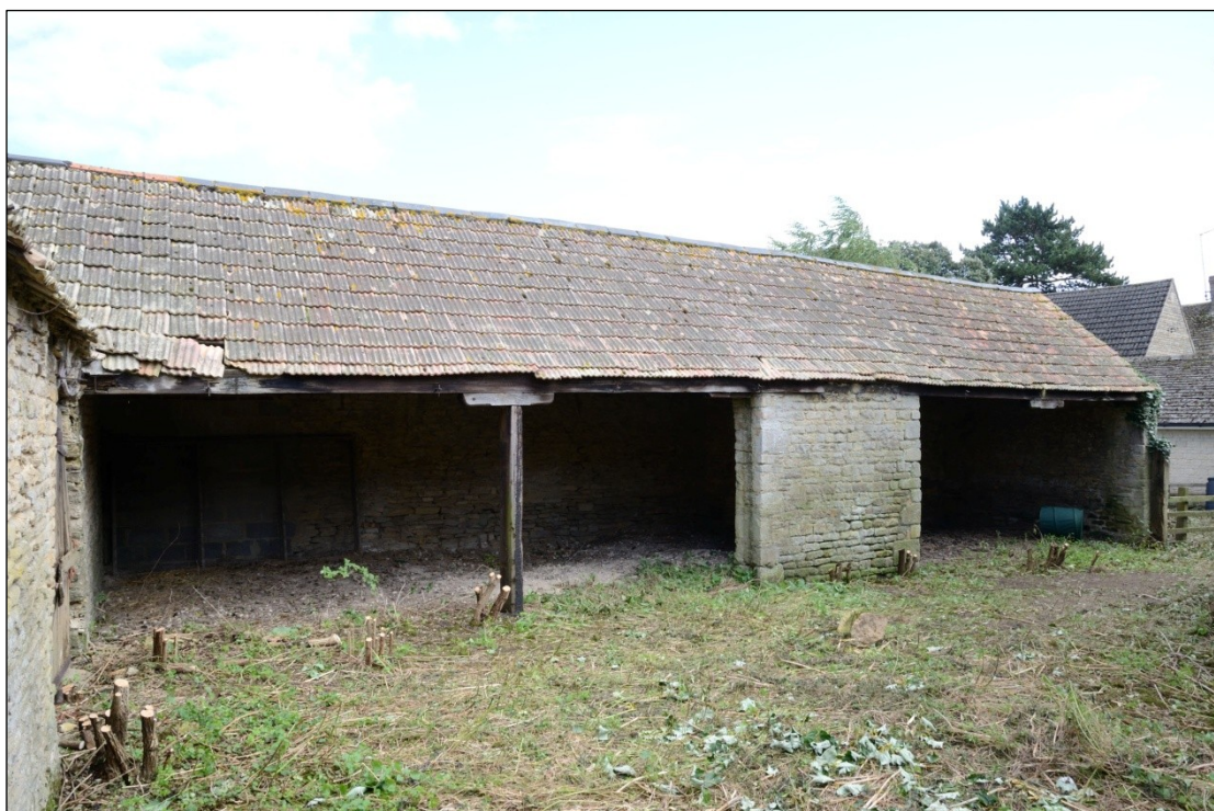
Plate 62: West elevation of Building 3, looking west-southwest
