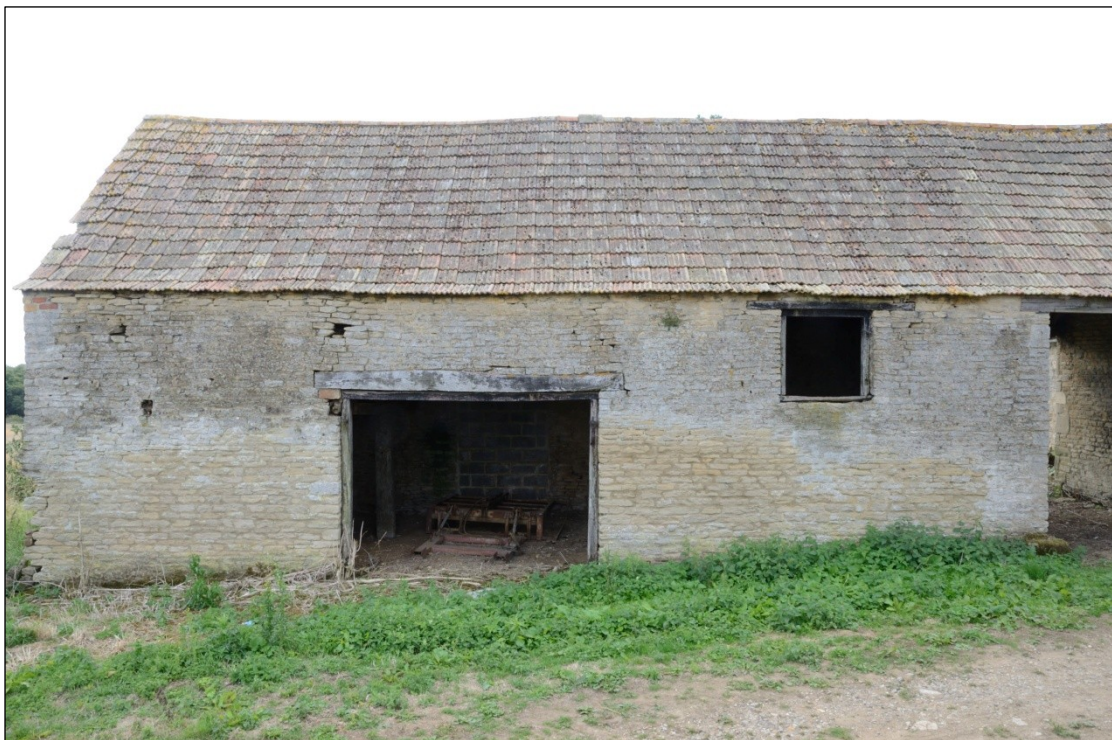
Plate 51: North elevation of Building 1, looking south-southeast
