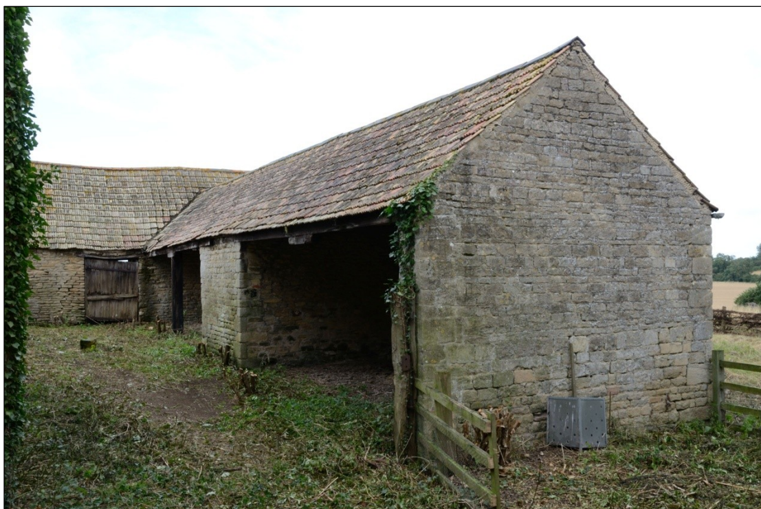
Plate 63: West and south elevations of Building 3, looking north
