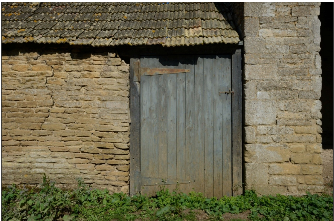
Plate 59: Door in the west wall of Building 4, looking east-northeast
