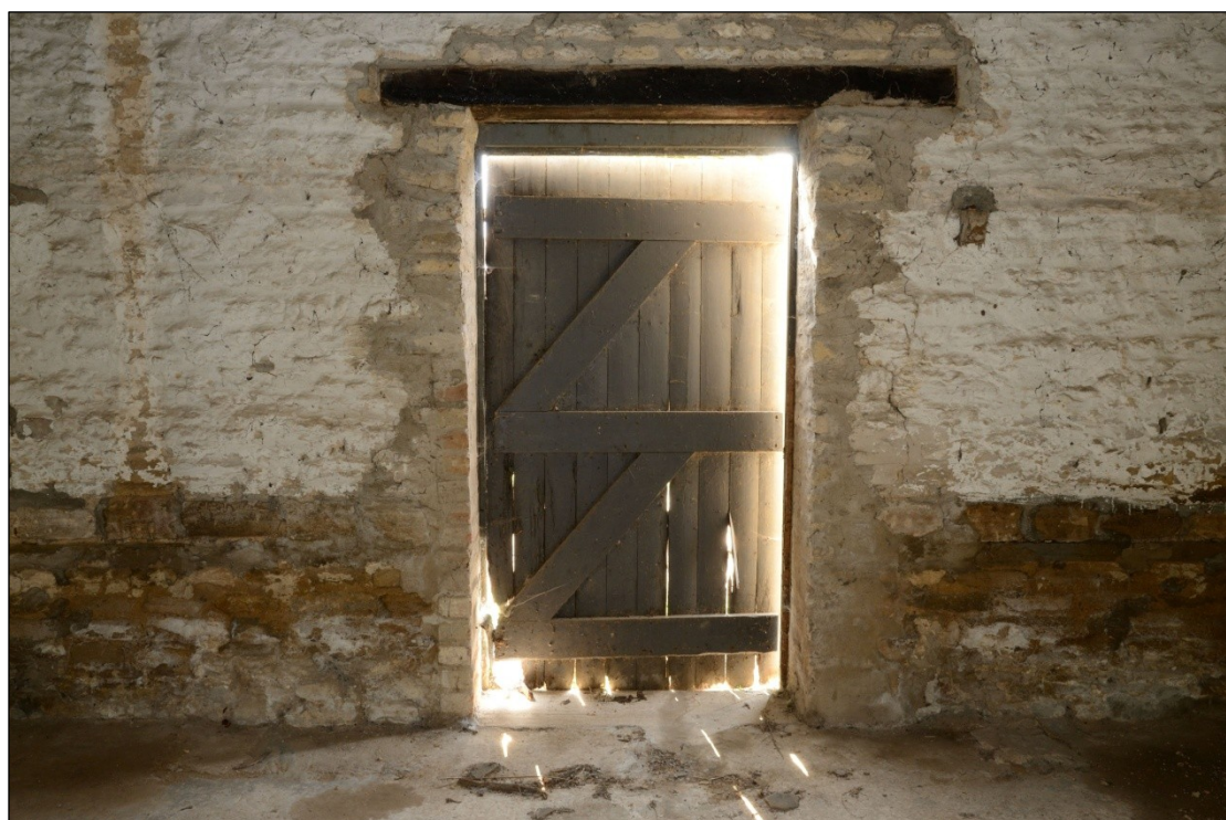
Plate 39: Door in the east wall of Building 5C, looking west-southwest
