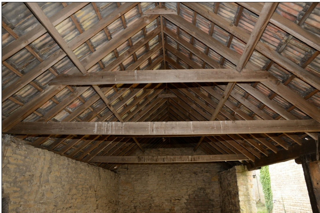
Plate 84: Roof structure in Building 3A, looking south-southeast
