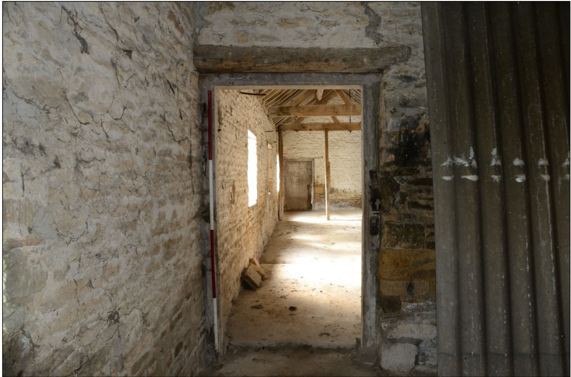
Plate 28: Door in the south wall of Building 5B, looking south-southeast
