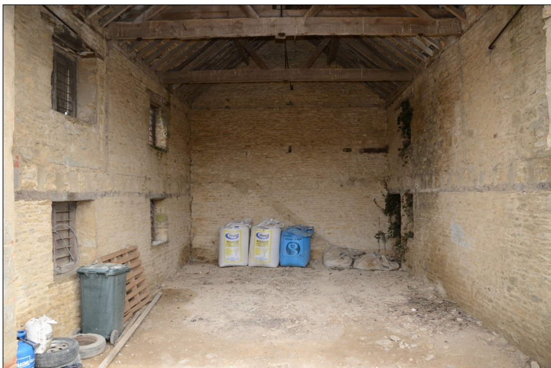
Plate 20: Interior of Building 5A, looking east-northeast
