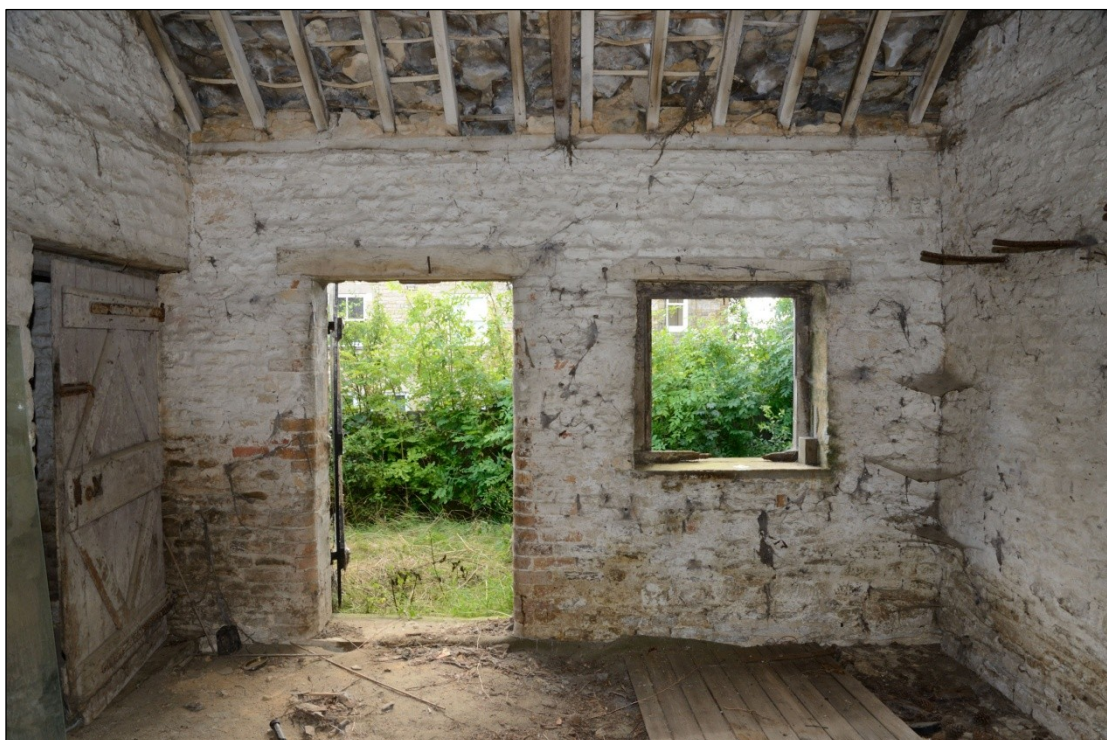
Plate 44: Interior of Building 5C, looking east-northeast
