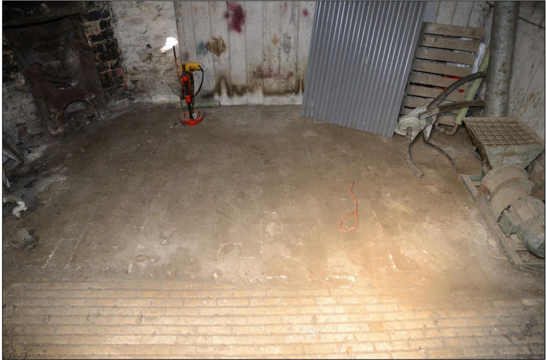
Plate 106: Floor on the north side of Building 6D, looking north-northwest
