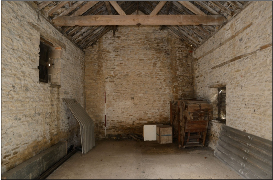
Plate 26: Northern end of Building 5A, looking north-northwest (2m scale)
