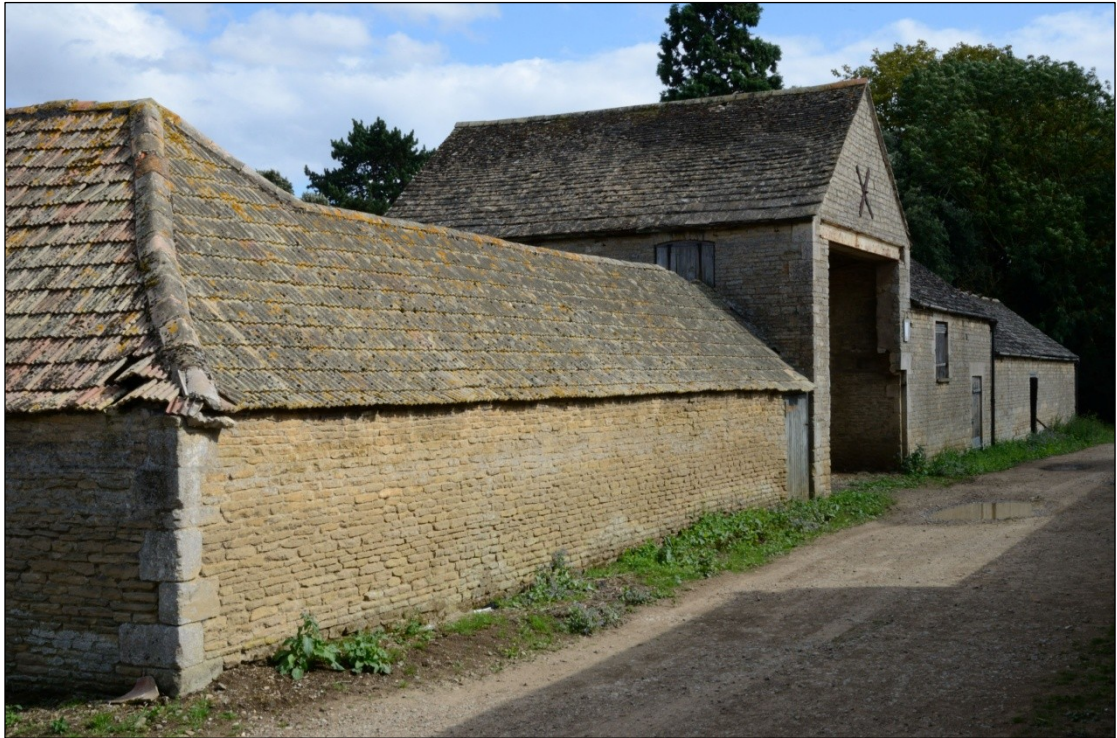
Plate 58: West elevation of Buildings 2 and 4 (also 5), facing southeast
