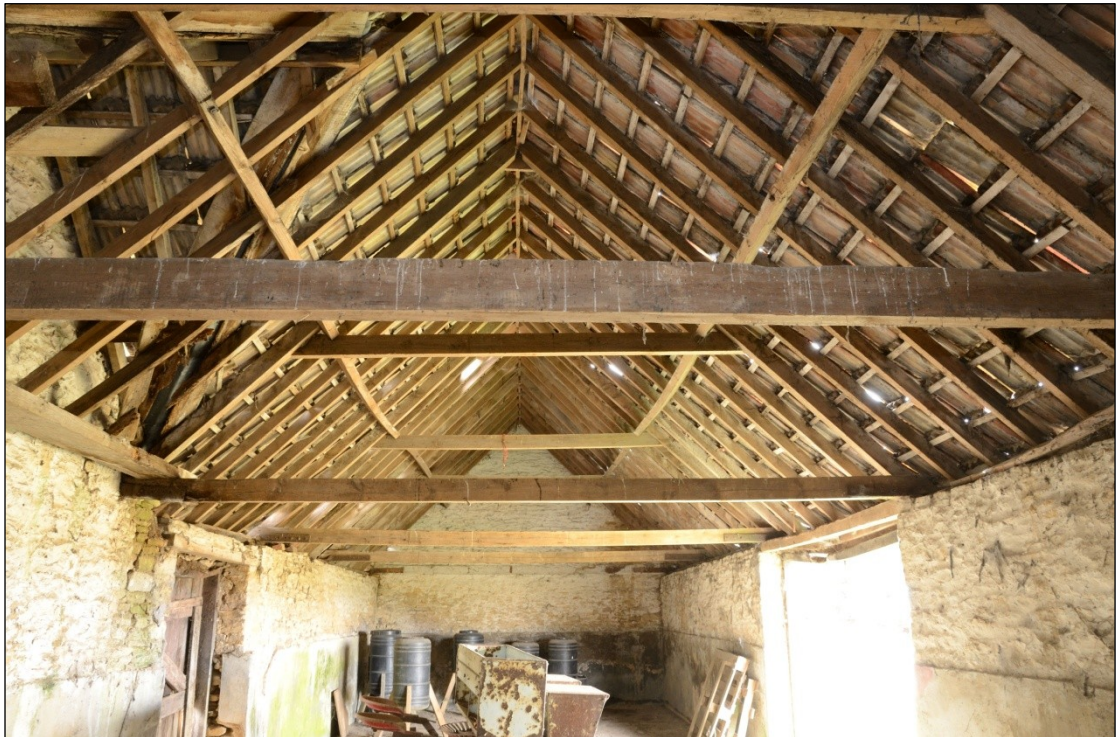
Plate 77: Roof structure in Building 2, looking west-southwest
