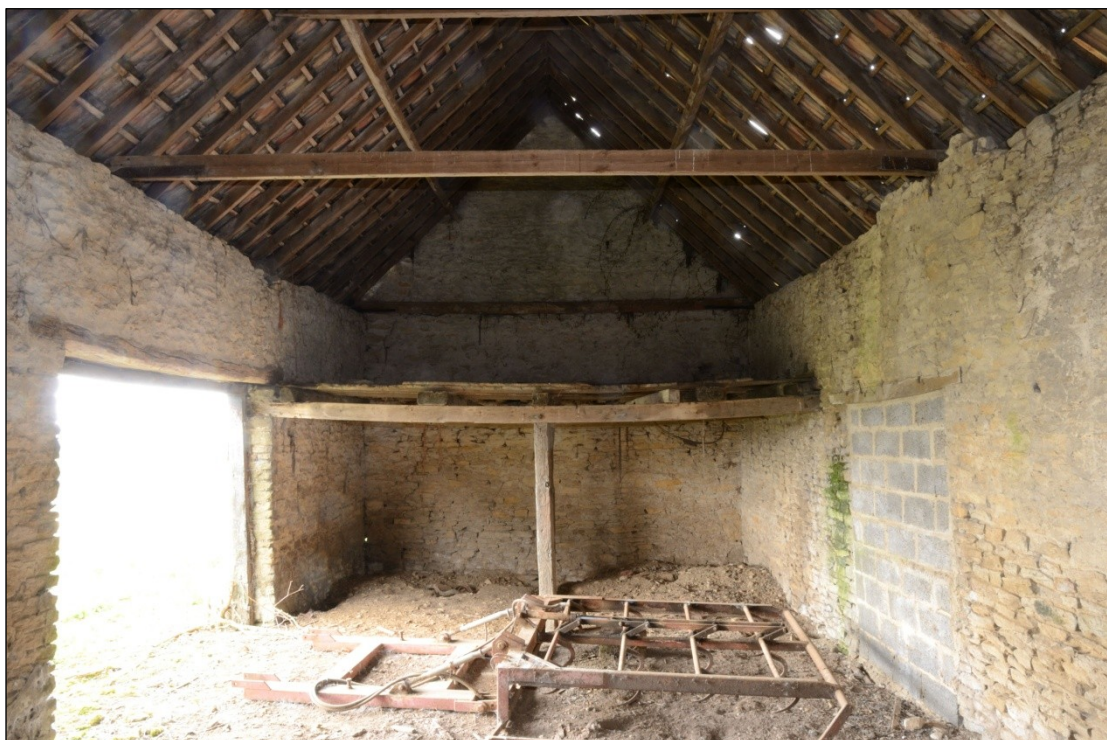
Plate 69: Interior of Building 1 – eastern end, looking east-northeast
