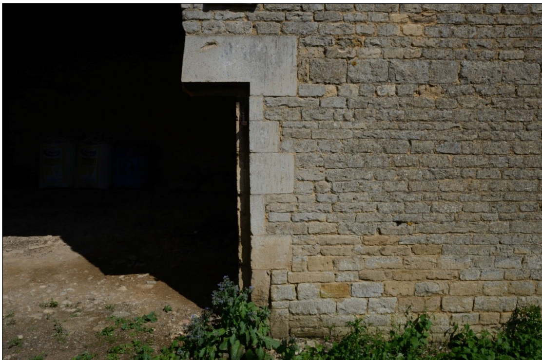
Plate 3: Surviving extent of door to Building 5B, looking east-northeast
