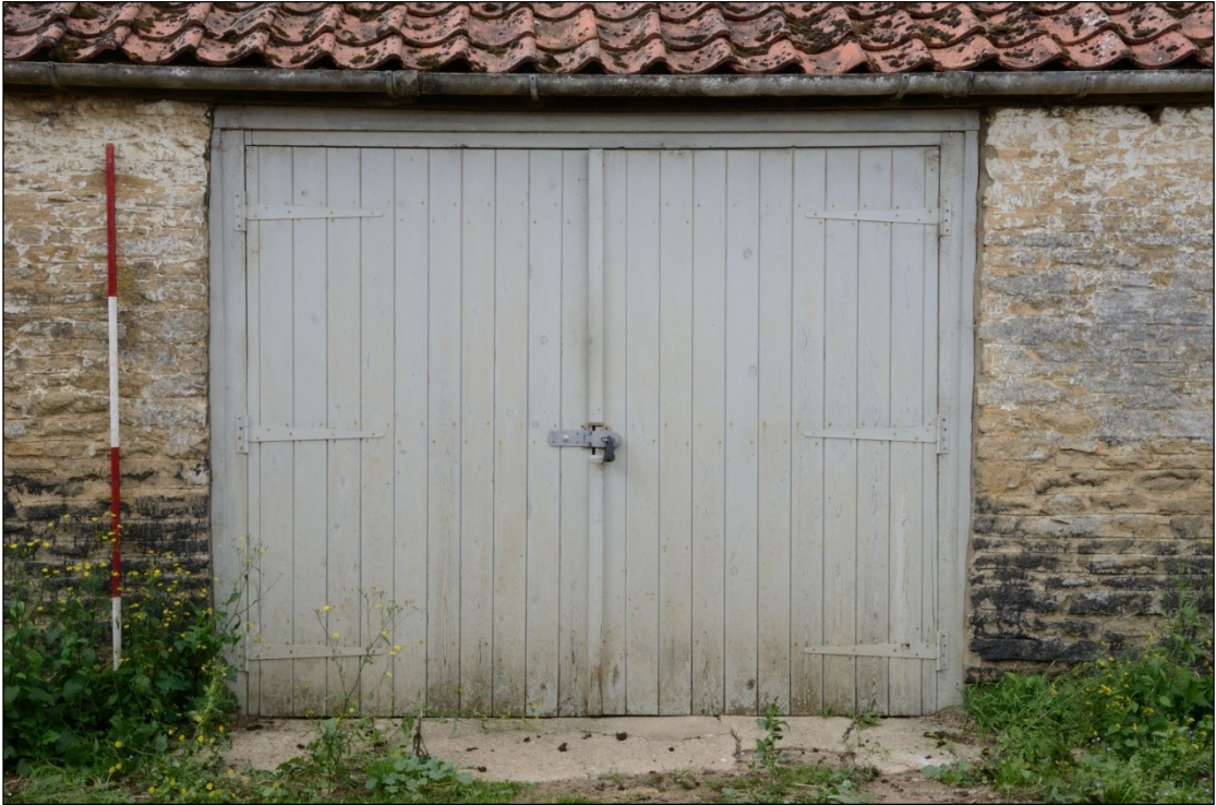
Plate 92: Door to Building 6C, looking west-southwest
