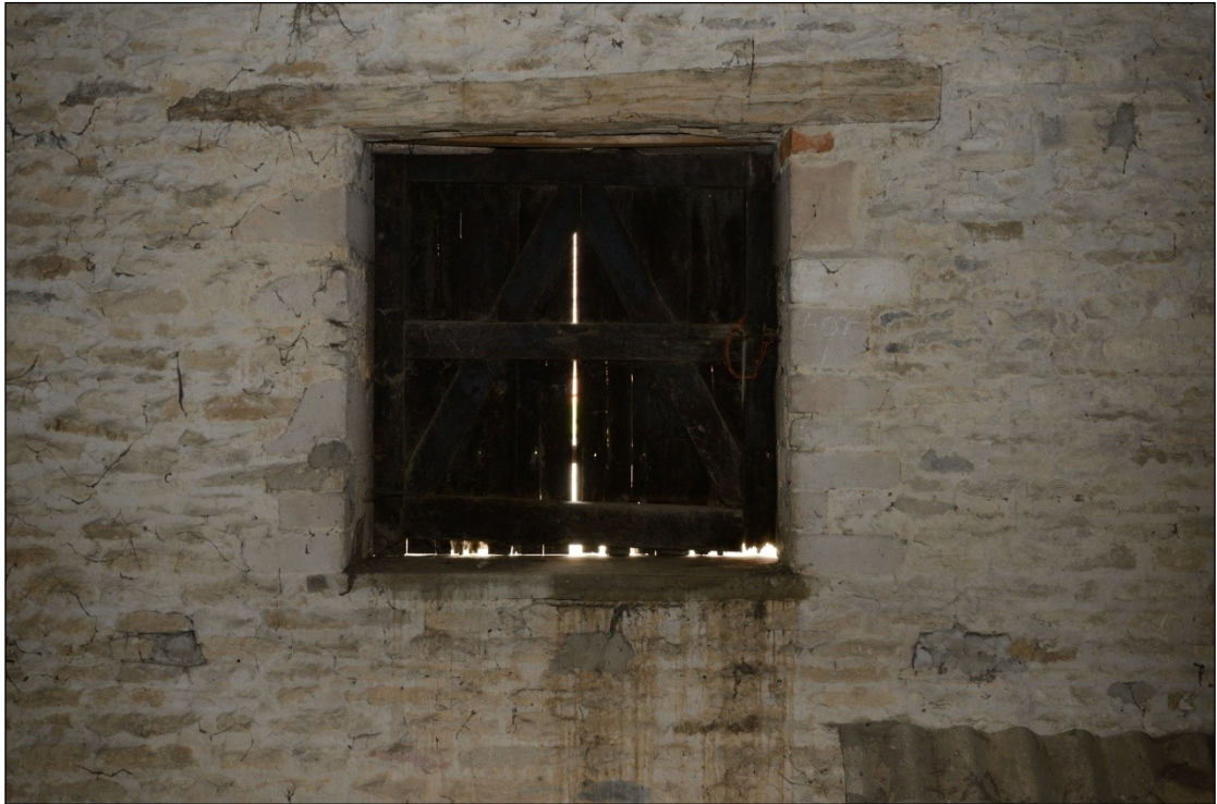
Plate 32: Pitching door in the west wall of Building 5B, looking west-southwest
