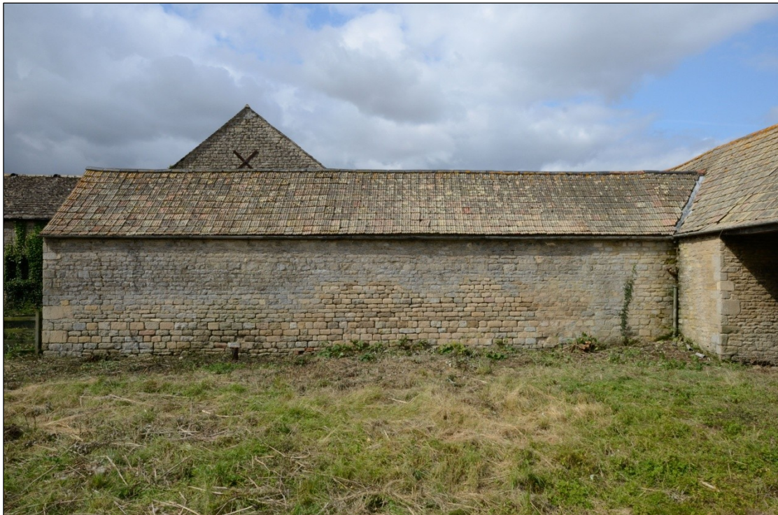
Plate 65: East elevation of Building 3, looking west-southwest
