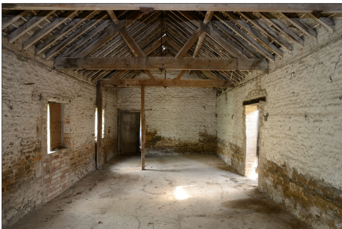
Plate 35: South end of Building 5C, looking south-southeast
