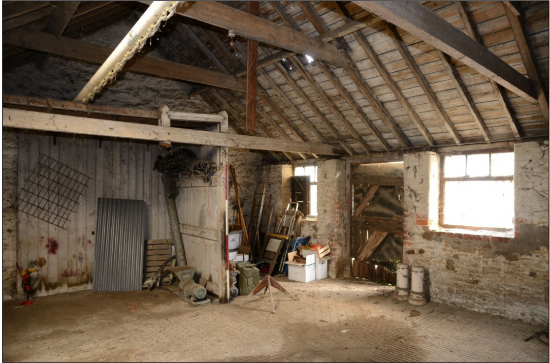
Plate 102: Interior of Building 6D, looking north (2m scale)
