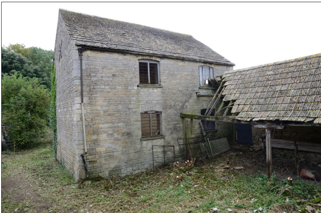
Plate 17: North facing elevation of Building 5A, looking south
