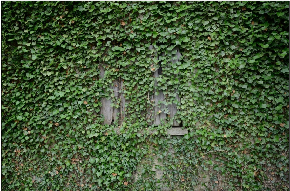
Plate 14: Window in the east wall of Building 5B, looking west-southwest
