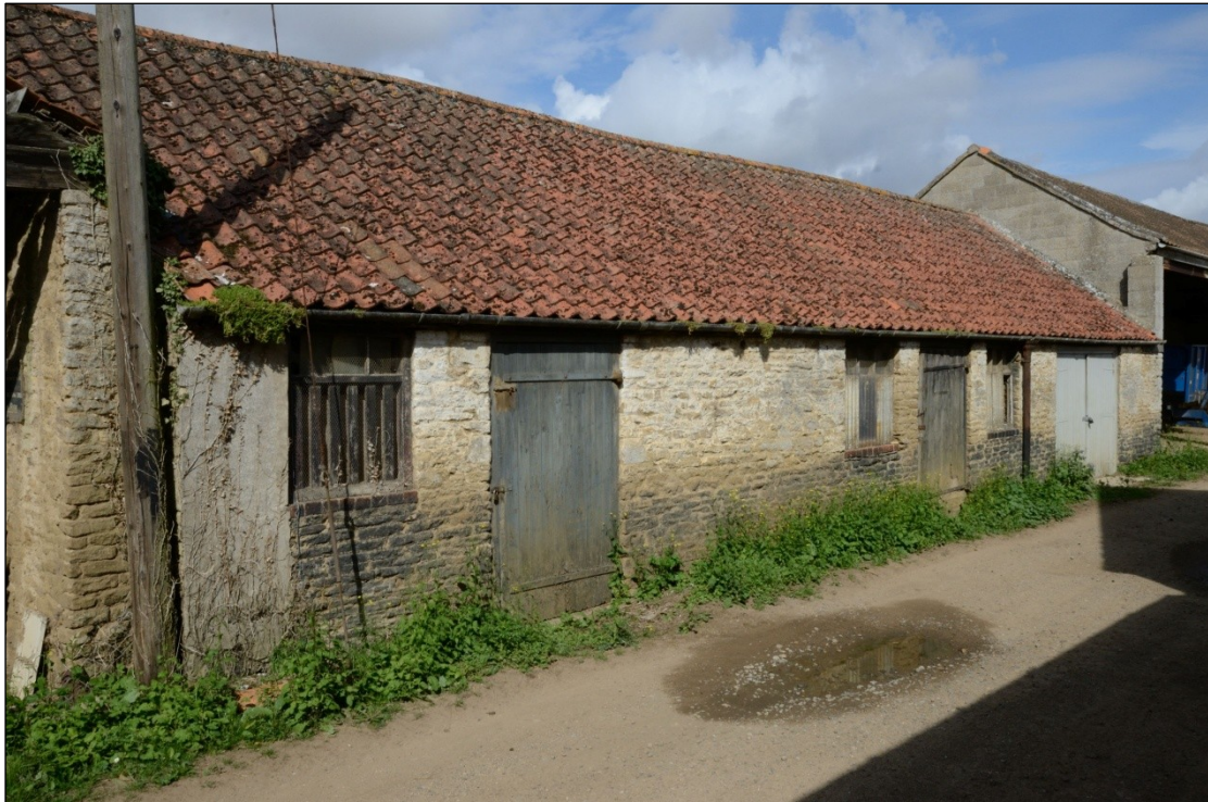
Plate 89: East elevation of Building 6 (C, D and E), looking west-northwest
