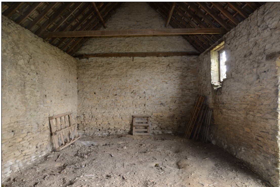
Plate 70: West side of Building 1, looking west-southwest
