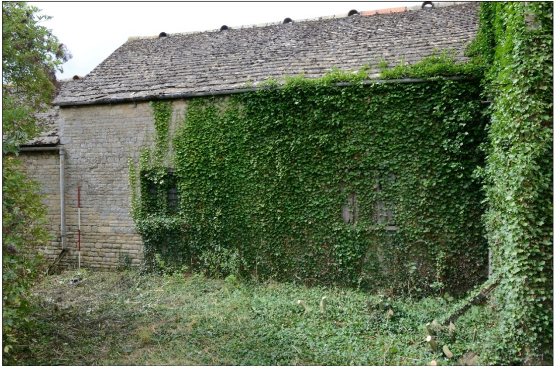
Plate 12: East side of Building 5B, looking southwest (2m scale)
