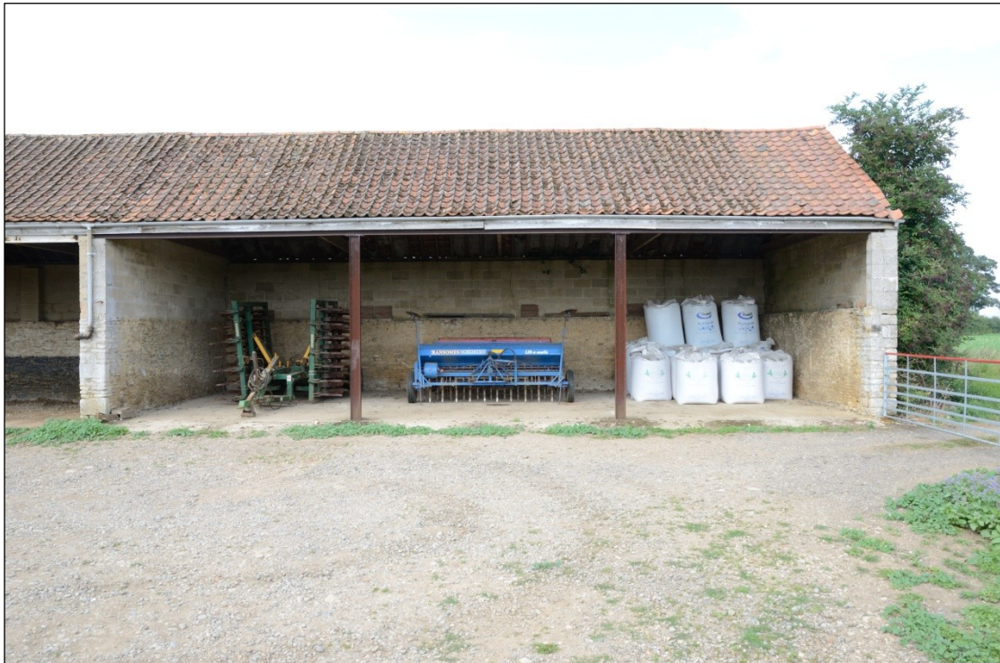
Plate 94: East elevation of Building 6A, looking west-southwest
