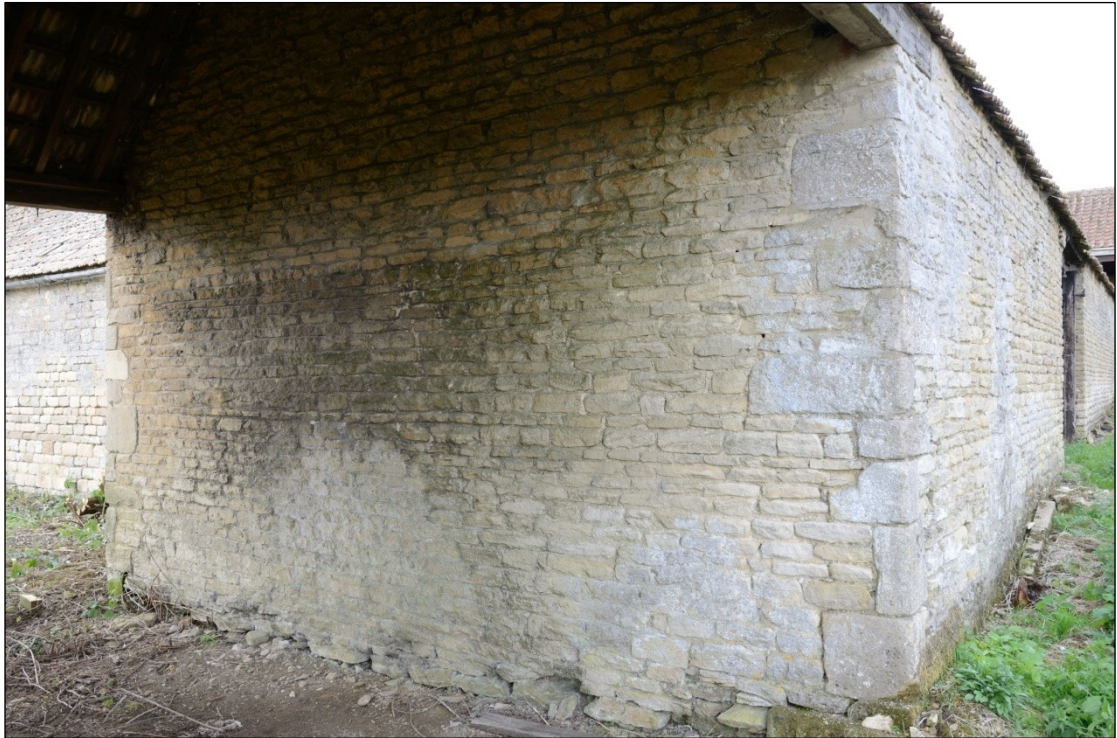
Plate 56: East elevation of Building 2, looking southwest
