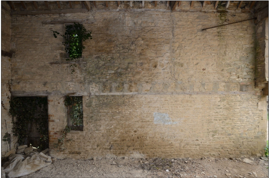
Plate 24: Interior of the south wall in Building 5A, looking south-southwest
