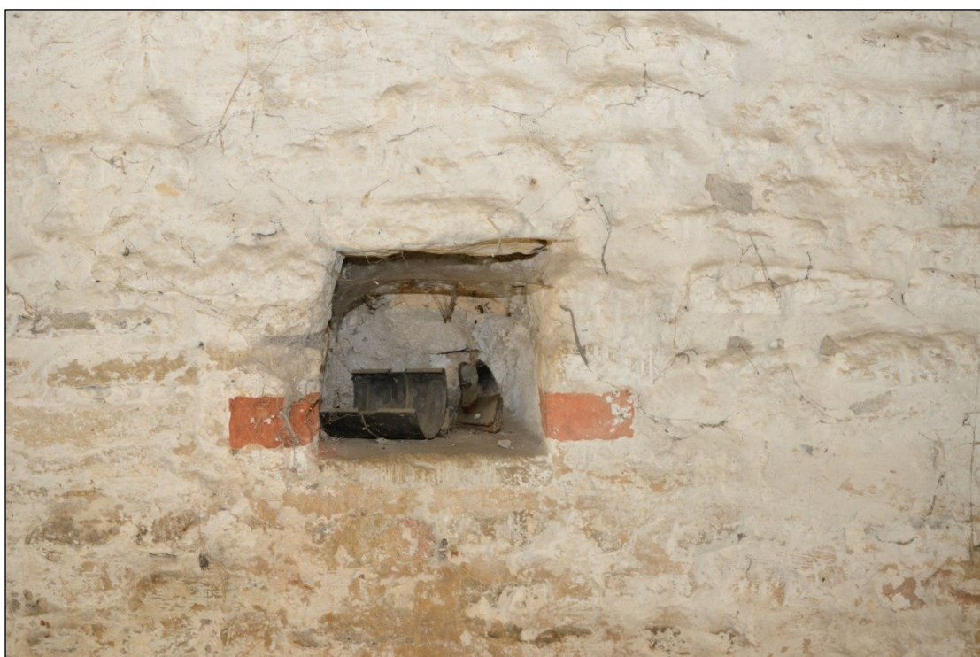
Plate 41: Recess in the east wall of Building 5C, looking east-northeast
