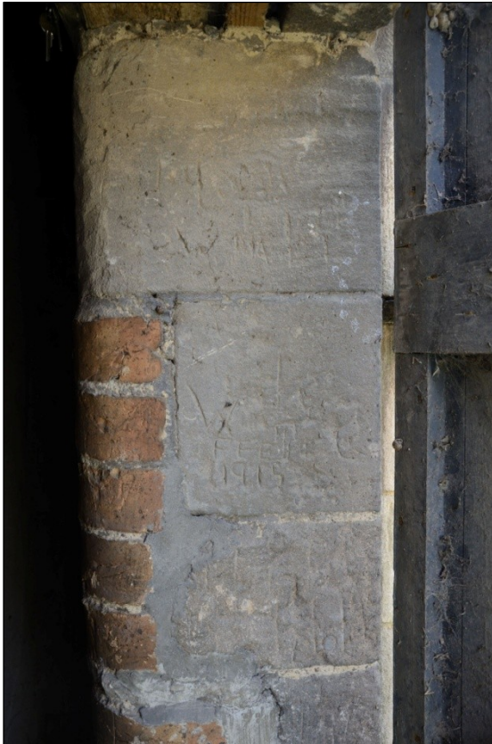
Plate 30: Graffiti on the south side of the door to Building 5B, looking south
