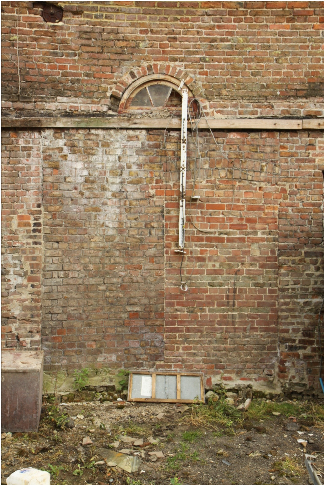
Plate 17: Bricked up doorways in the north elevation of Barn 1, looking south
