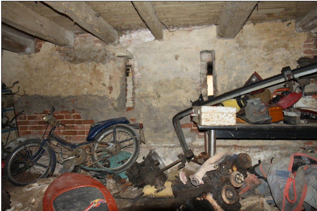
Plate 77: Interior view of ventilation slots in the south wall (east end) of Barn 2, looking south
