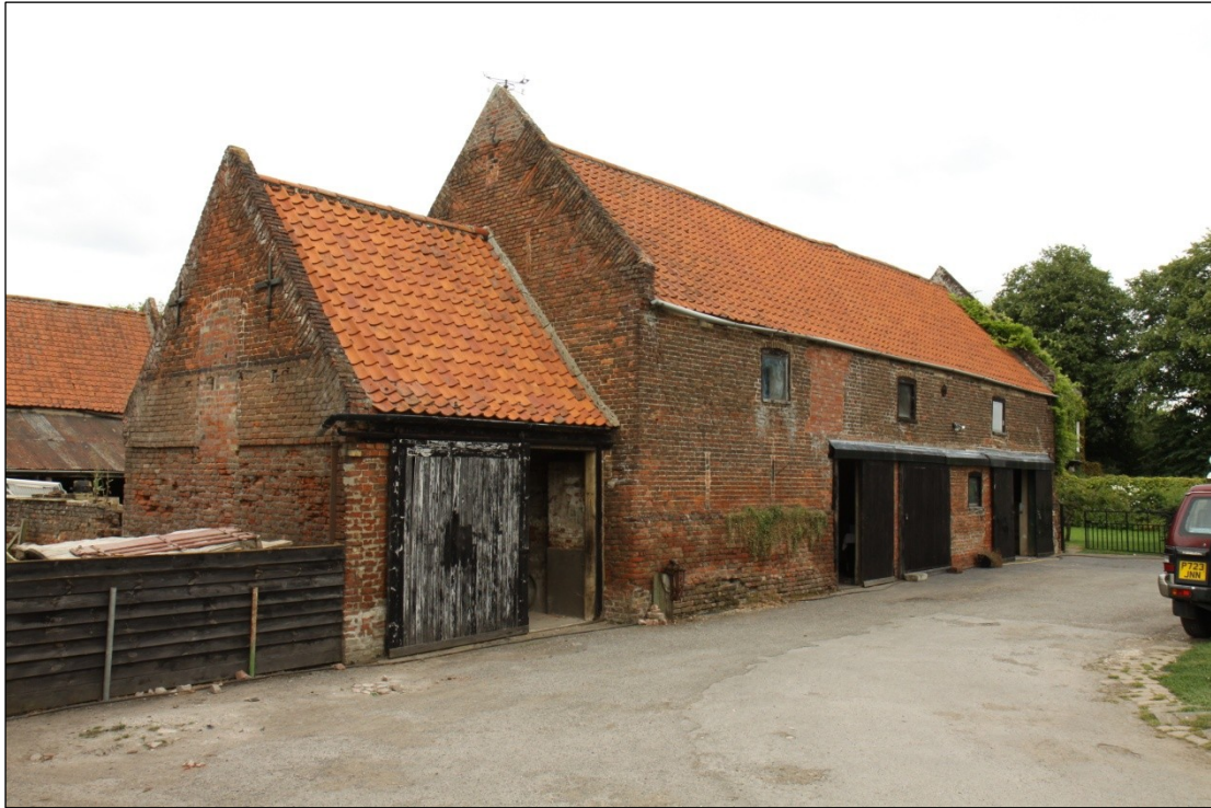
Plate 1: General view of Barn 1, looking northeast
