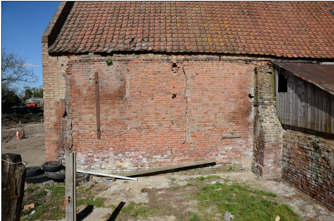
Plate 51: South facing elevation of Barn 2 (lean-to removed), west side, looking north
