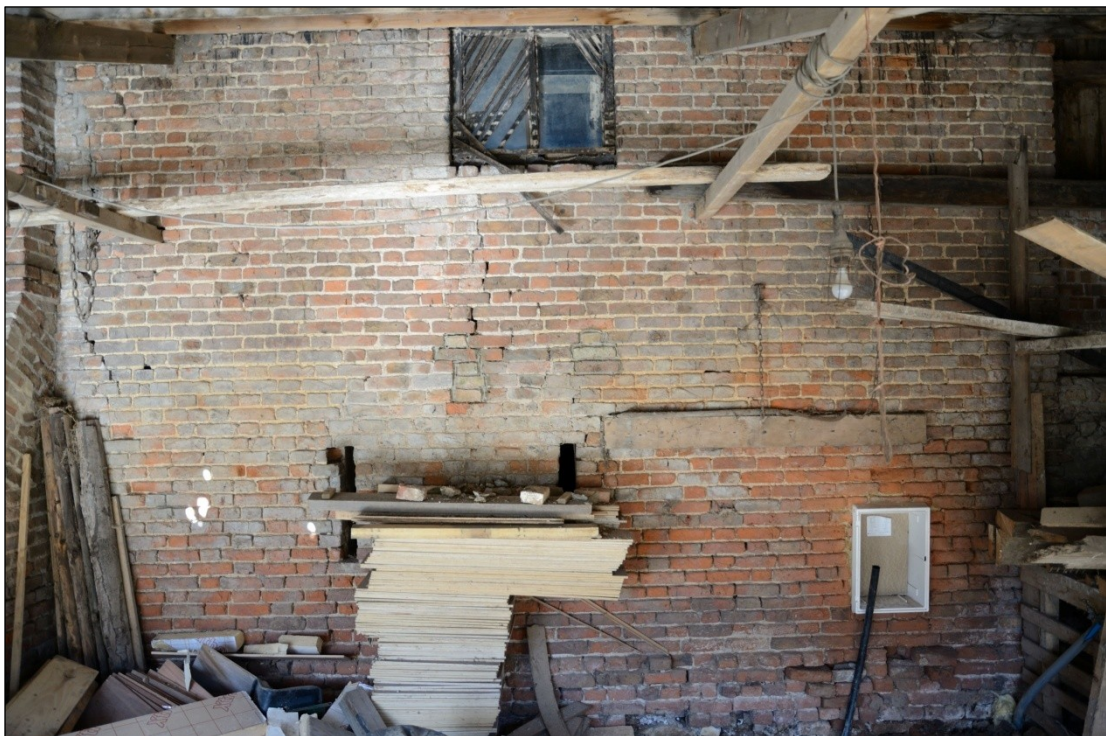
Plate 54: South facing elevation, Barn 2 east of door, looking north
