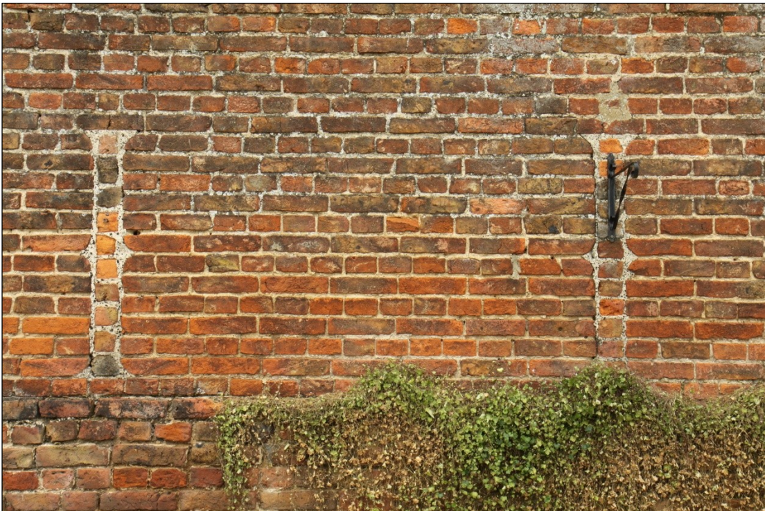
Plate 6: Ventilation slots in the south facing elevation of Barn 1, looking north
