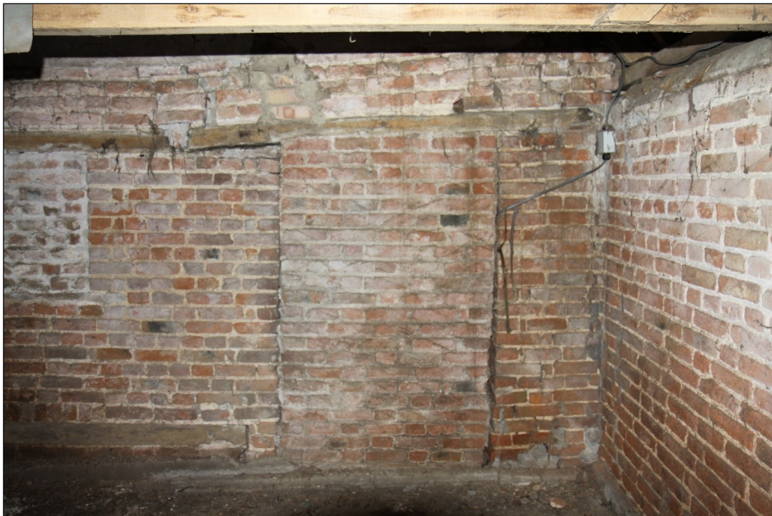
Plate 82: Bricked up door in the east wall of Barn 2, looking east
