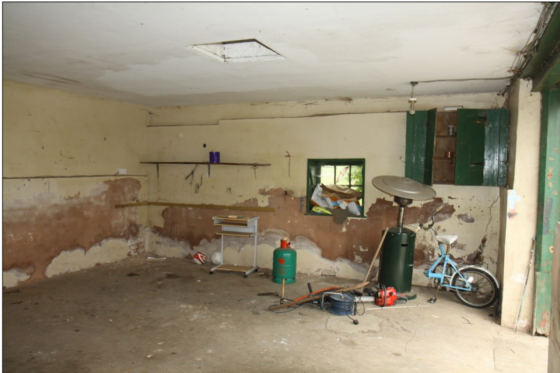
Plate 32: Unit at the eastern end of Barn 1, looking northeast
