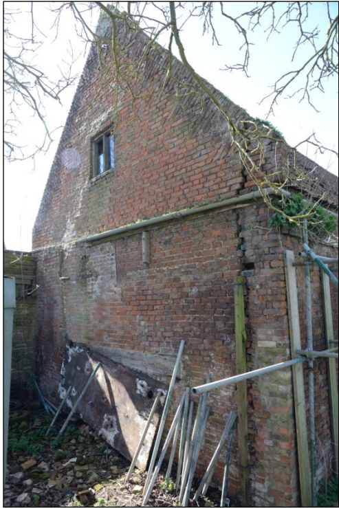
Plate 55: East end of Barn 2, looking southwest
