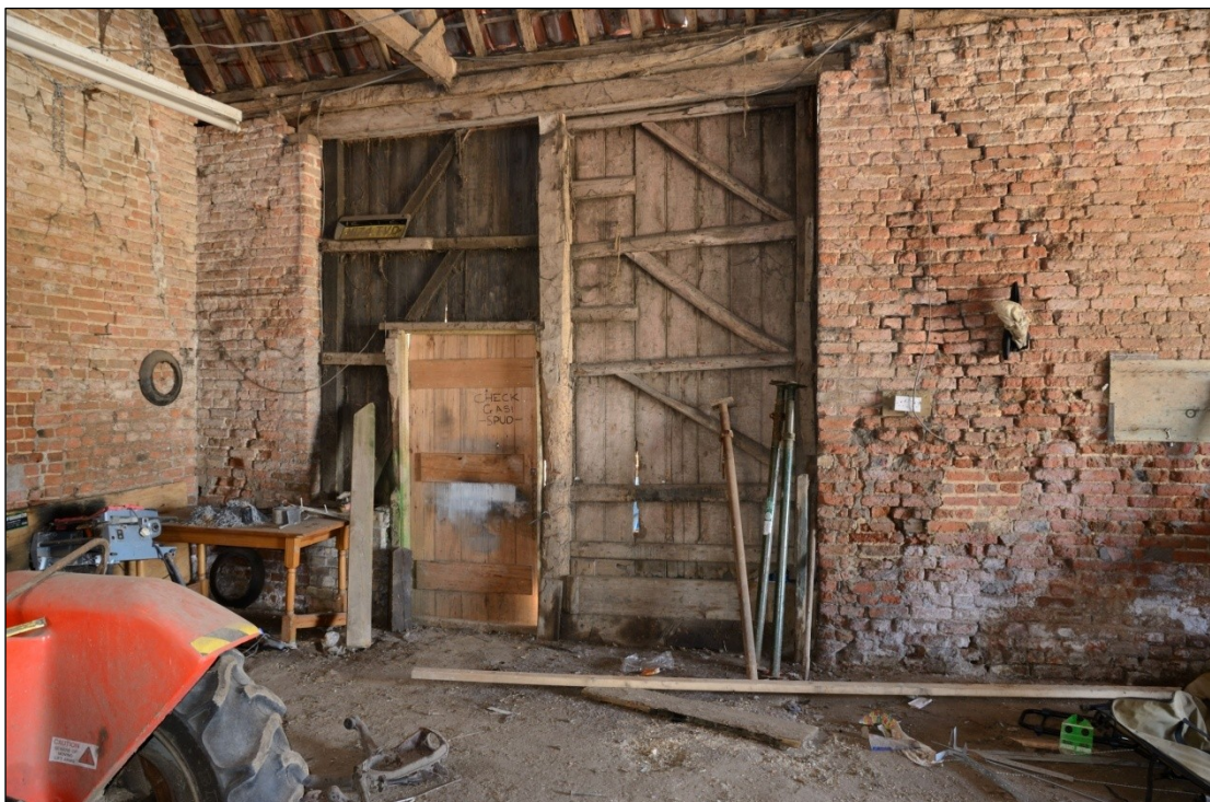
Plate 70: Interior of the door in Barn 2, looking southeast
