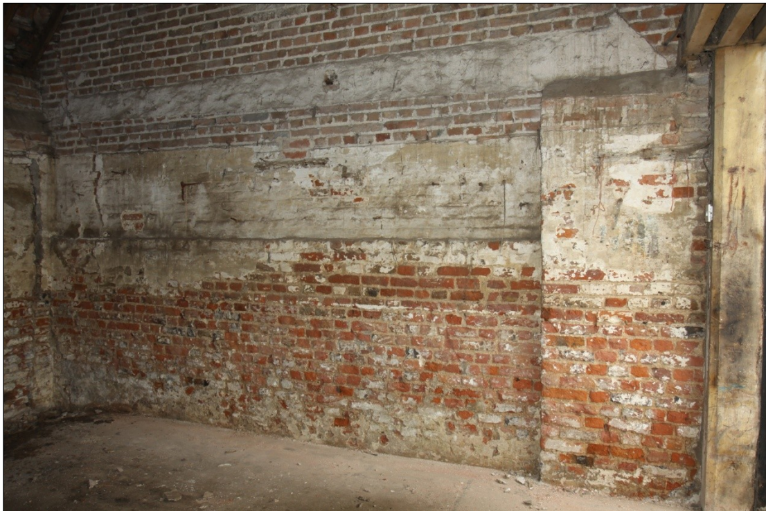
Plate 47: Interior of the extension west of Barn 1, looking northeast
