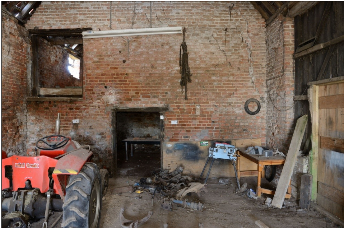
Plate 73: Internal wall in Barn 2, looking east
