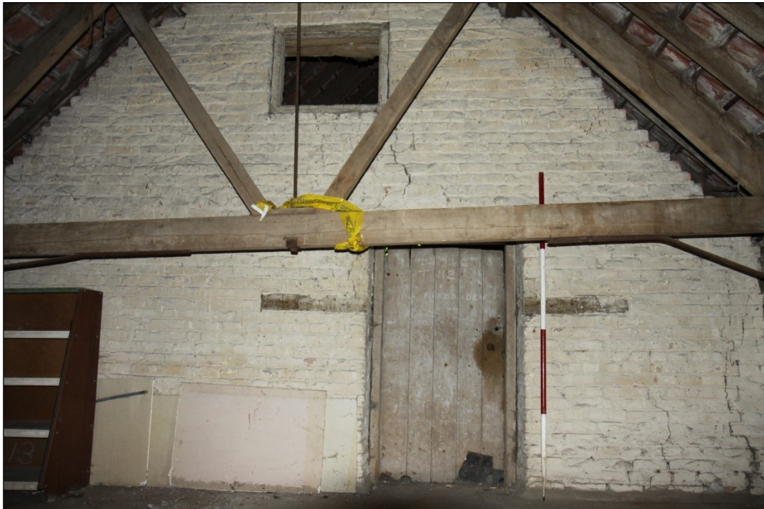
Plate 36: Interior of the hayloft in Barn 1, looking east (2m scale)
