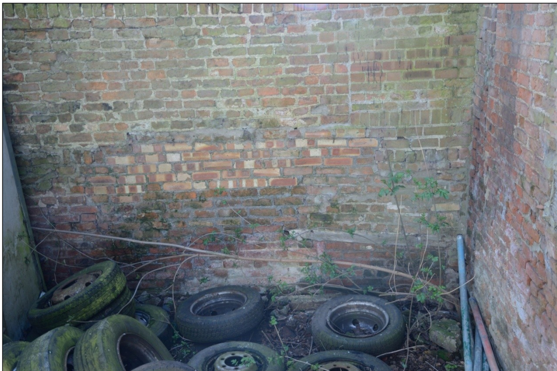
Plate 60: Yard wall at east end of Barn 2, looking south
