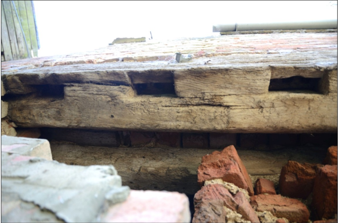
Plate 59: Underside of reused timber lintel, east facing elevation of Barn 2, looking up
