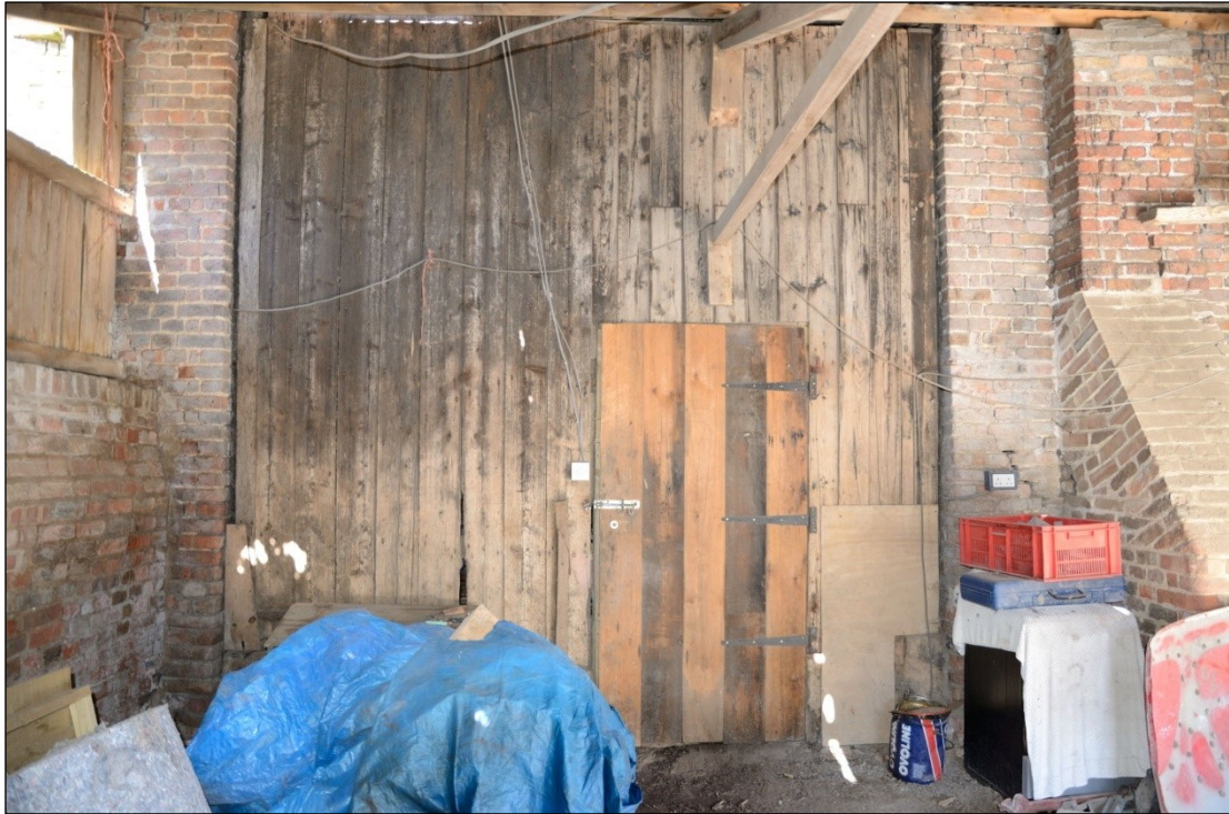
Plate 53: Door in the south facing elevation of Barn 2, looking north
