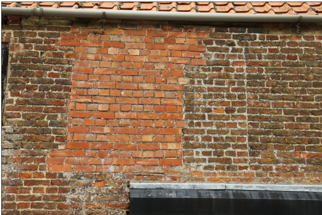
Plate 8: Position of probable pitching door in the south facing elevation of Barn 1
