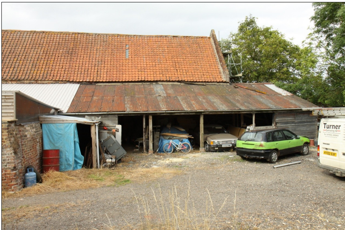
Plate 50: South facing elevation of Barn 2, looking north
