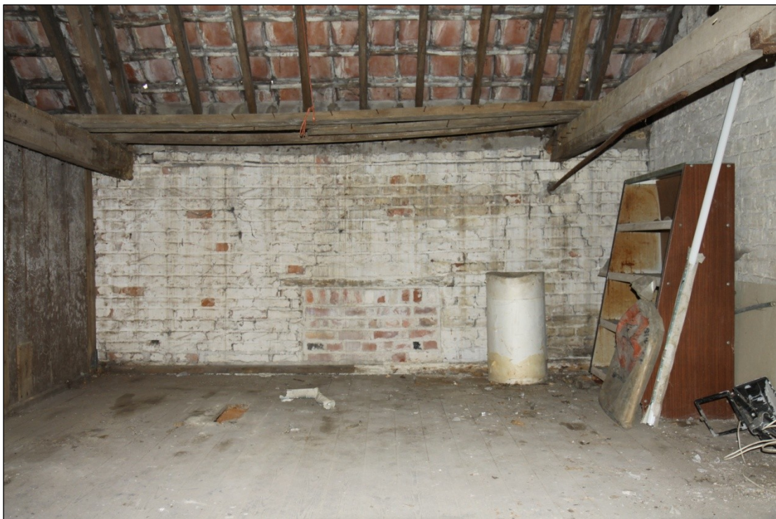
Plate 37: Interior of the hayloft in Barn 1, looking north
