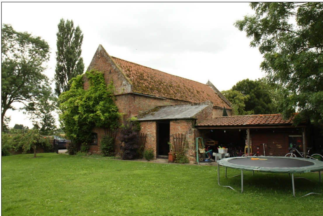
Plate 2: General view of Barn 1 and adjacent outhouse, looking southwest
