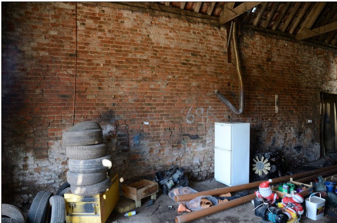
Plate 72: Interior view of ventilation slots in the north wall of Barn 2, looking northeast
