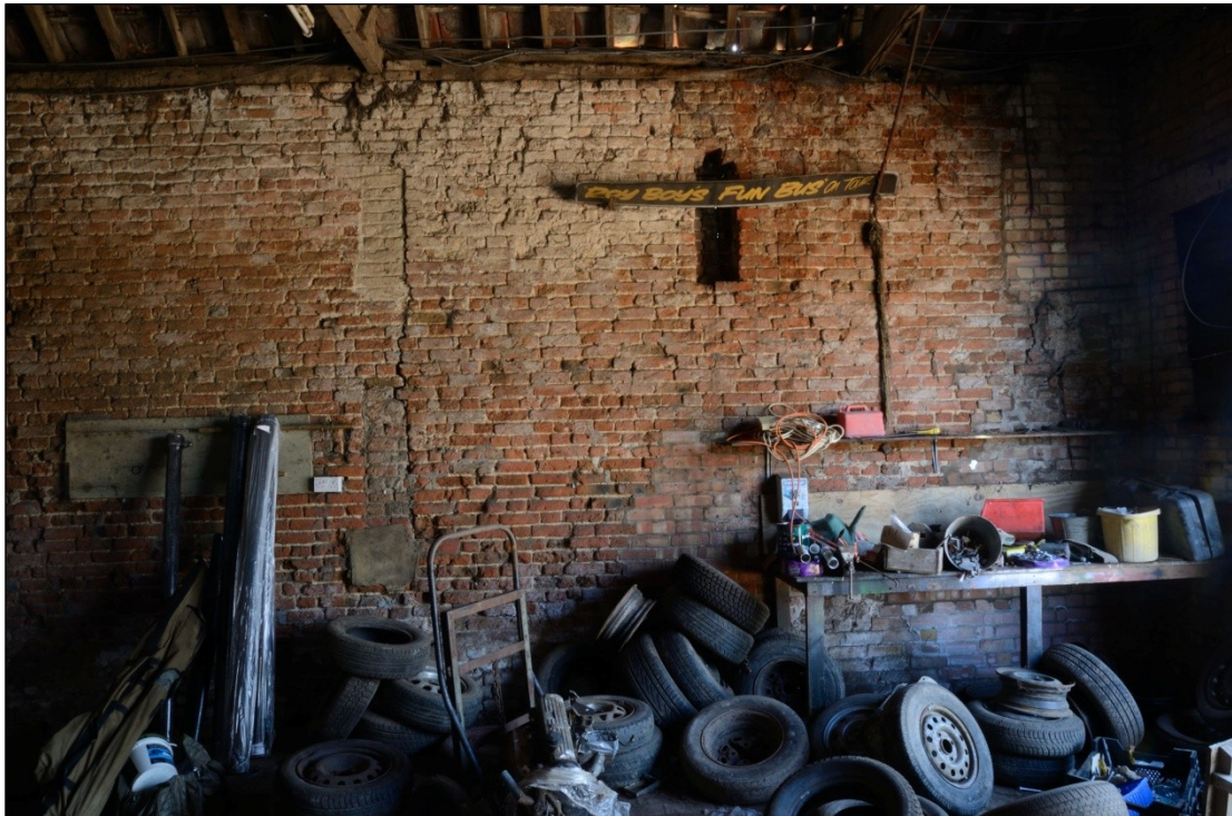
Plate 69: Interior of Barn 2, ventilation slots in the south wall, looking south
