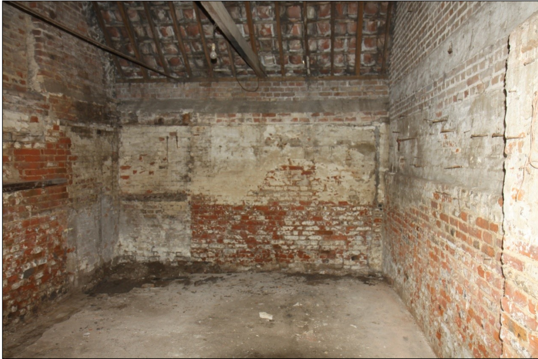
Plate 46: Interior of the extension west of Barn 1, looking north
