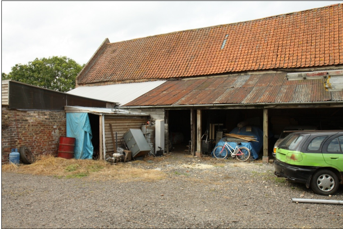
Plate 49: South facing elevation of Barn 2, looking northwest
