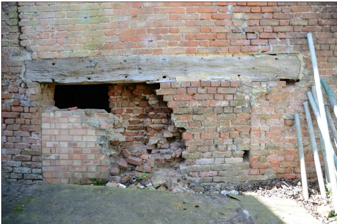
Plate 56: Ground floor opening, east end of Barn 2, looking west
