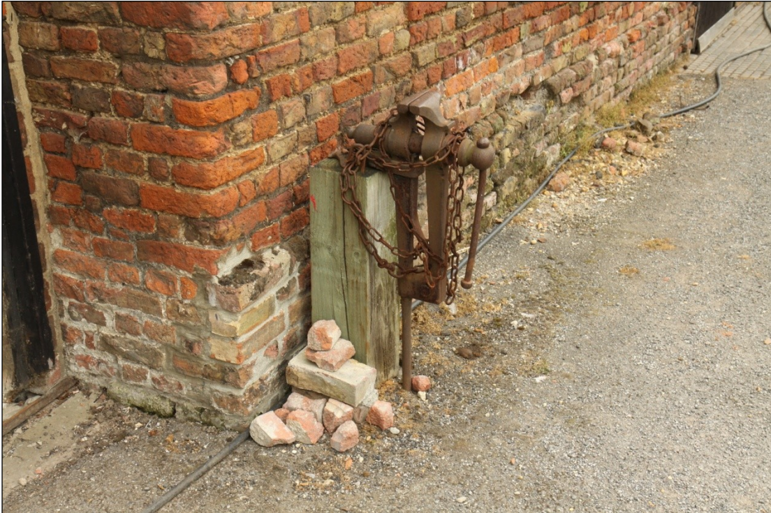
Plate 5: Vice positioned near the southwest corner of Barn 1, looking northeast
