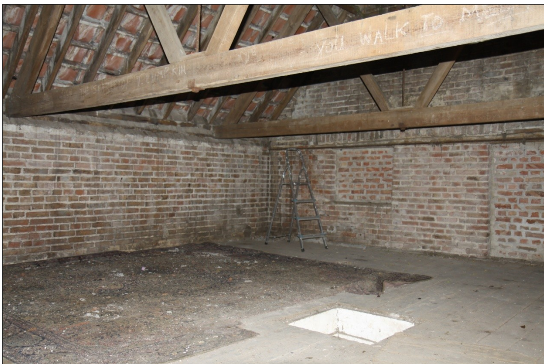
Plate 41: Interior of the probable granary in Building 1, looking northeast
