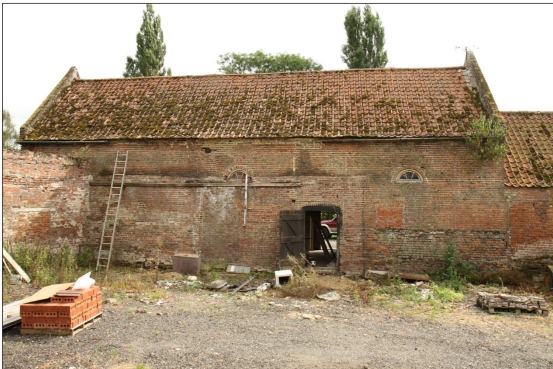
Plate 16: North facing elevation of Barn 1, looking south
