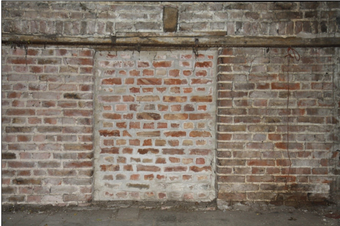
Plate 42: Bricked up doorway in the east wall of the probable granary in Barn 1, looking east
