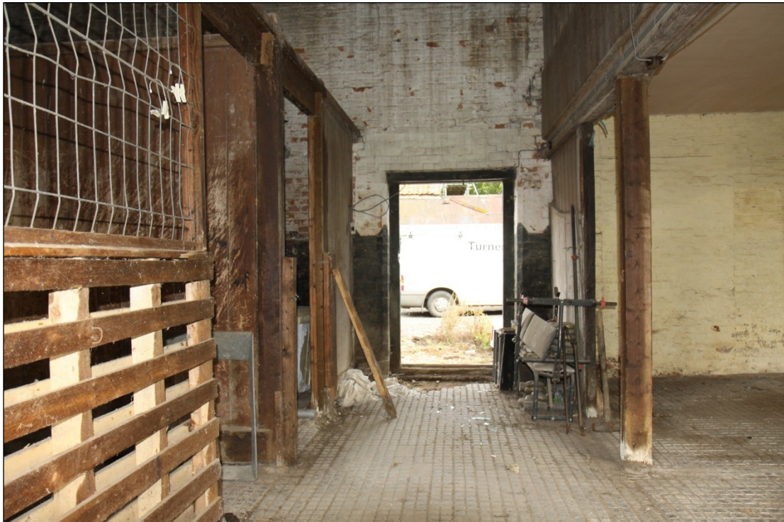
Plate 26: Passage through the stables in Barn 1, looking north
