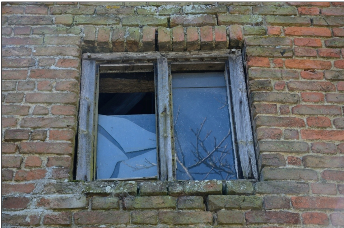
Plate 58: East facing elevation of Barn 2, opening in gable, looking west
