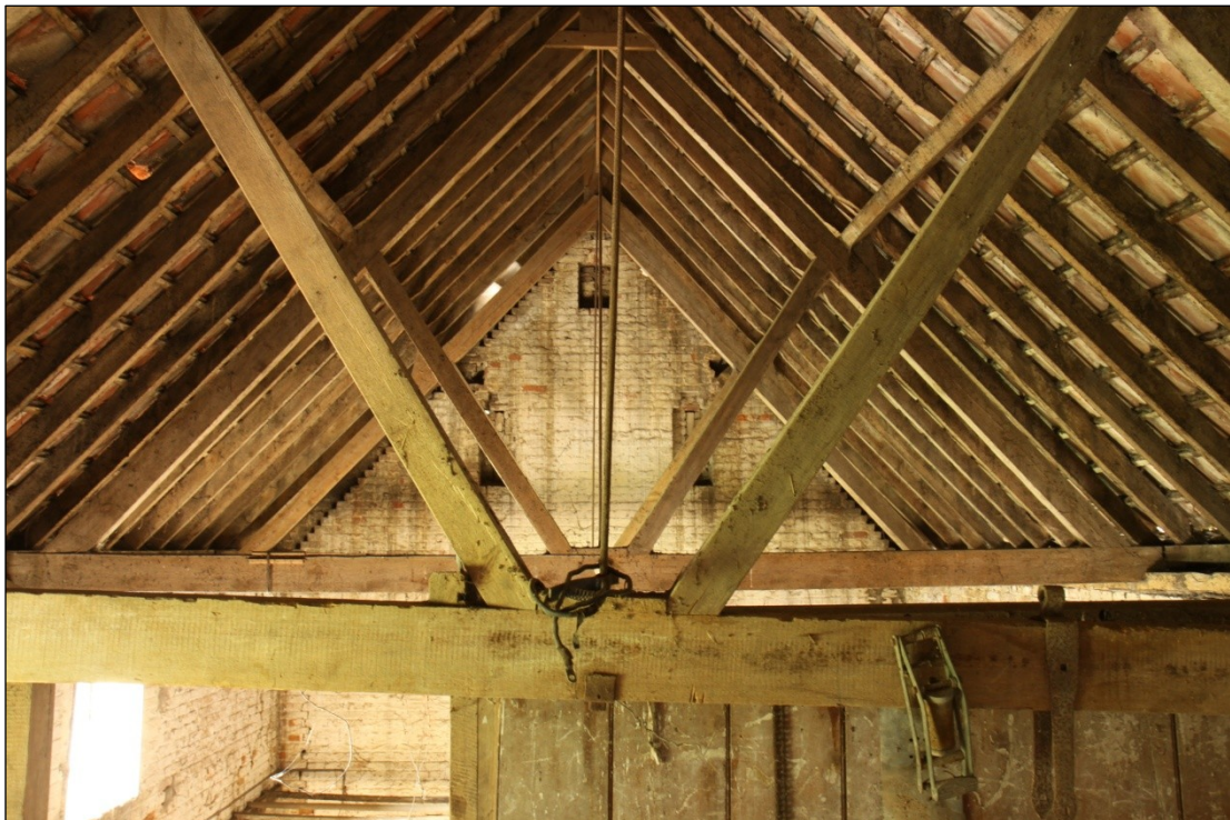
Plate 45: Roof structure in the western part of Barn 1, looking west
