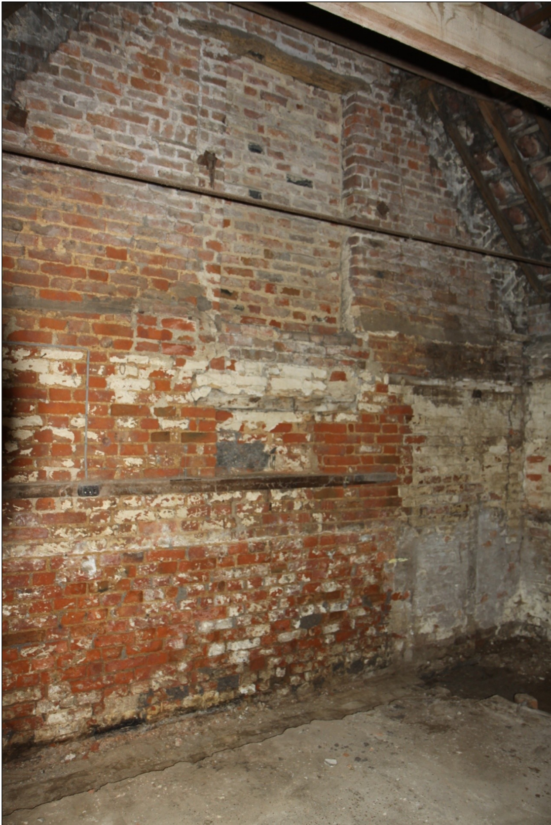
Plate 48: Interior of the extension to Barn 1, looking northwest
