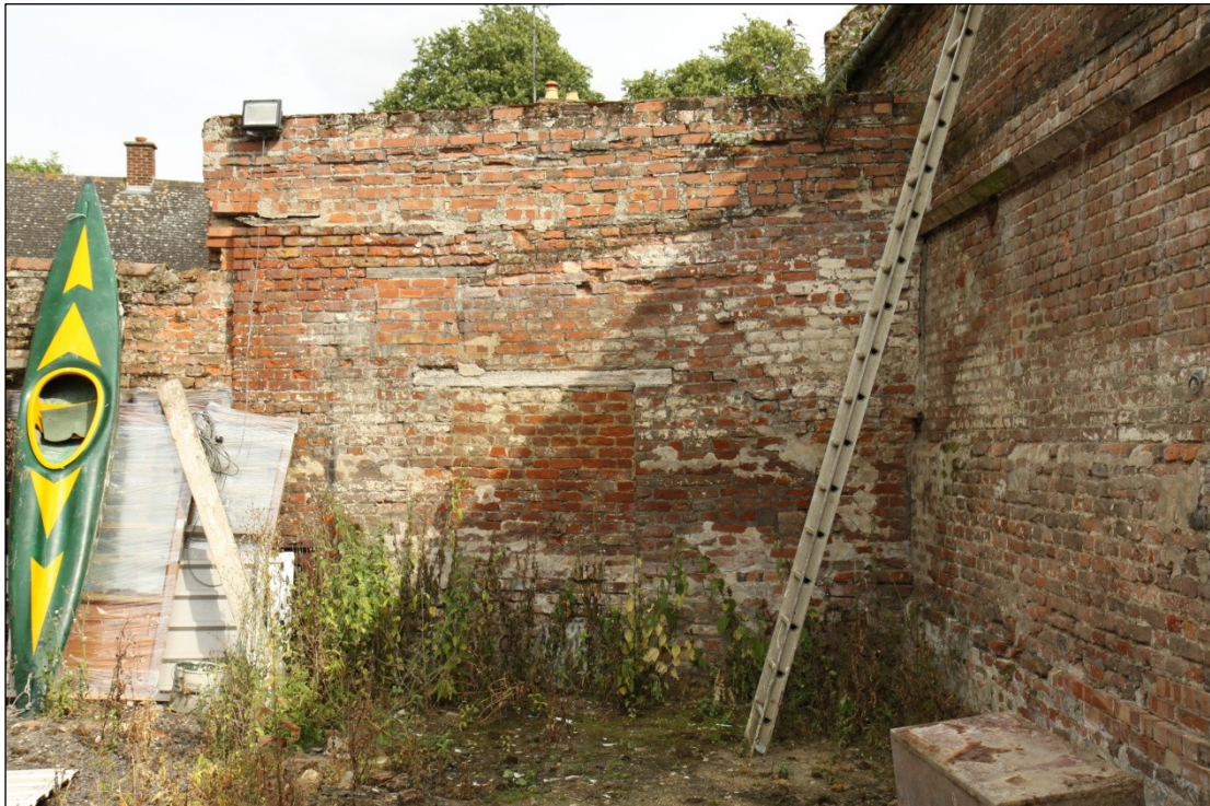
Plate 15: Rear wall of the outhouse north of Barn 1, looking east
