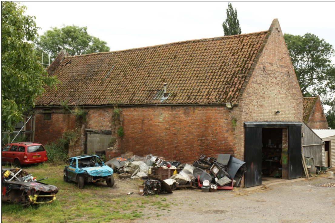
Plate 61: General view of Barn 2, looking southwest
