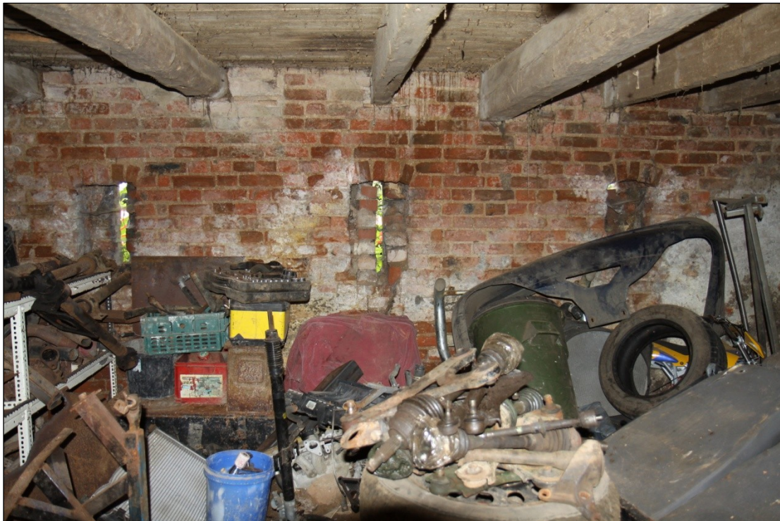
Plate 76: Interior view of ventilation slots in the north wall (east end) of Barn 2, looking north
