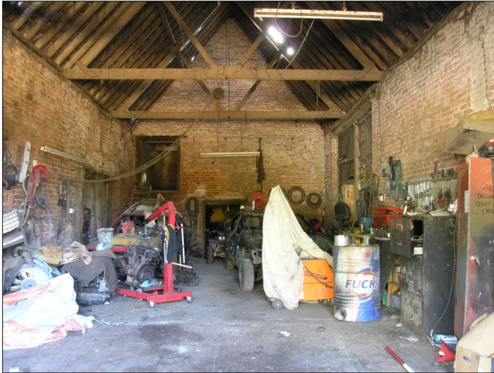
Plate 67: Interior of Barn 2, looking east
