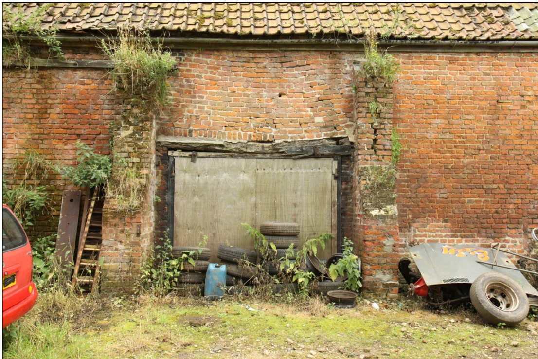
Plate 64: Doorway in the north facing elevation of Barn 2, looking south
