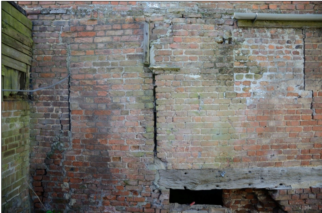
Plate 57: East facing elevation of Barn 2, first floor openings, looking west
