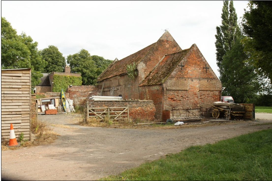
Plate 3: General view of Barn 1, looking southeast
