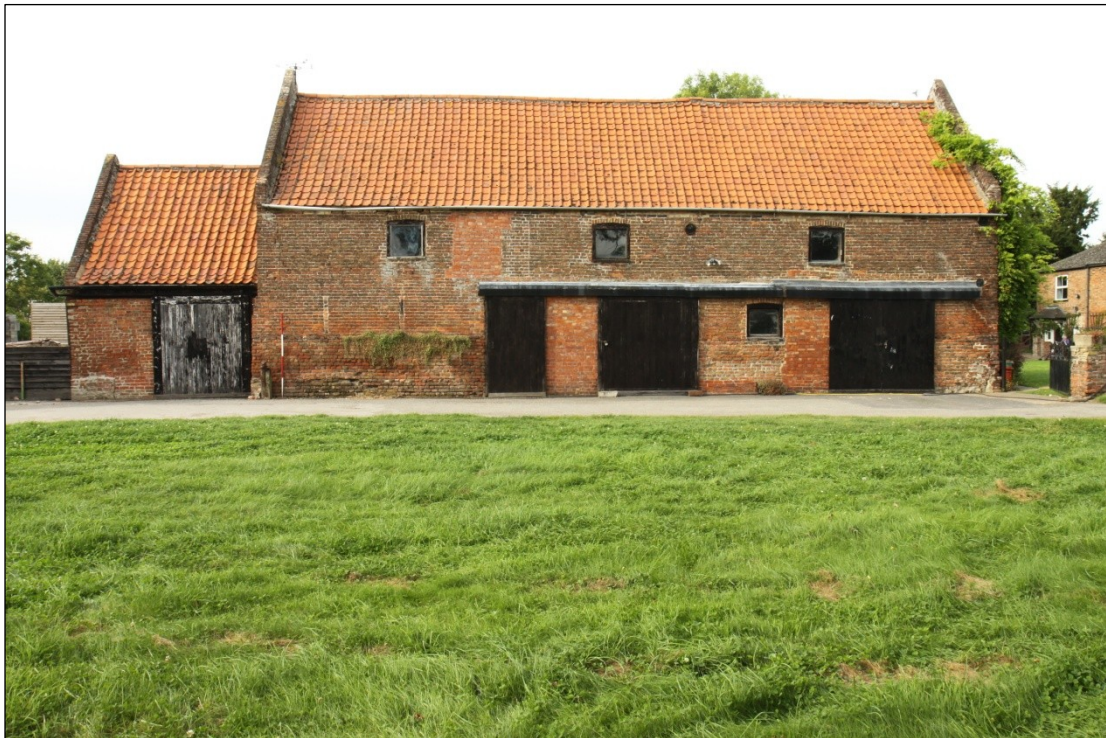
Plate 4: South facing elevation of Barn 1 with 2m scale, looking north
