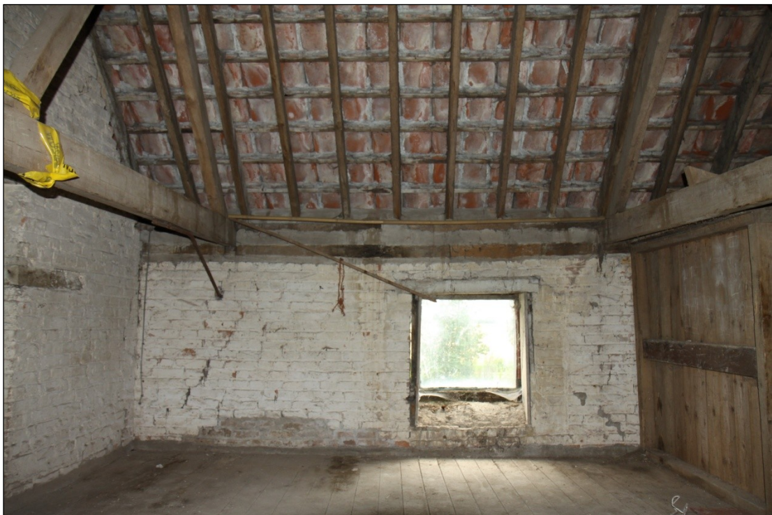
Plate 35: Interior of the hayloft in Barn 1, looking south
