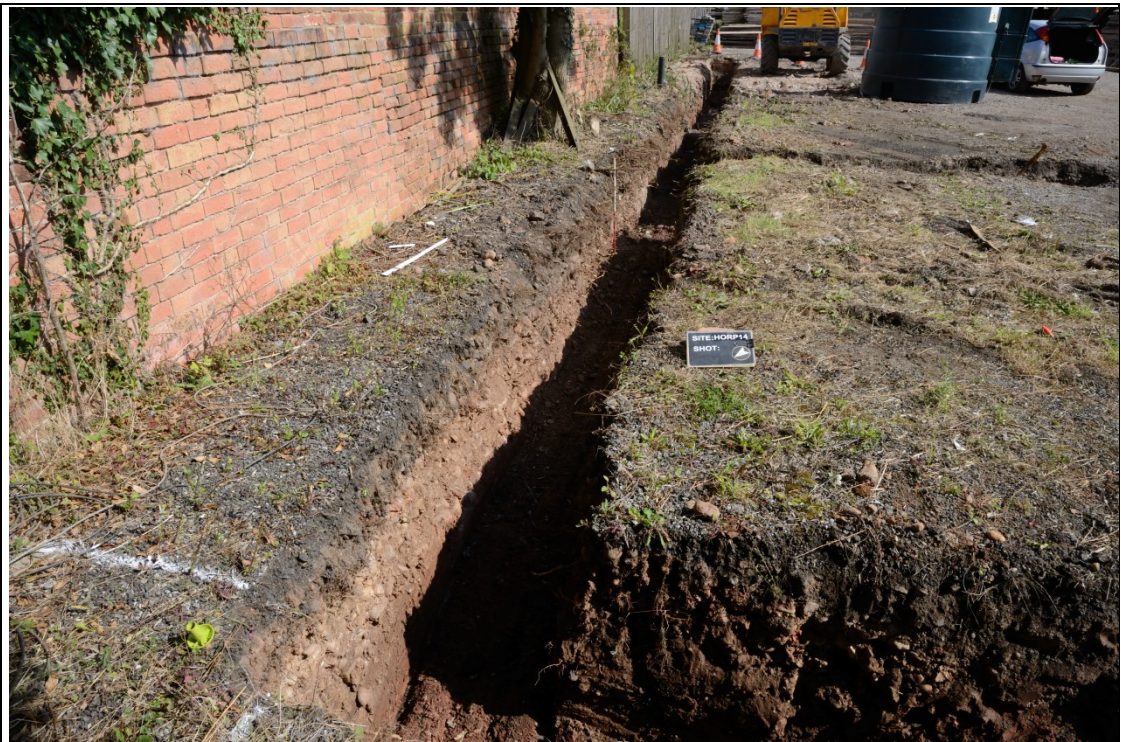
Plate 4: Northeast side of the new building, looking east; 1m scale
