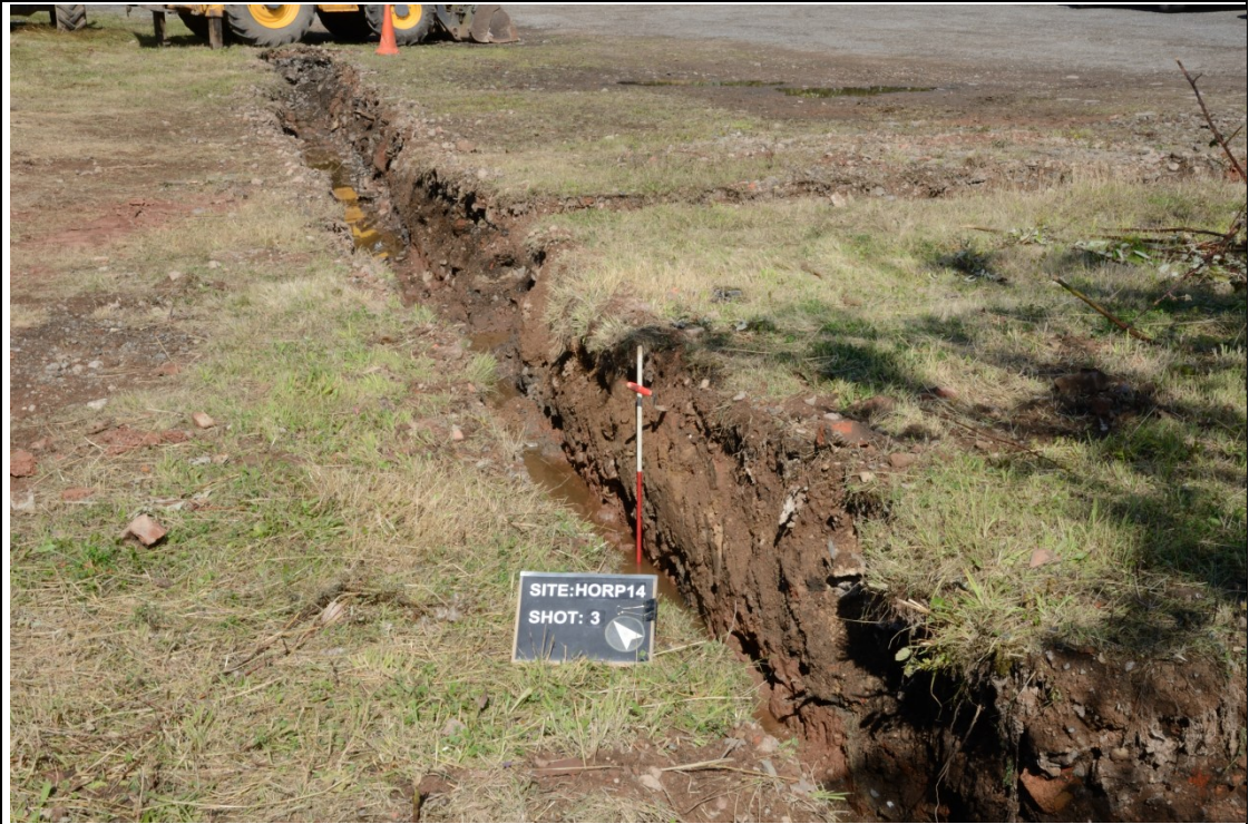
Plate 3: Southeast side of the main block, looking northeast; 1m scale
