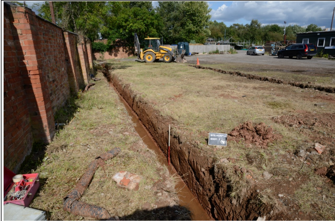
Plate 1: Foundation trench including Section 2, looking northeast; 1m scale
