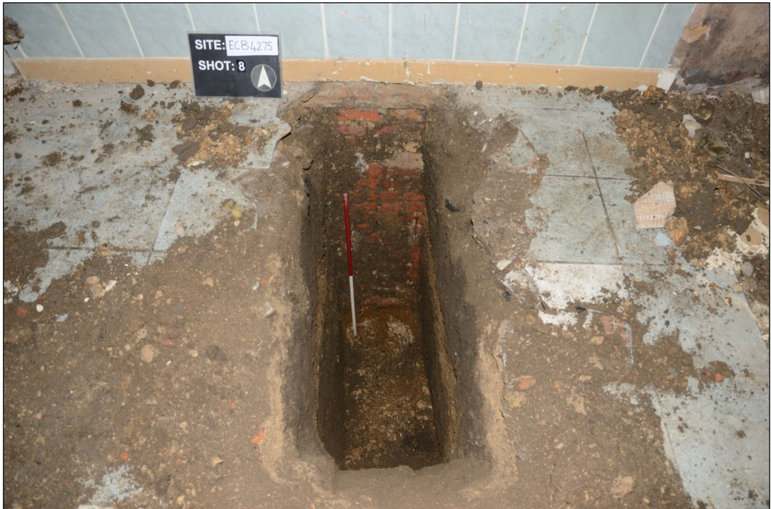
Plate 12: Pit 2, wall foundations, looking north; 1m scale
