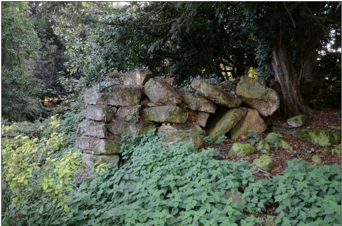
Plate 10: Stone structure west of Trench 2; looking west
