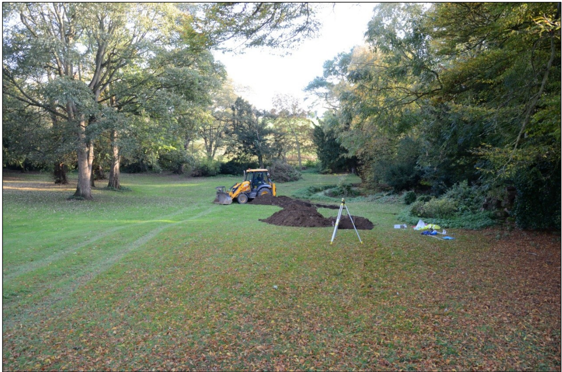
Plate 2: General view of Trenches 2 and 3, looking south
