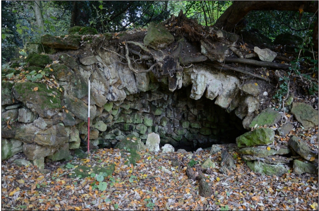
Plate 9: Stone 'grotto', looking c. northwest; 1m scale
