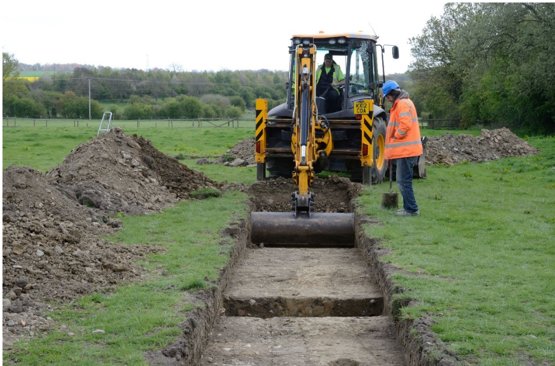
Plate 2: Machining of Trench 4. Looking southeast
