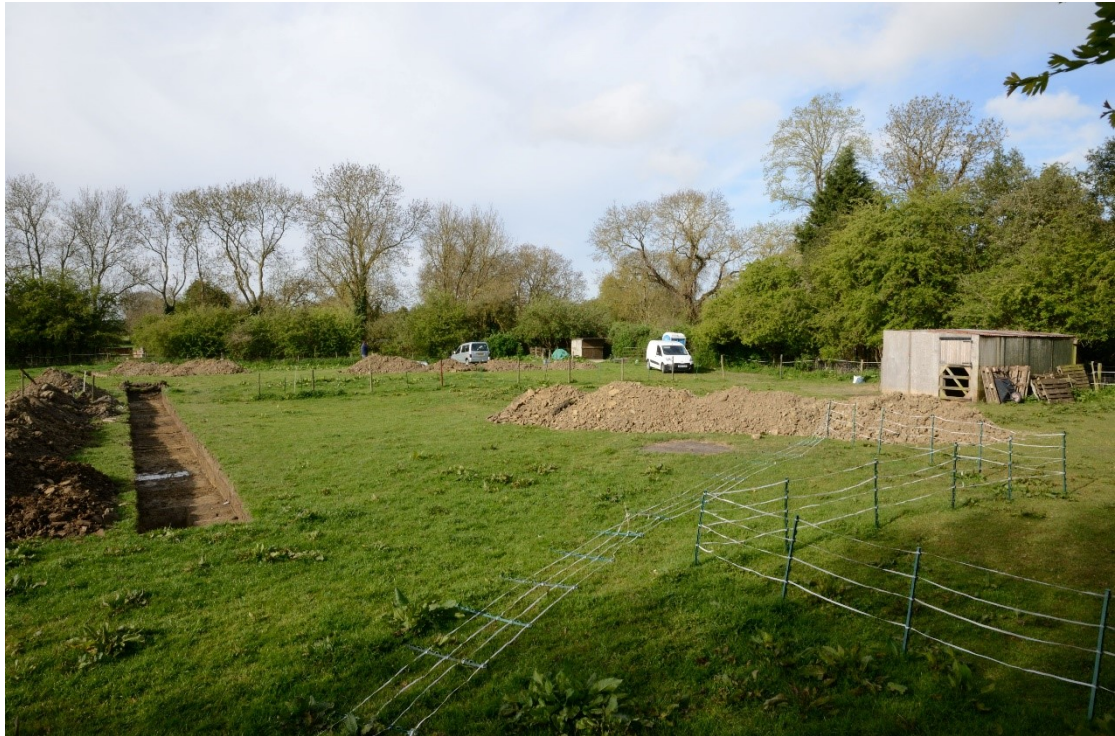
Plate 1: General view of the site during trial trenching, looking southwest
