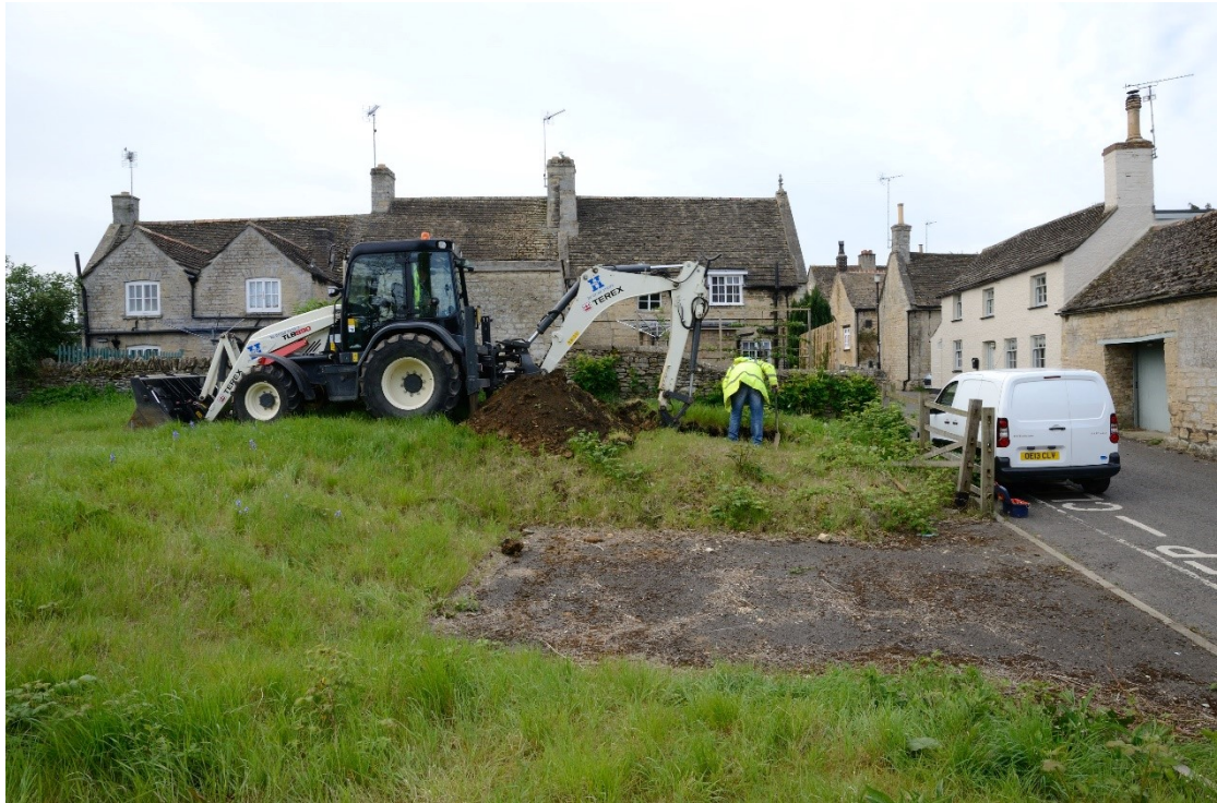
Plate 1: Excavation of Trench 1 in progress. From north.
