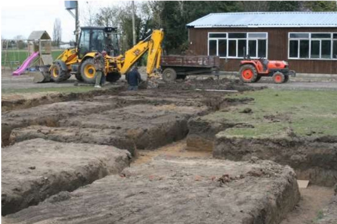
Plate 1: General view of work in progress from south
