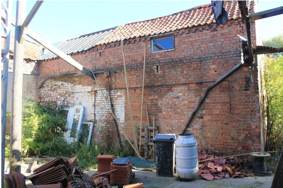
Plate 29 West external elevation of building E and barn C, looking east.
