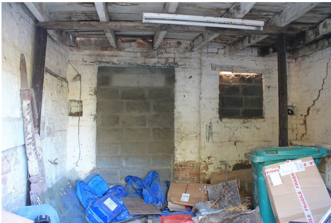
Plate 4 Ground floor interior of stable A, showing blocked door and window, tack hook and recesses in south wall, blocked door and timber of east wall visible at left, looking south.
