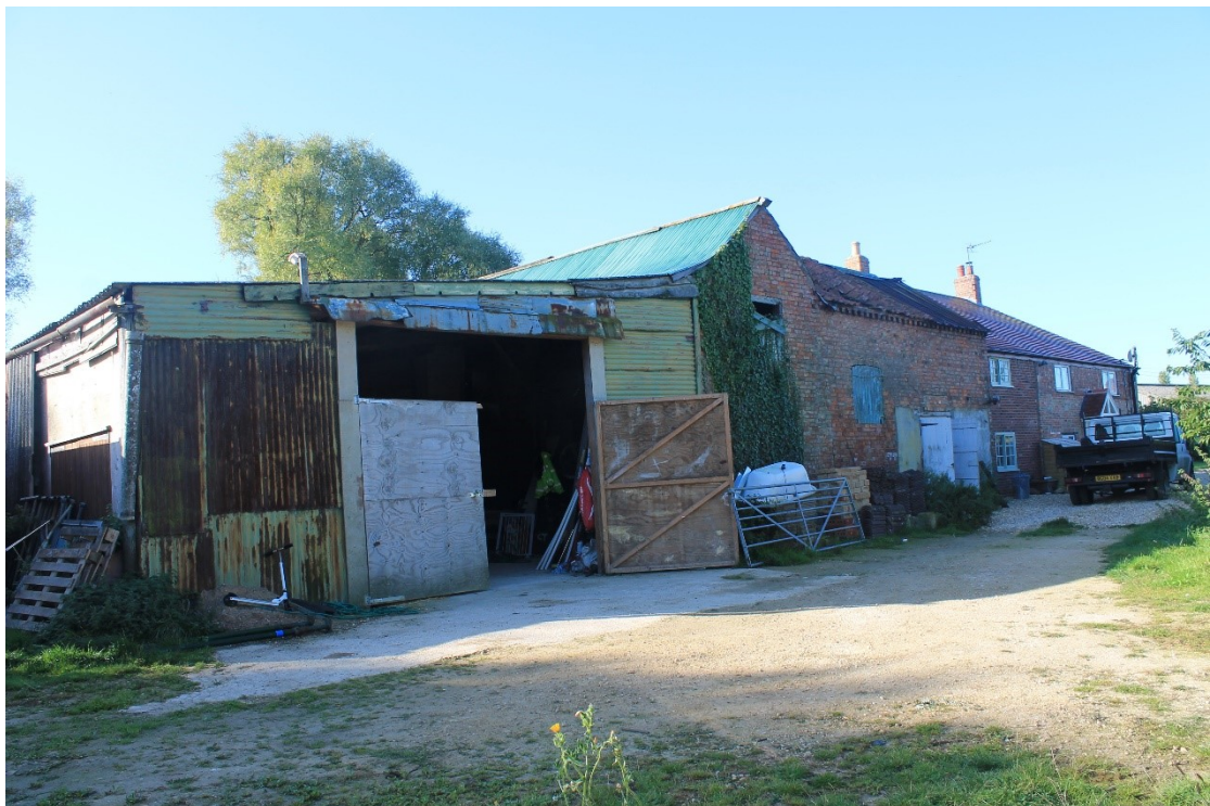
Plate 30 North elevation of shelter shed D, attached to barn C, and general view of north elevation of farmhouse and outbuildings, looking southwest.
