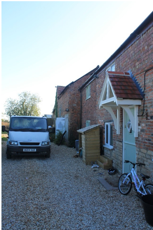
Plate 1 General view showing north elevation of farmhouse and recorded outbuildings in background, looking east.
