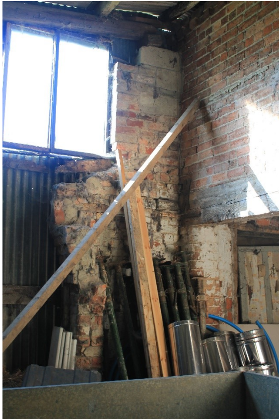
Plate 21 Detail of fragmentary masonry of structure G, apparently forming passageway associated with conversion of cart shed E to stables, looking southwest.
