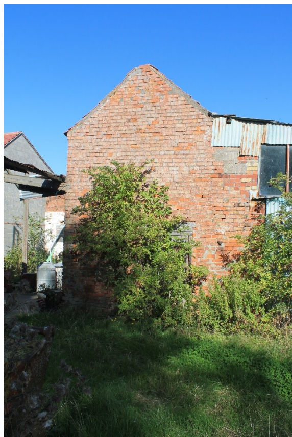
Plate 28 South gable of building E and adjoining structure G, looking north.
