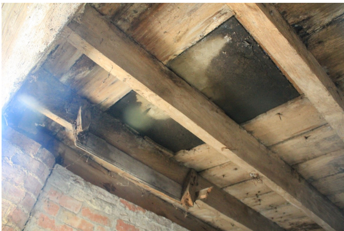
Plate 24 Interior detail of north bay of cart shed E, possible trapdoor in ceiling and possibly associated woodwork attached to joist, looking south.
