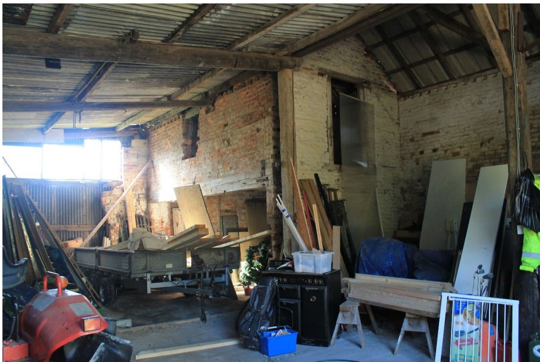
Plate 19 Cart shed and possible granary E, as viewed from inside shelter shed D, looking southwest.
