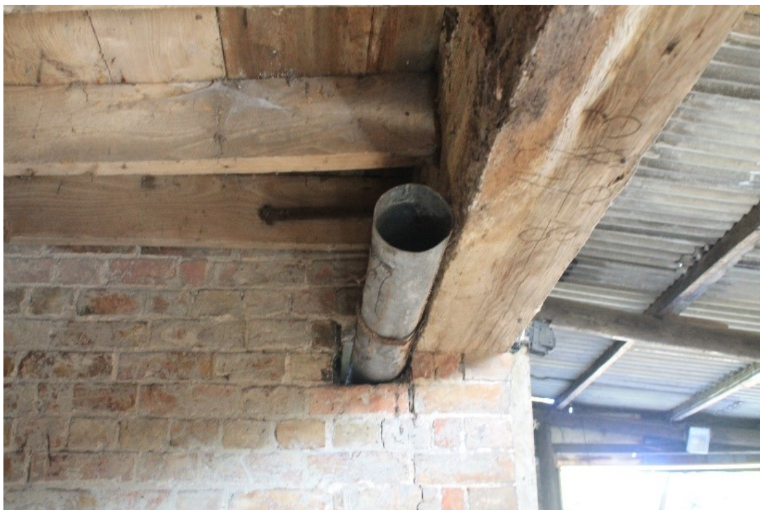
Plate 23 Interior detail of north bay of cart shed E, showing metal pipe exiting north wall of bay, possibly associated with former stove within this room during use as a stable, looking north.
