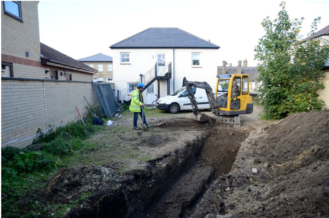
Plate 1: General view of the site during backfilling of Trench 1, looking north
