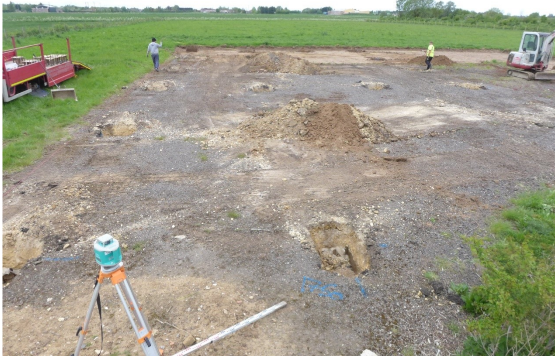
Plate 2: General view of the excavated stanchion pits looking west
