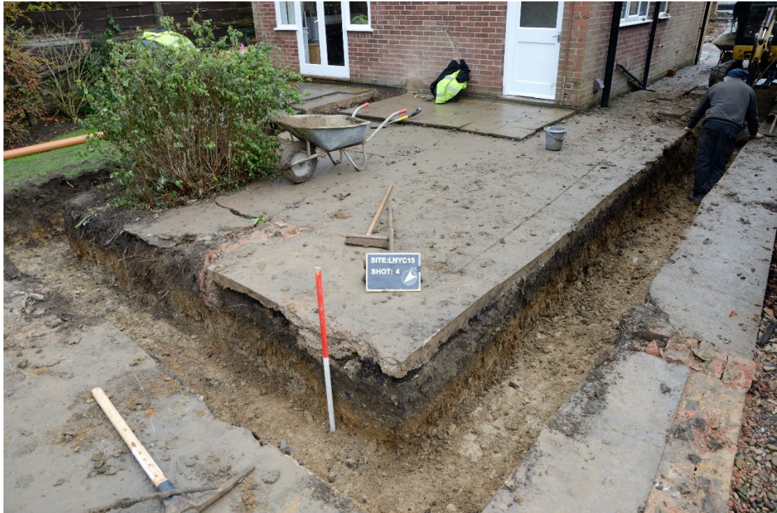
Plate 1: General view of footings from northeast, Scale 1m
