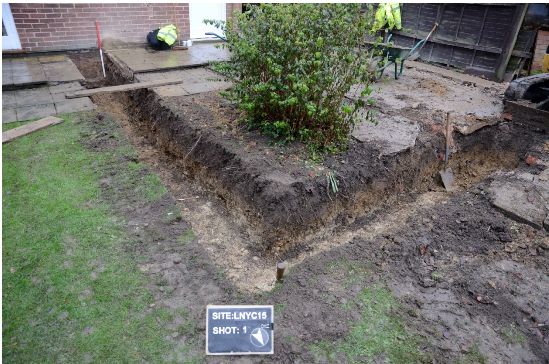
Plate 2: General view of footings from northwest, Scale 1m
