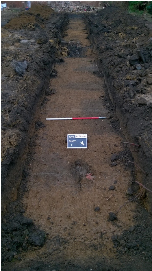
Plate 2: Trench 1, looking southwest
