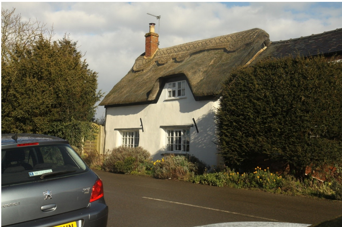
Plate 16 Maytree Cottage from west side of Mill Lane
